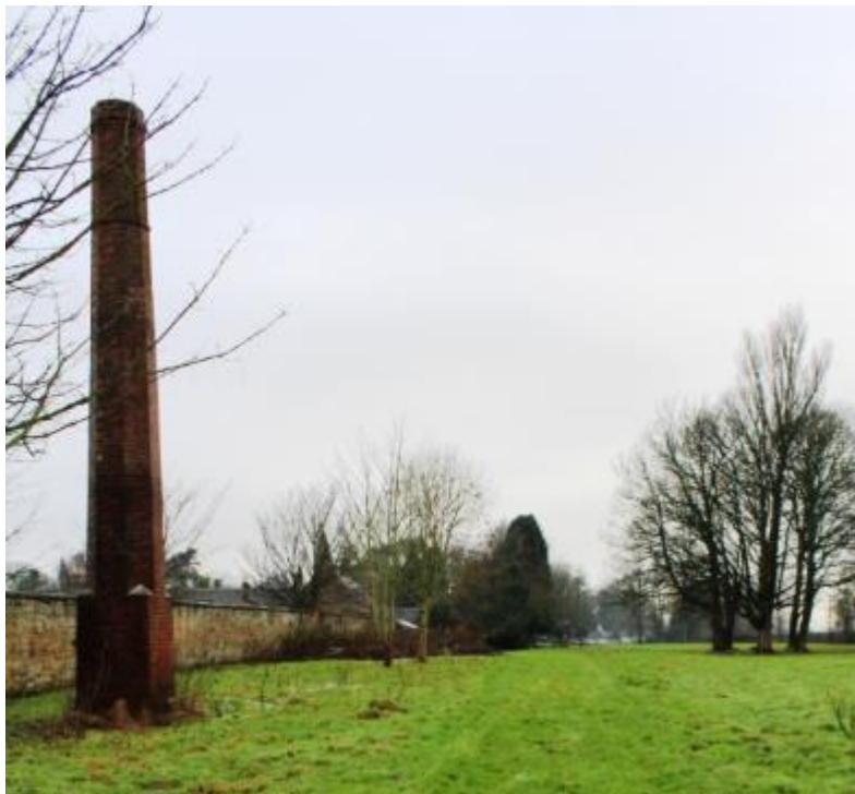
Illus 22: Chimney stack with oven / stove adjacent to walled garden
