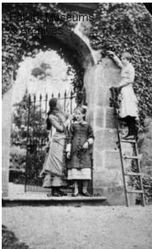
Illustration 16 : Late 19th century photograph of the arched entrance to the Walled Garden
