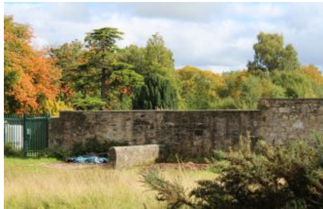
Illustration 29 : Concrete pads and remains of the new stable block adjoining the western wall of the Walled Garden
