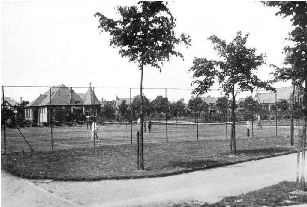
Illus 16: The tennis courts c 1920. Source: SCRAN.
