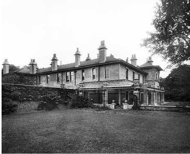
Illus 15: Carronvale House from the north-west. The west wall of the walled garden is on the left. Date of the photograph unknown. Provided by Keith Morrison of the Boys Brigade.
