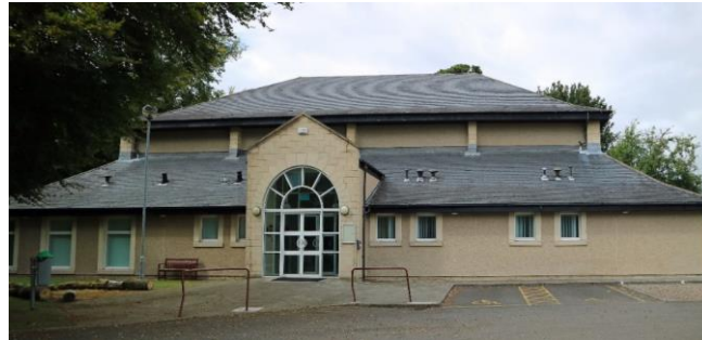
Illus 18: The new recreation centre on the site of the former stables and domestic offices
