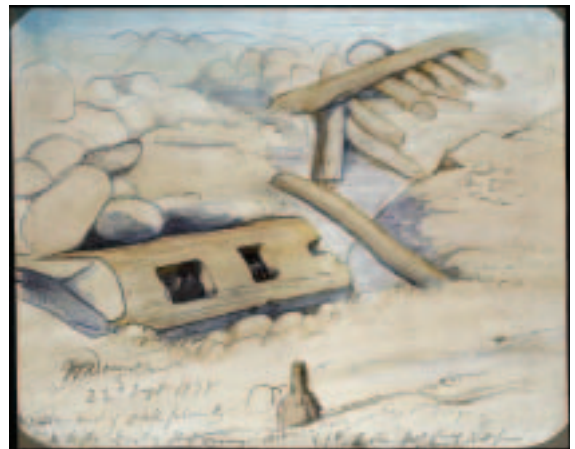
Fig. 30 The excavation of the ladder, 1898. (SC709690)
