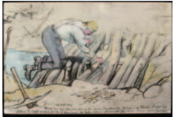
Fig. 29 Ned uncovering the path to the boat dock. (SC709693)
