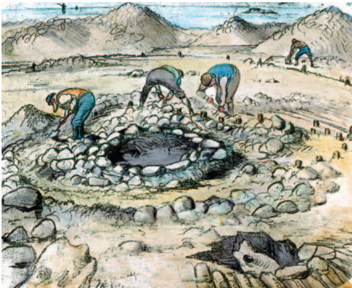
Fig. 28 Excavation of the central pit. (SC691876)
