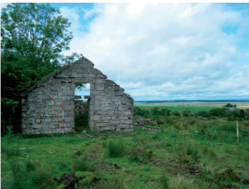
Illus 25 East facing elevation of Building A
