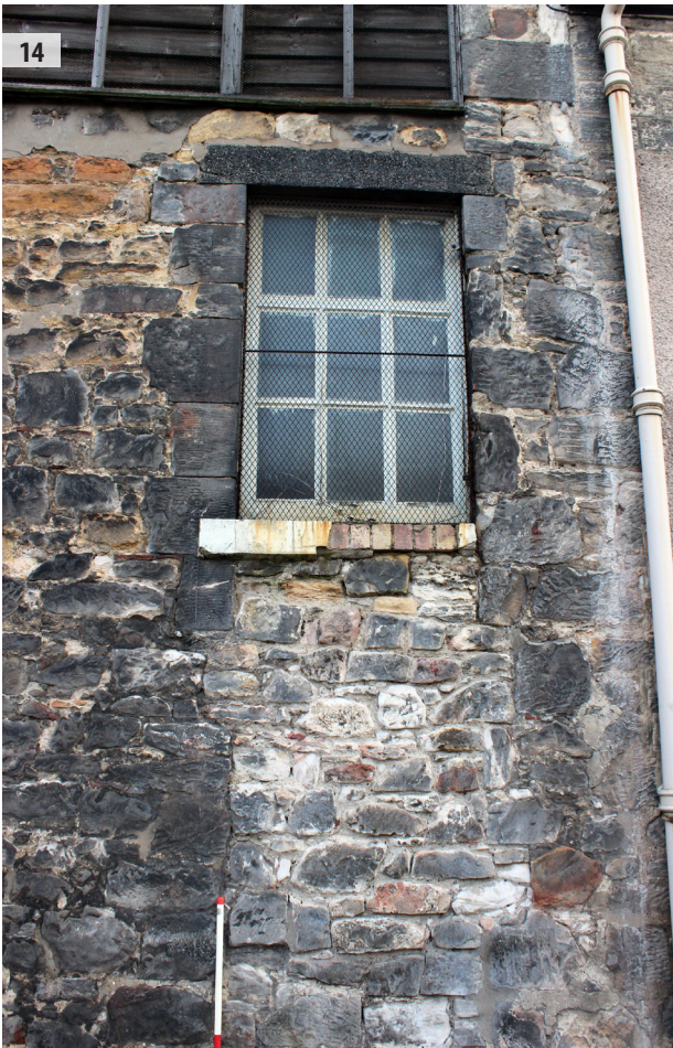
ILLUS 14 Detail of the construction lines on to the west side of Building C
