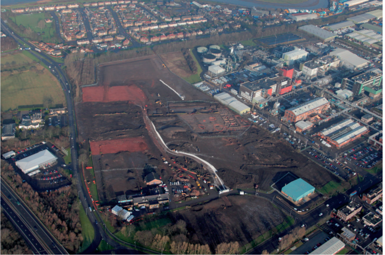
Aerial photo of development area from south Taken by Guthrie Aerial Photography
