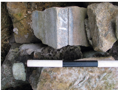
Pile No. B Stone No. 21 Direction W Description Block of buff/light grey ashlar with saw marks - unclear if underside is irregularly shaped/weathered or carved.
