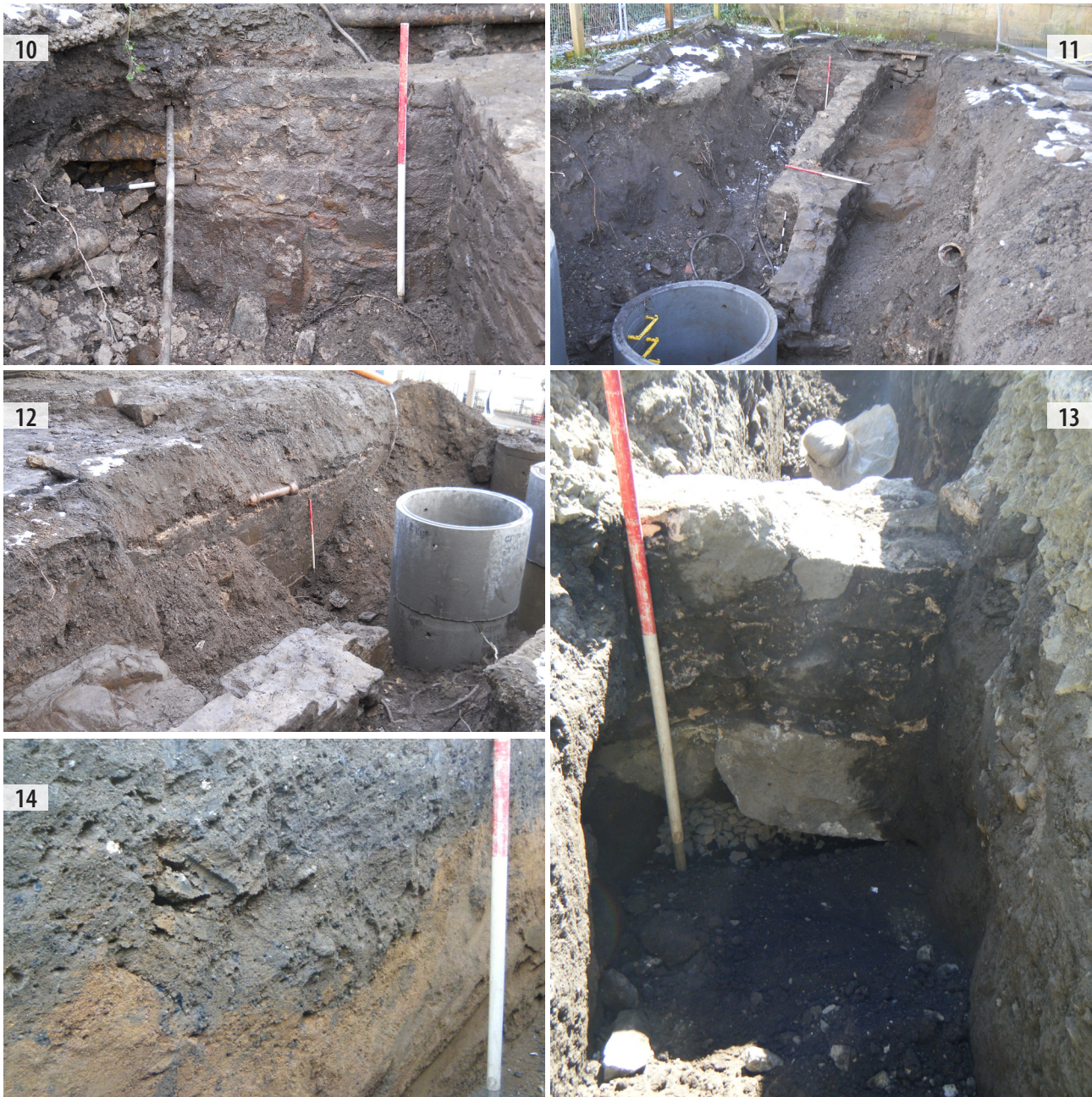
ILLUS 10 Opening [246] in wall [245]. Facing SW ILLUS 11 Wall [247]. Facing S ILLUS 12 Wall [254] at edge of trench. Facing N ILLUS 13 Boundary wall [272]. Facing NW ILLUS 14 Pit [280] exposed in side of service trench. Facing N
