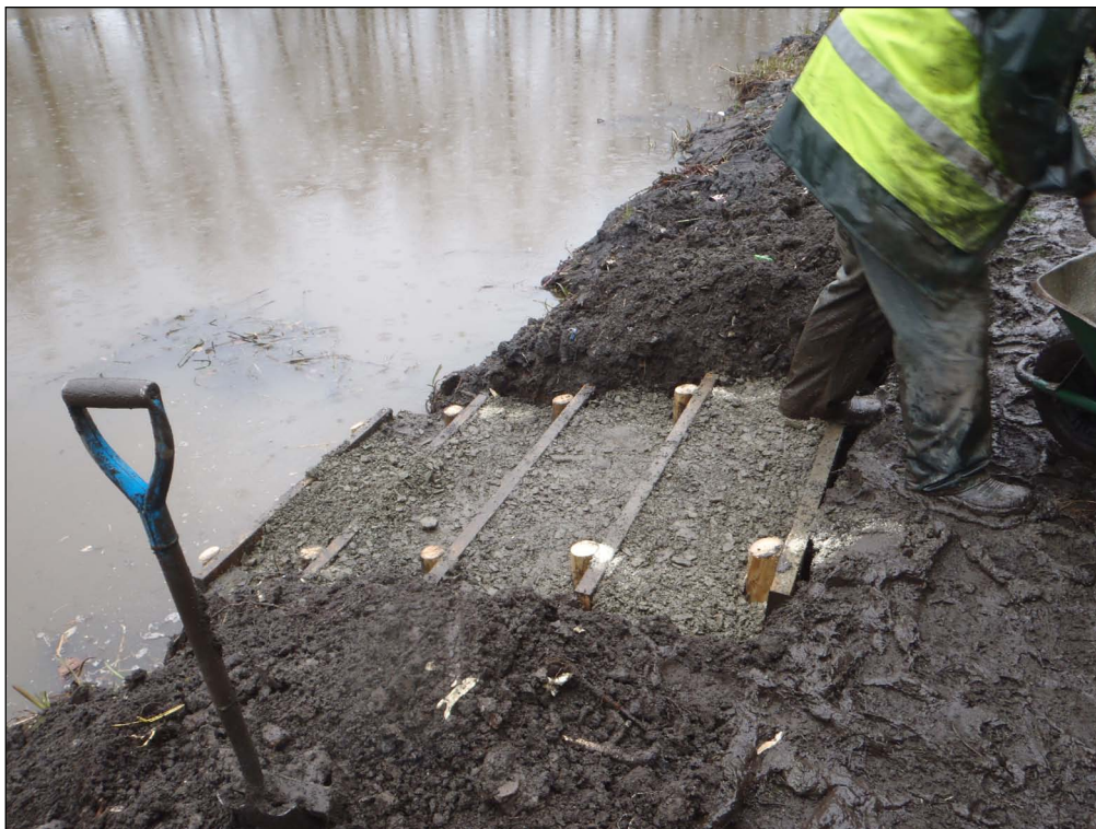
Plate 4 – Completed steps near Bridge 51
