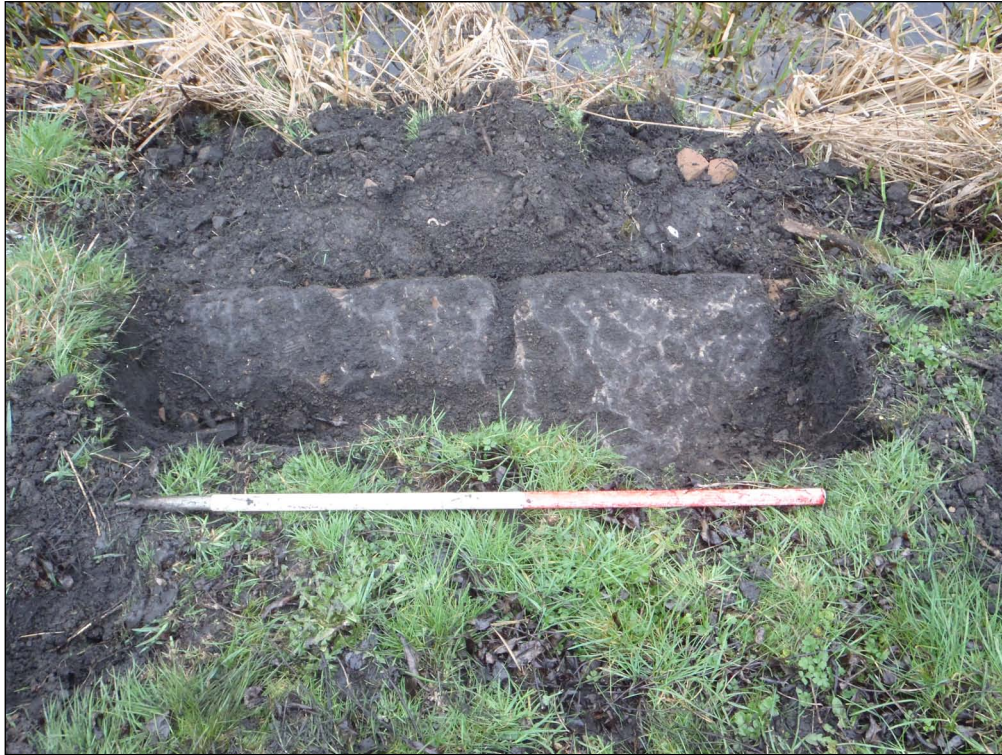
Plate 1 – Exposed canal wall, Broxburn
