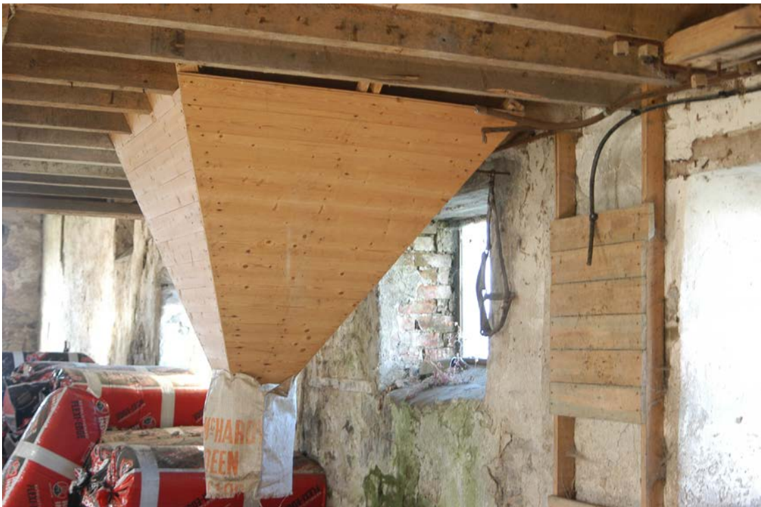
Plate 5 A Sack-filling hopper below the grain store loft
