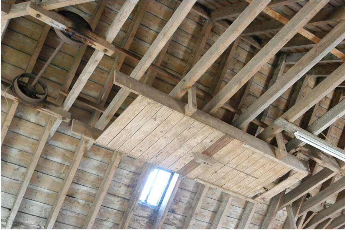
Plate 4 Tie beams and belt-drive wheels in the roof space of the barn
