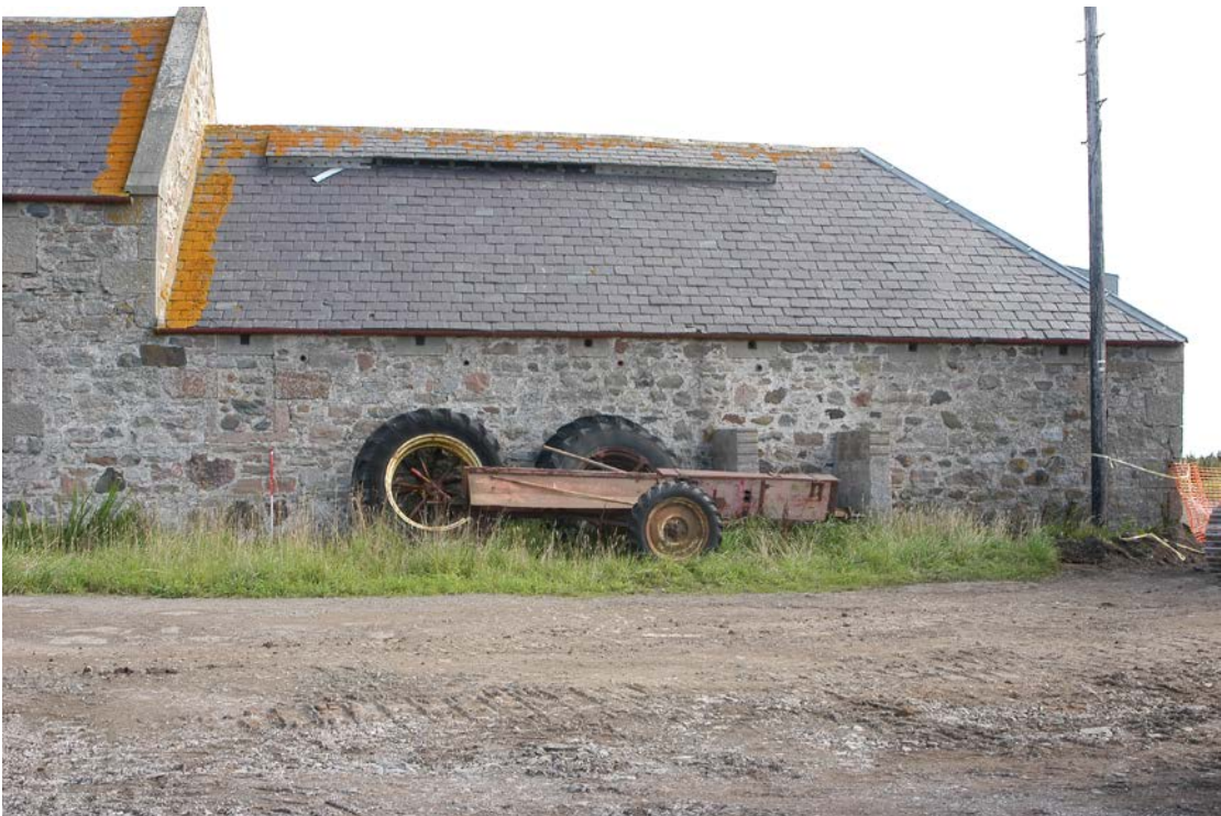
Plate 9 South end of the west range, former cattle shed
