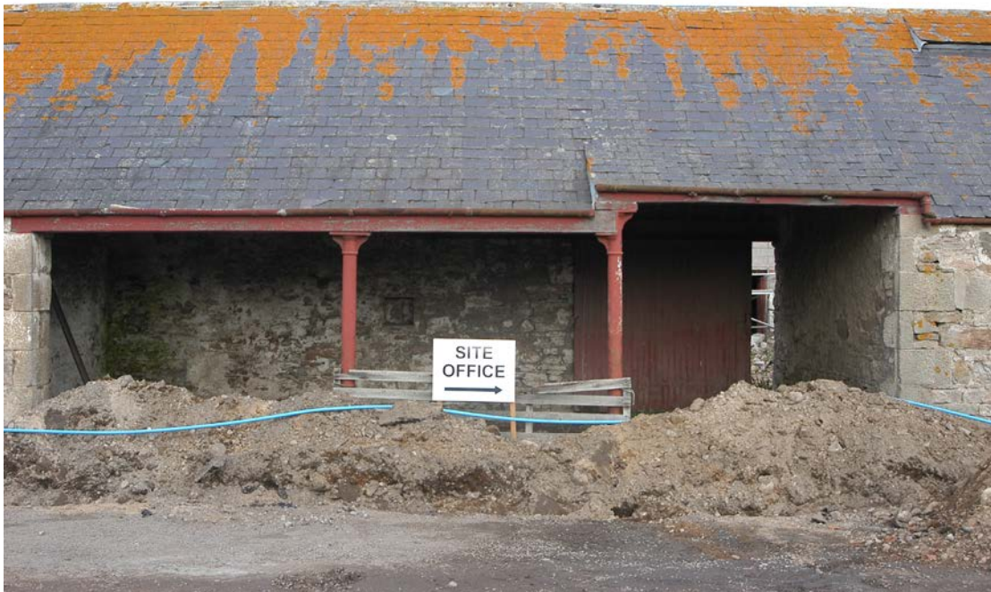
Plate 7 Three-bay cart shed in the middle of the south range
