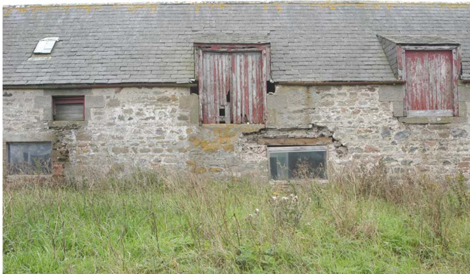
Plate 2 North range, north facing elevation, middle section
