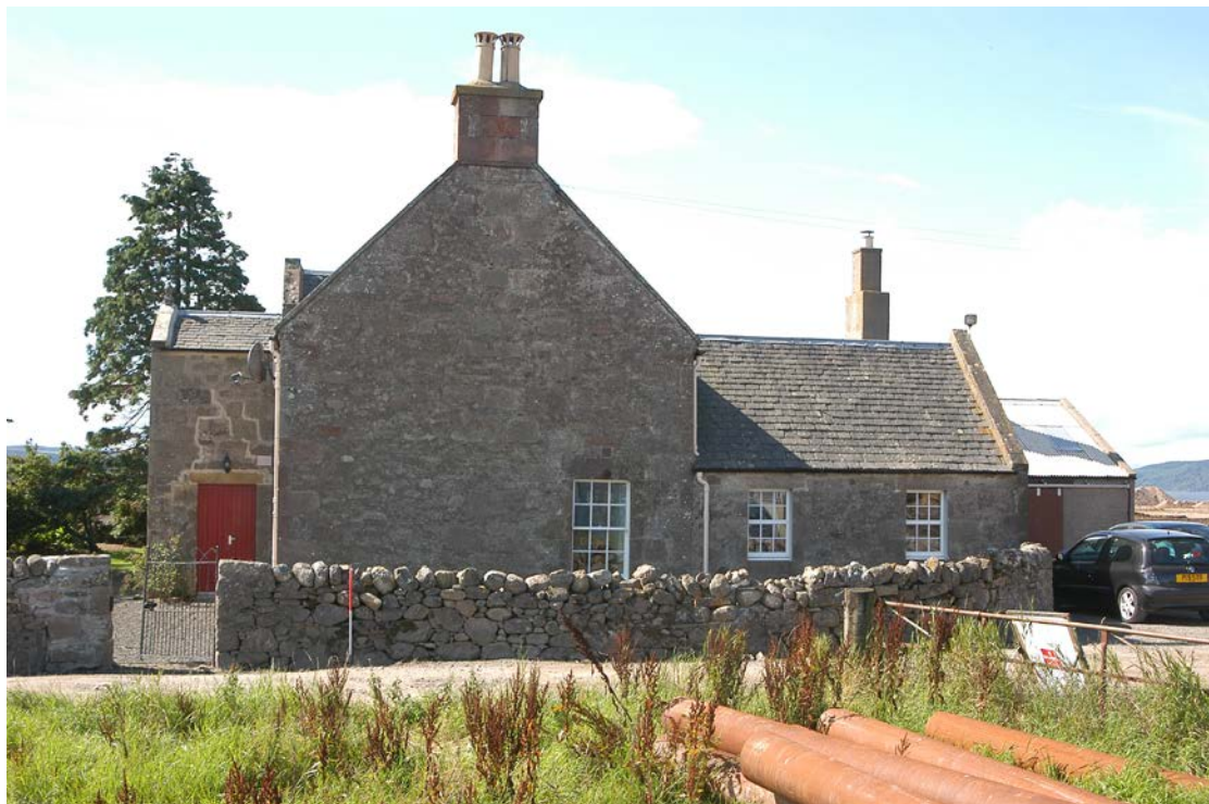
Plate 11 Balnaglack farmhouse, north elevation
