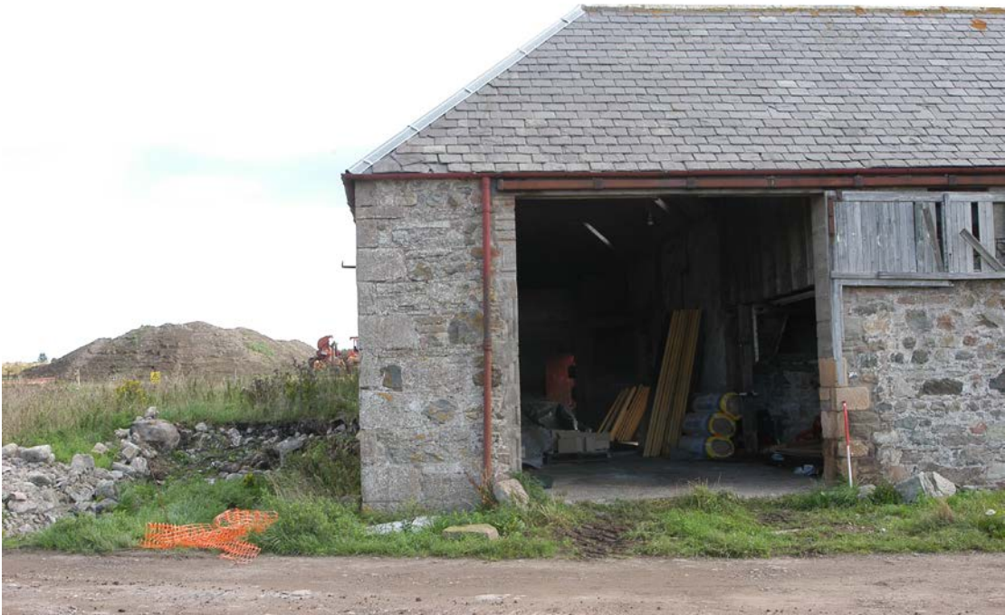
Plate 8 Main entrance to the single-ailed barn on the west range
