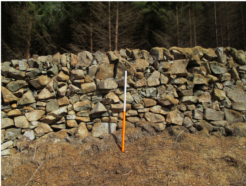
Fig. 3 - Photograph showing wall height and condition of Site 183
