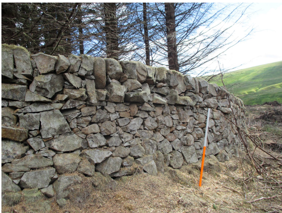
Fig. 5 - Photograph showing wall height and condition of Site 181
