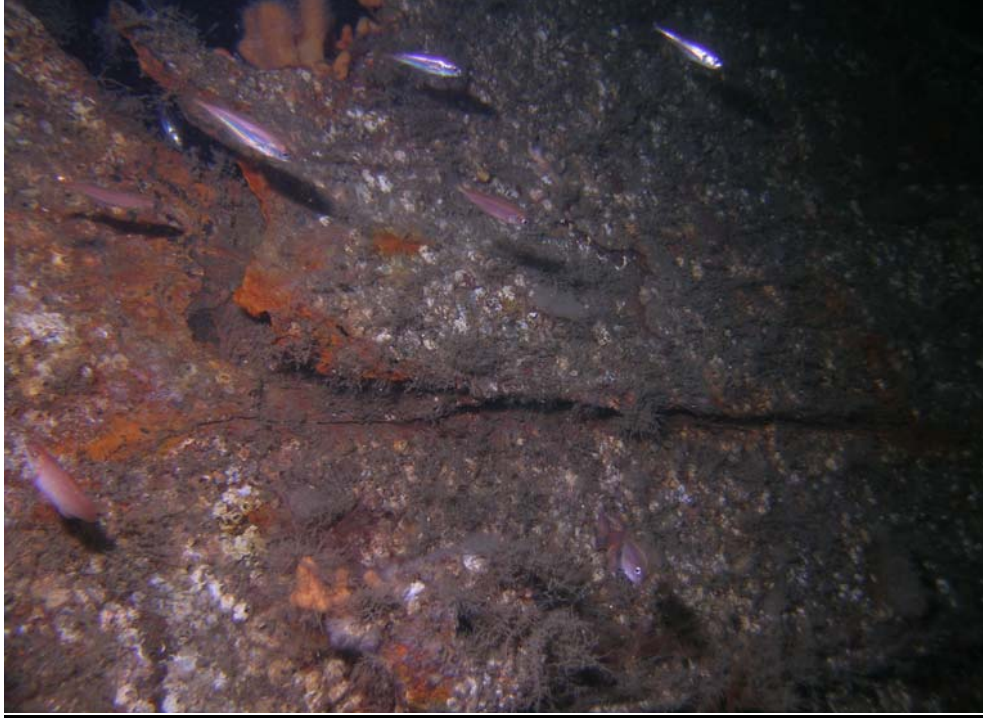
Figure 4.13: Image of overlapping hull plates on SMS Cöln showing corrosion where plates have separated.
