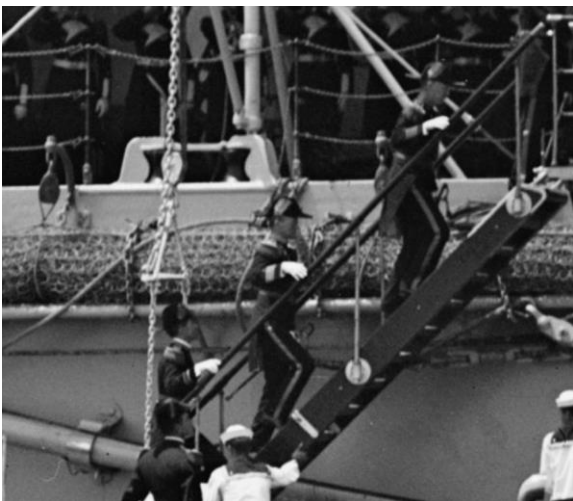
Plate 11: Archive images of a gangway in use on SMS Moltke (G. Staff Collection). Note The brass fittings at the top of each side member of the gangway (circled, left) and the brass sockets support for hand rail stanchion (right).
