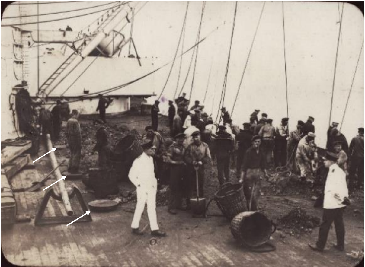
Plate 20: Archive image of coal loading on the SMS Von der Tann (G. Staff Collection). Note the three circular deck hatches (arrows) that would be lifted to allow coal to drop into the bunkers.
