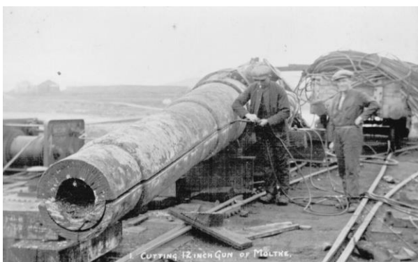
Plate 7: Cutting up one of SMS Moltke's 12-inch guns at Lyness from one of the two turrets left behind in Orkney (B Forbes Collection).
