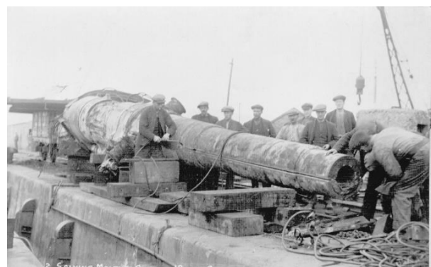
Plate 7: Cutting up one of SMS Moltke's 12-inch guns at Lyness from one of the two turrets left behind in Orkney (B Forbes Collection).
