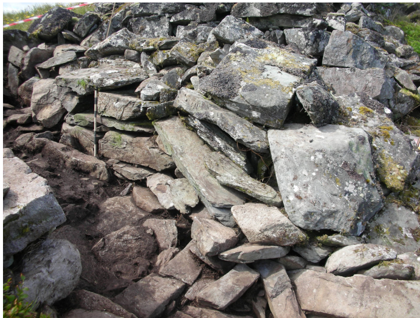
Collapsed Wall [006] from NE
