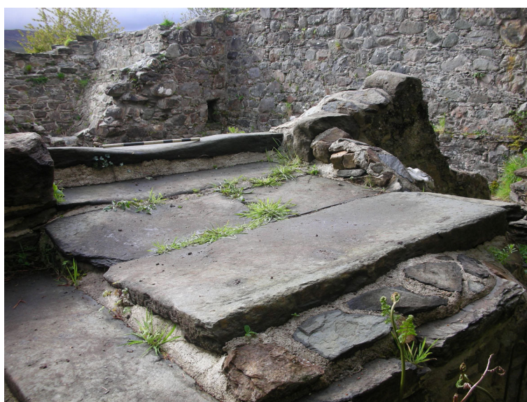
Stair landing at stones-floor level
