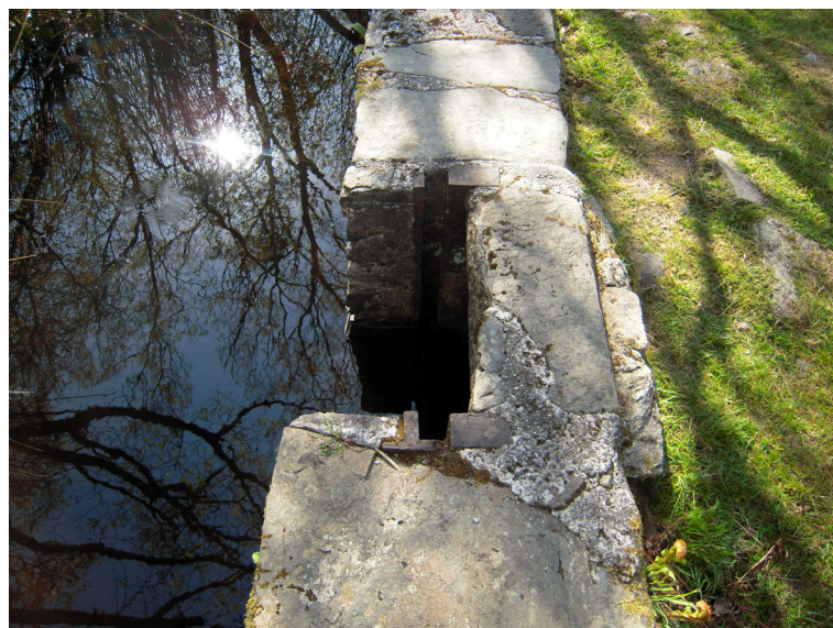
Lade sluice gate
