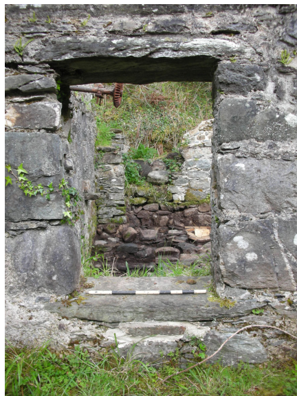
Ground floor window in SE wall
