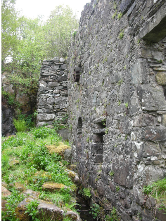
Lade wall and pier
