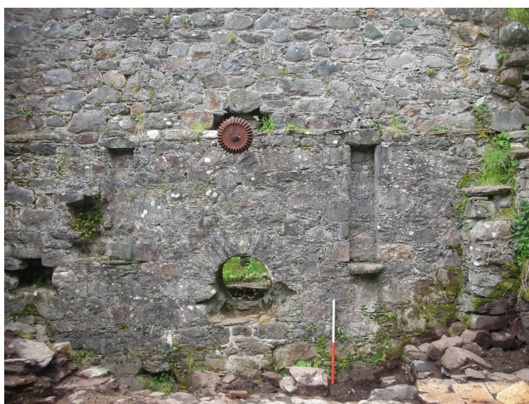
Vertical timber slots, axle hole and upper gearing
