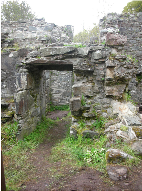
Ground floor door into kiln
