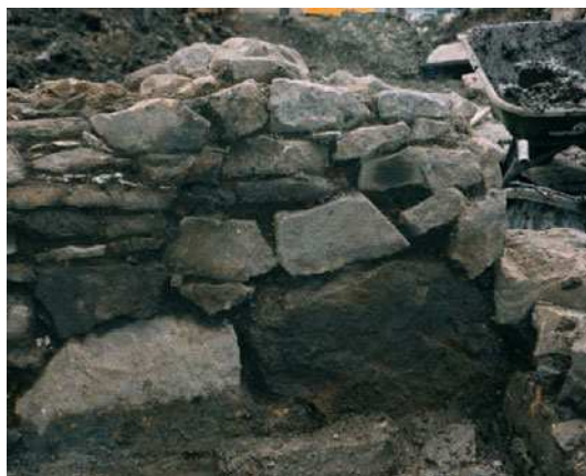
Plate 2. Rebuilt masonry in the east wall
