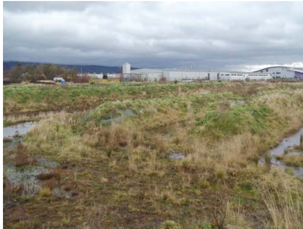
Plate 1 - Shot of remediation bunds on site
