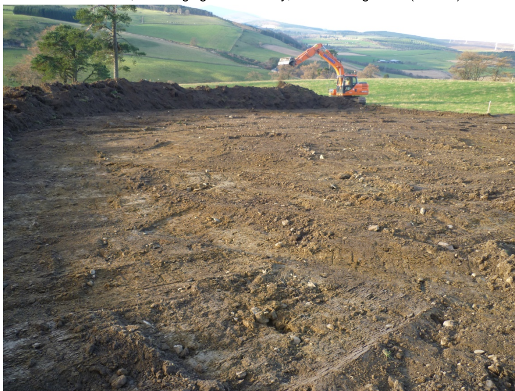
Plate 1 – Topsoil strip of T1 crane pad and turbine base
