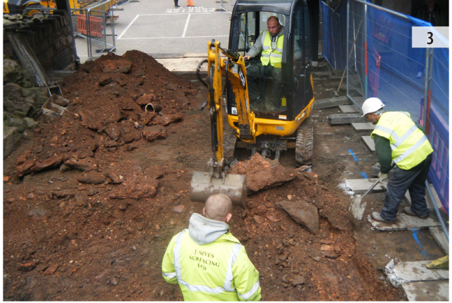
ILLUS 2 Working shot showing sand levelling layer beneath slabs ILLUS 3 Working shot showing red blaes across whole area
