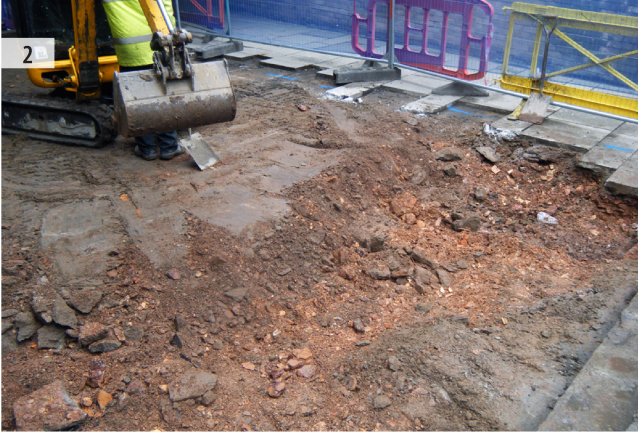
ILLUS 2 Working shot showing sand levelling layer beneath slabs ILLUS 3 Working shot showing red blaes across whole area
