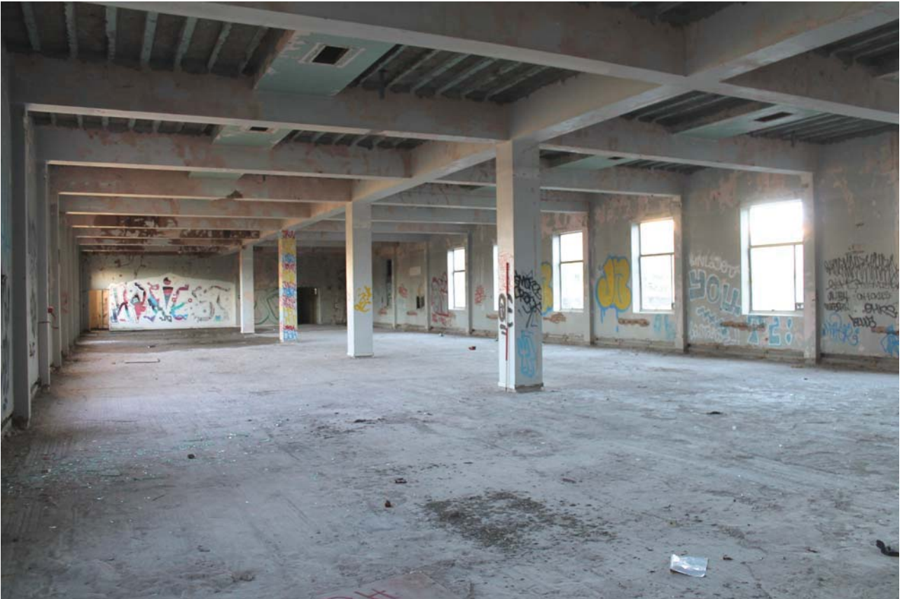
Plate 21: North Wing, ground floor, general view from the south-west
