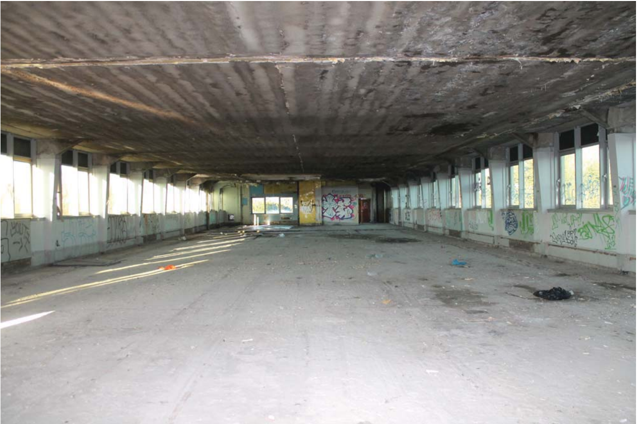
Plate 23: North Wing, third floor, general view from the south
