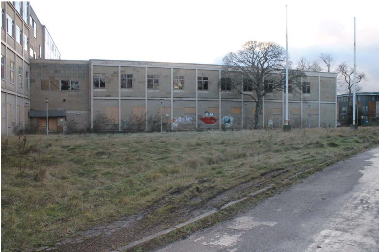
Plate 4: West Wing, general view of the north elevation from the north
