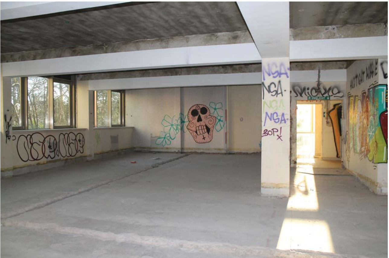
Plate 24: South Wing, ground floor, general view from the north-east
