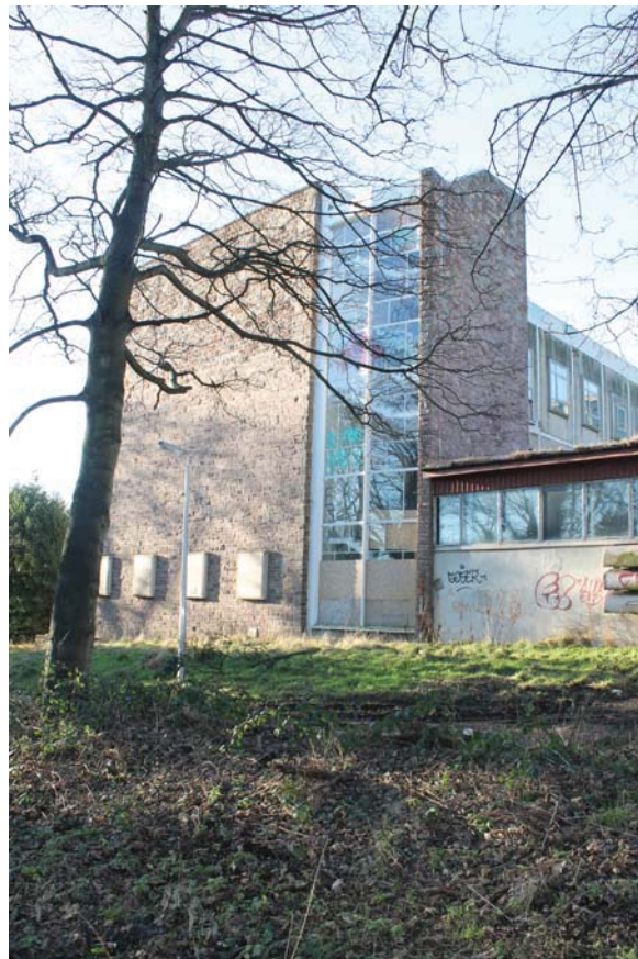
Plate 10: East Wing, general view of east elevation from the north-east
