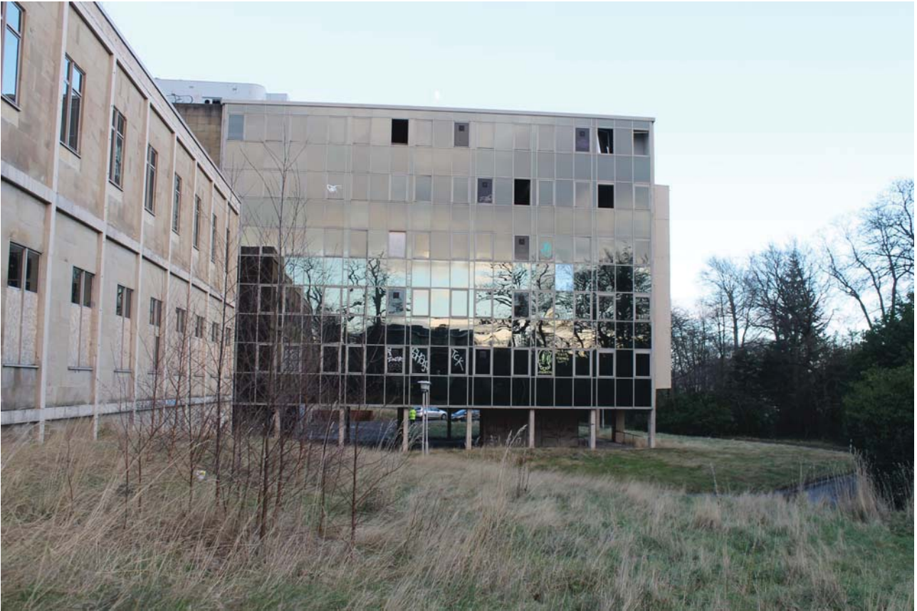
Plate 9: South Wing, general view of the west elevation from the west
