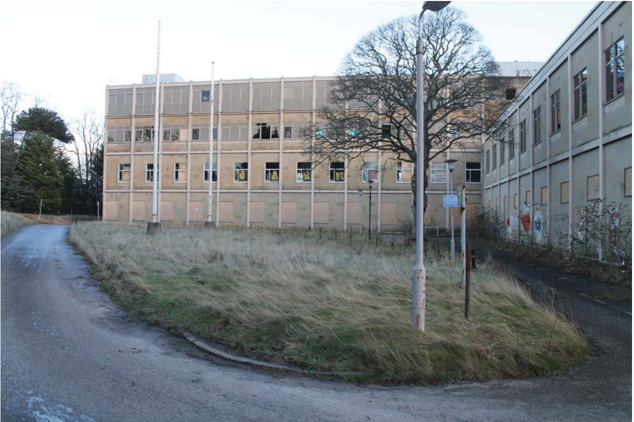
Plate 5: North Wing, general view of the west elevation from the west
