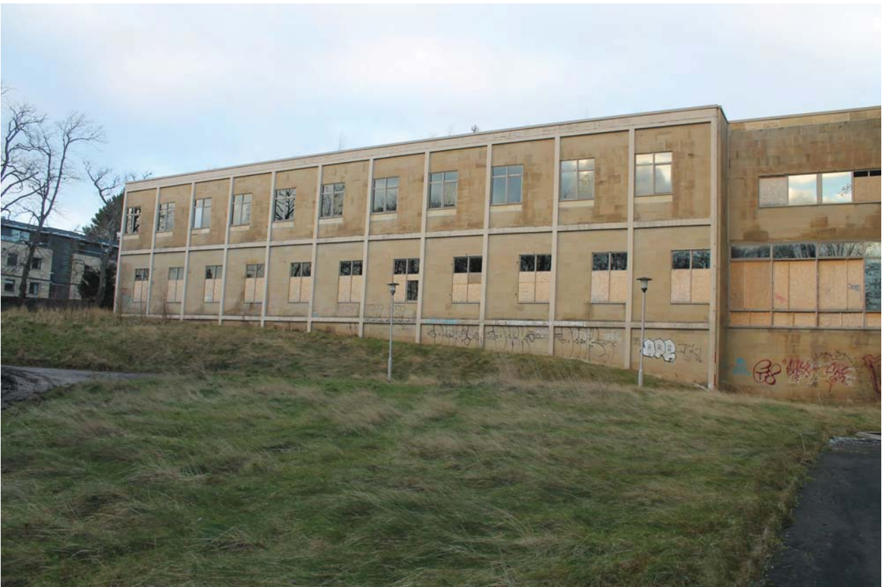
Plate 2: West Wing, general view of the south elevation from the south-east
