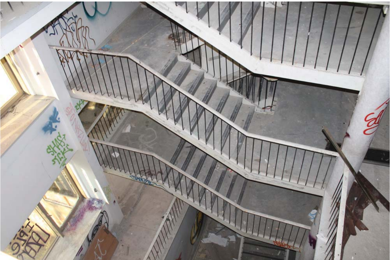
Plate 26: Detail of the central stair looking down from the south-east
