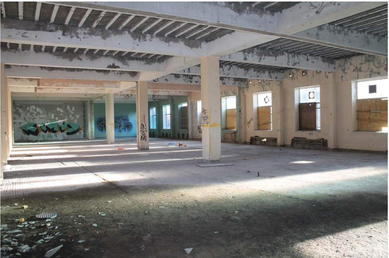
Plate 22: East Wing, ground floor, general view from the south-west
