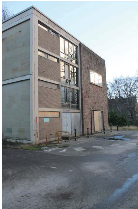
Plate 17: West Wing, general view of the west elevation from the north-west
