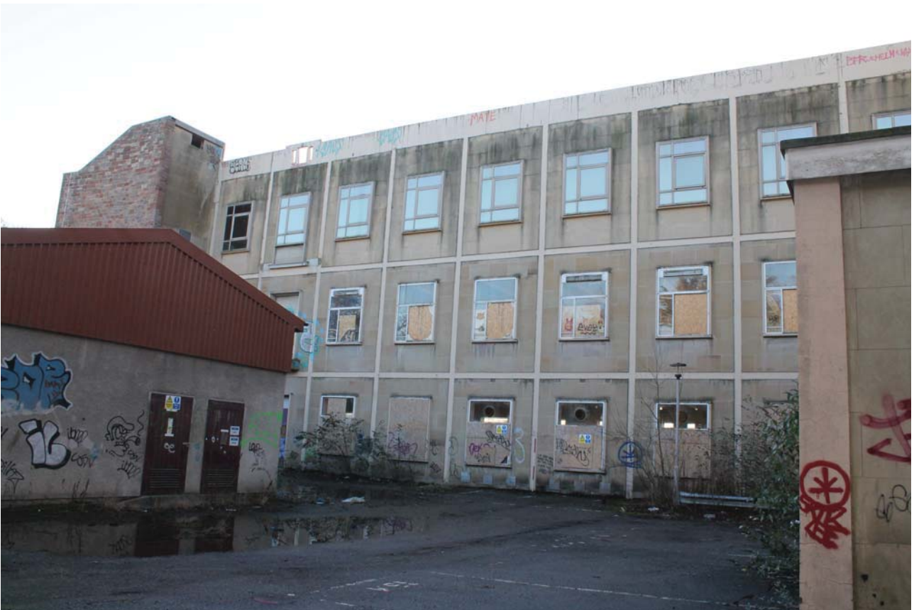
Plate 13: East Wing, general view of the north elevation from the north-east
