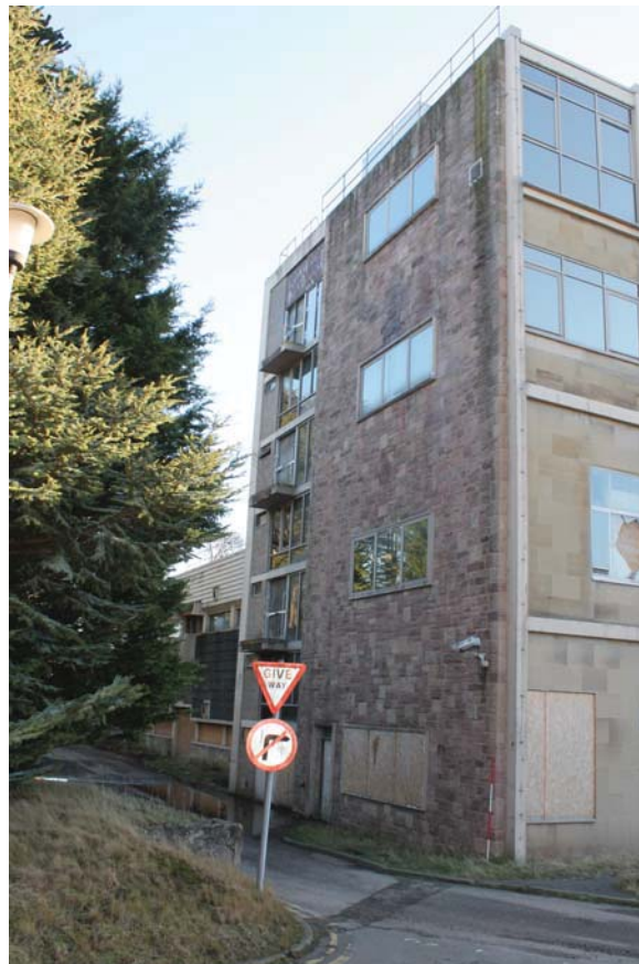
Plate 16: North Wing, general view of the north elevation from the north-west
