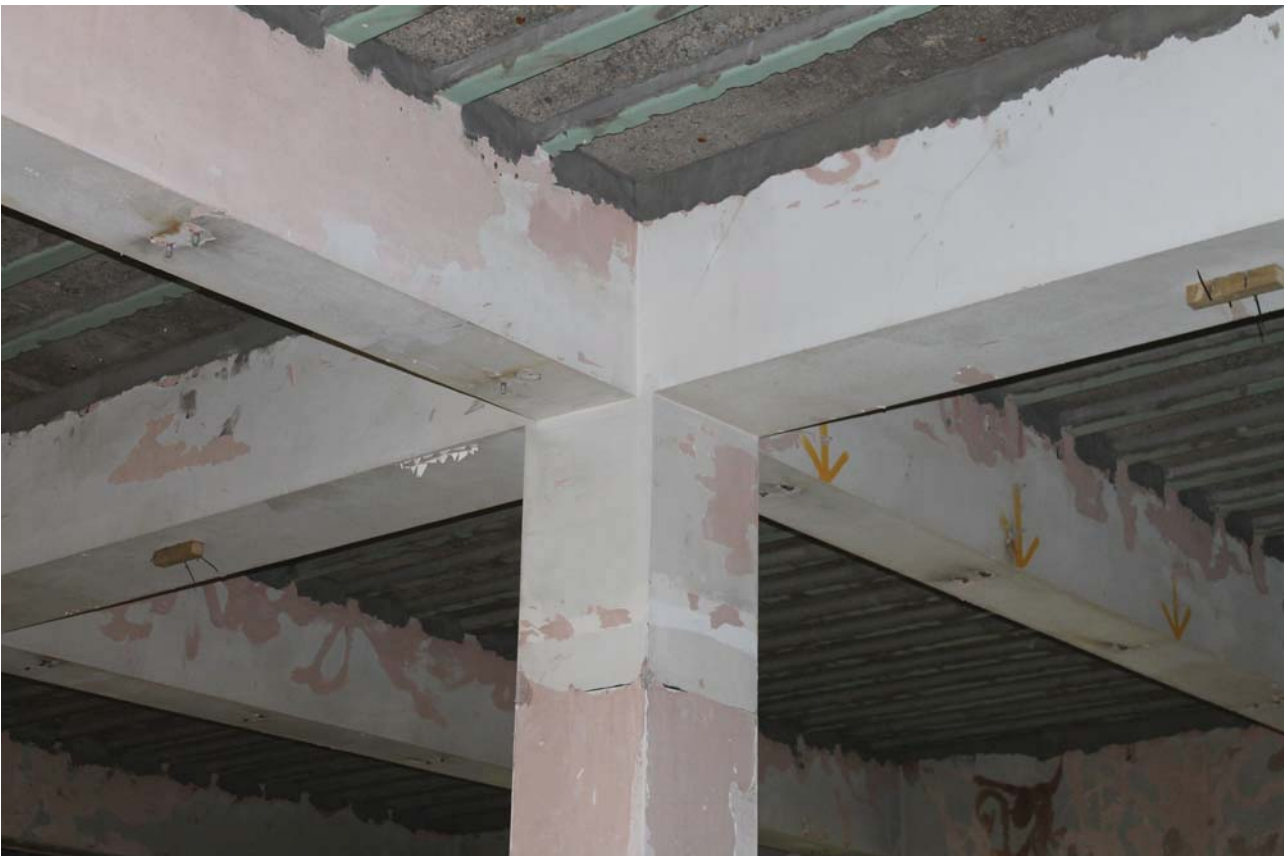
Plate 20: West Wing, ground floor, detail of the concrete column and beams
