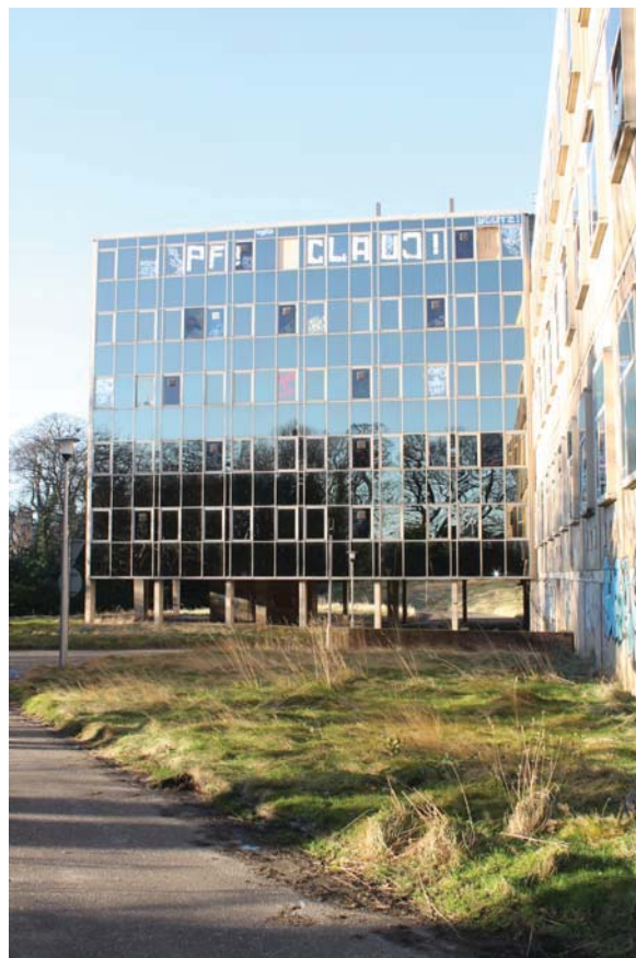
Plate 8: South Wing, general view of the east elevation from the east
