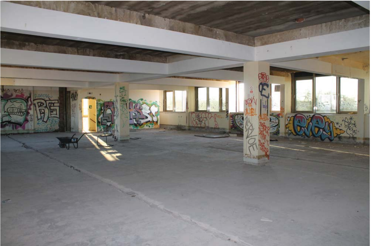
Plate 25: South Wing, first floor, general view from the north-west
