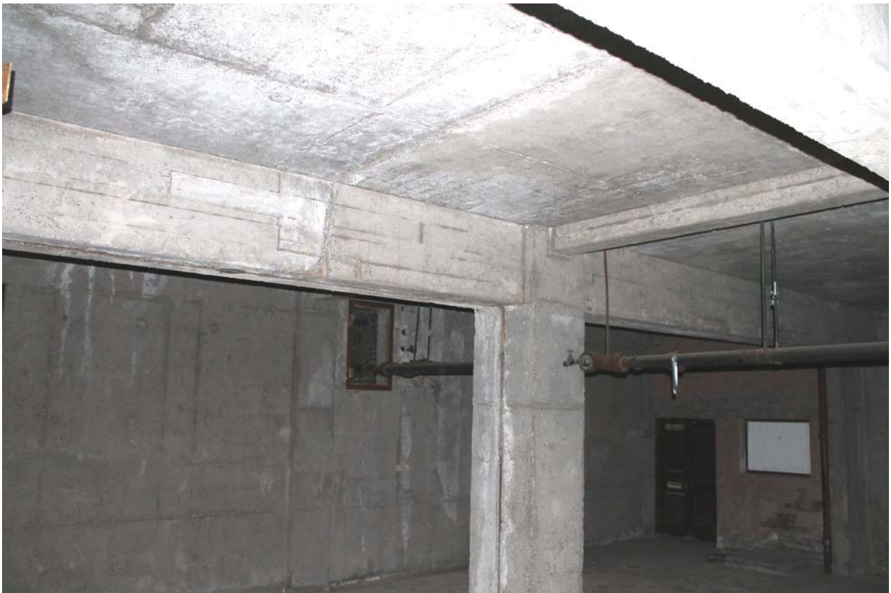
Plate 18: Basement, detail of concrete superstructure
