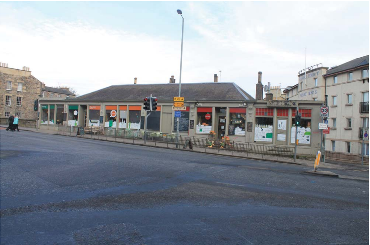
Plate 2: Nos 1 – 6 Canonmills Bridge, general view of the south-west elevation from the south
