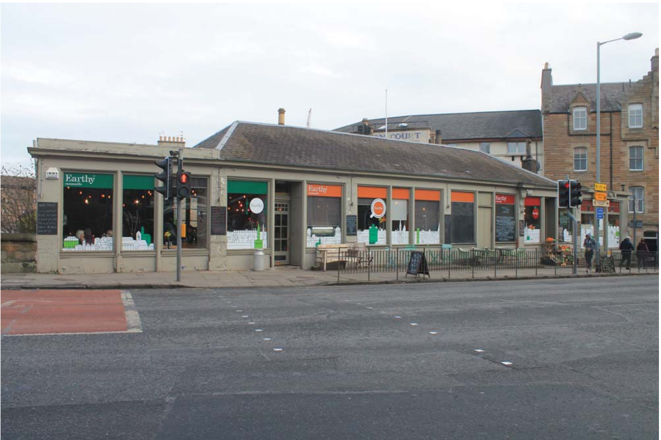
Plate 1: Nos 1 – 6 Canonmills Bridge, general view of the south-west elevation from the west
