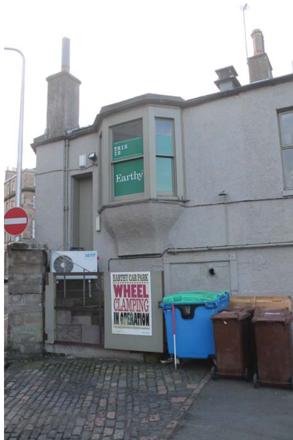
Plate 10: No 2 Canonmills Bridge, general view of the north-east elevation from the east
