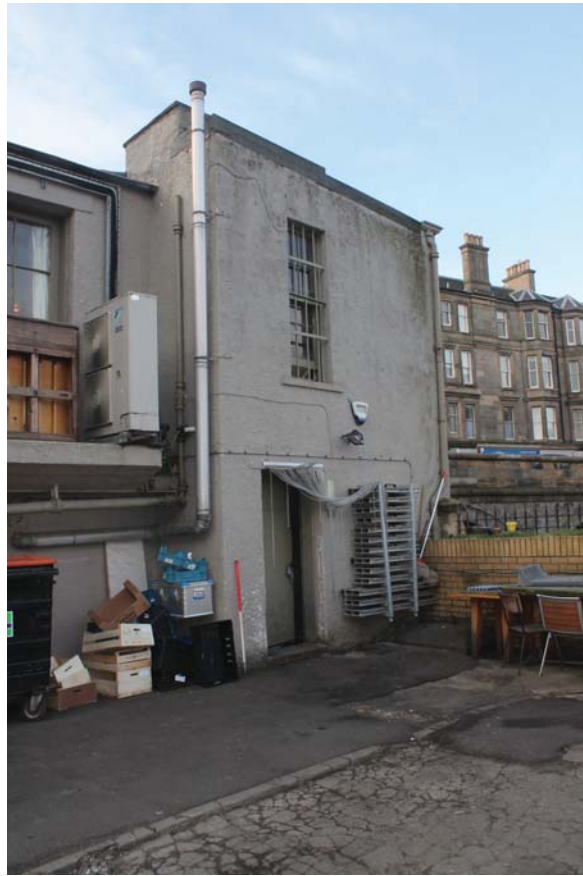
Plate 11: No 6 Canonmills Bridge, general view of the north-east elevation from the east
