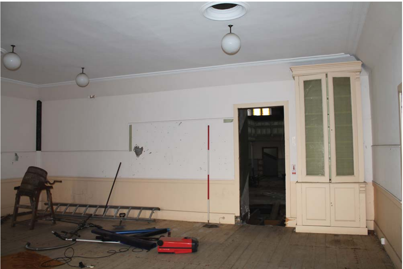
Plate 49: Room 0/3, general view from the SEE
