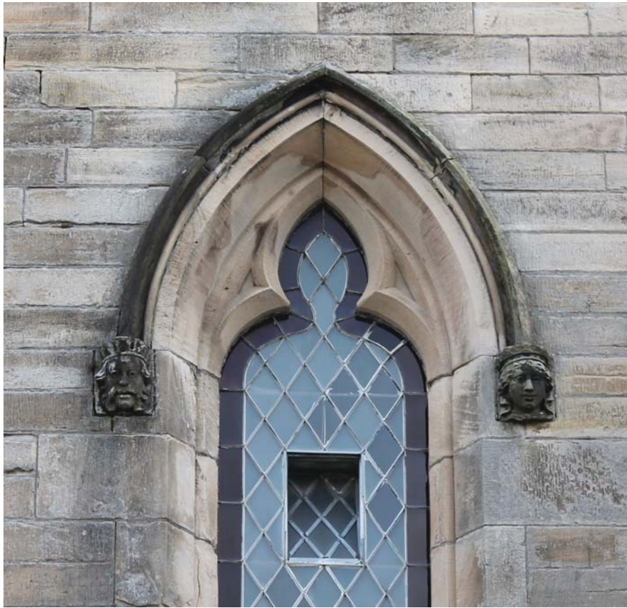
Plate 23: South-west elevation, detail of hood mould over north-westernmost window from the south-west
