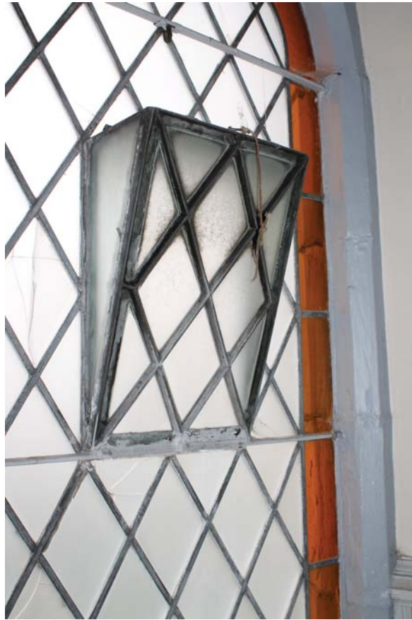
Plate 71: Room 1/1, detail of louvered window of the main window in the north-east wall from the west
