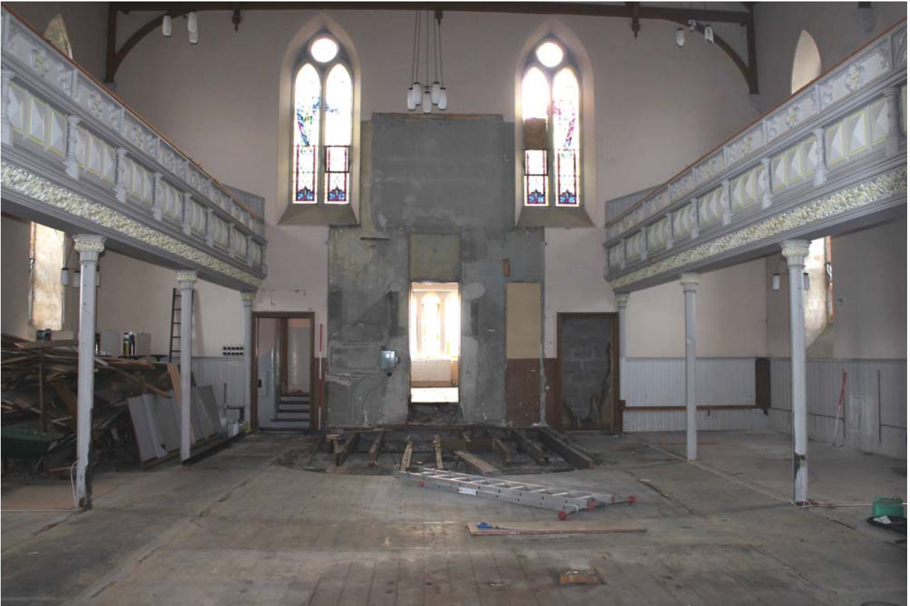
Plate 41: Room 0/1, general view from the north-west
