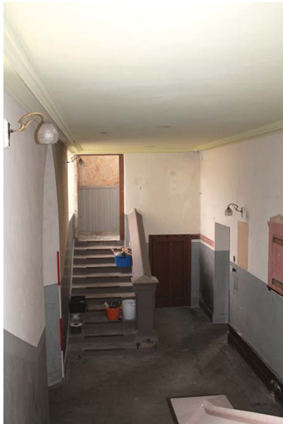
Plate 56: Room 0/5, general view from the south-west
