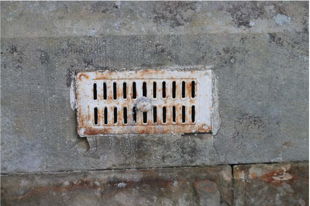
Plate 29: South-west elevation, detail of vent below window from the south-west
