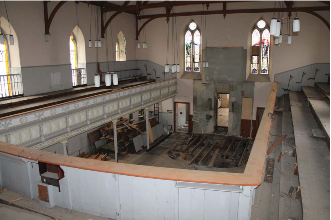
Plate 65: Room 1/1, general view from the west
