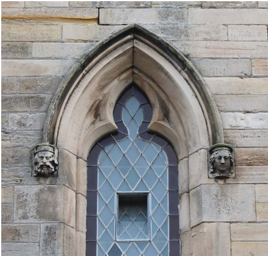
Plate 24: South-west elevation, detail of hood mould over second north-westernmost window from the south-west
