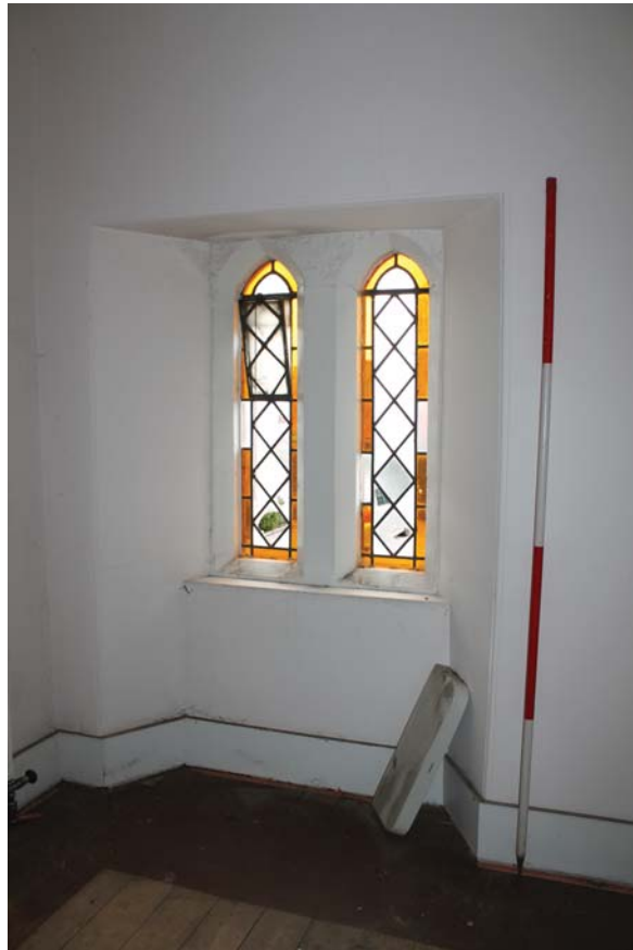
Plate 53: Room 0/4, detail of windows in the south-east wall, from the NWW
