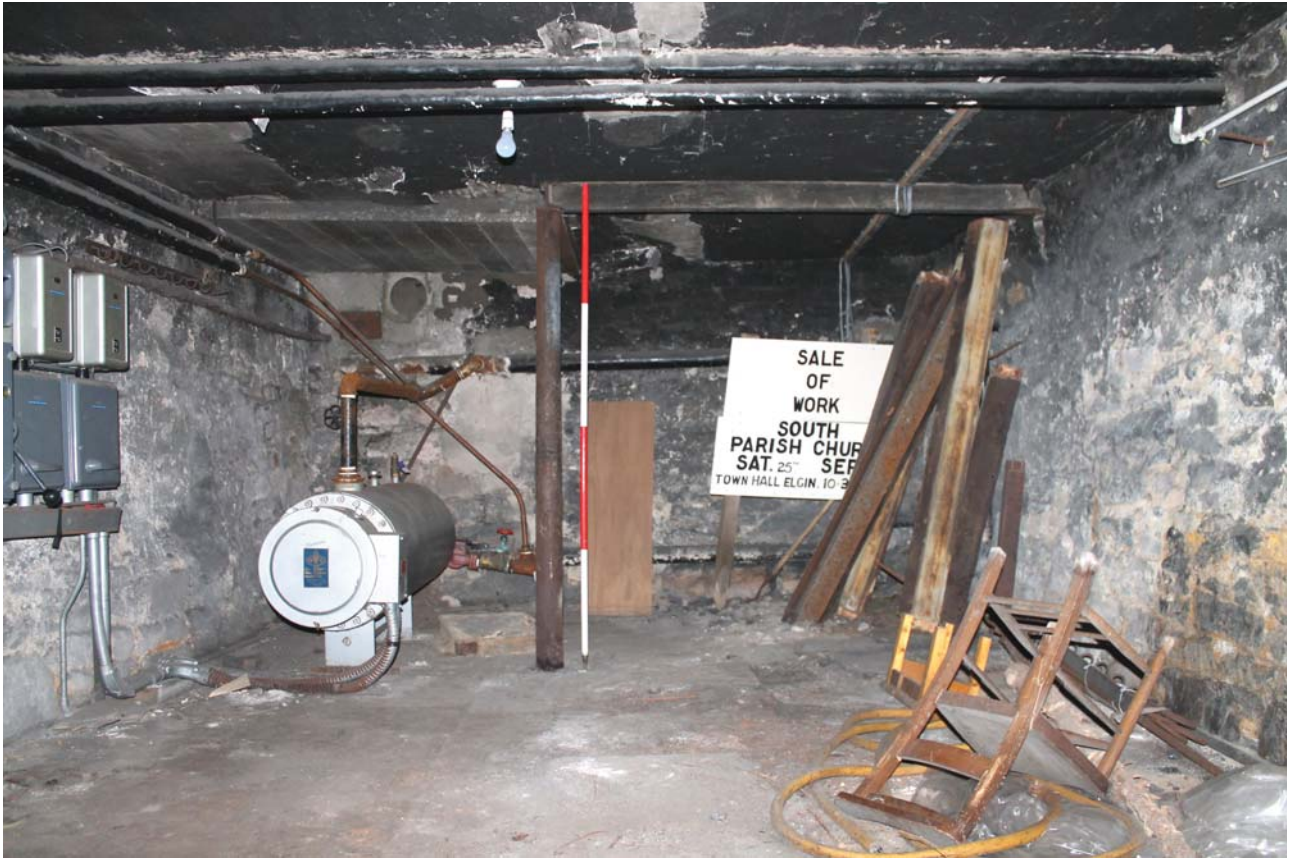
Plate 39: Room -1/1, general view from the south-east
