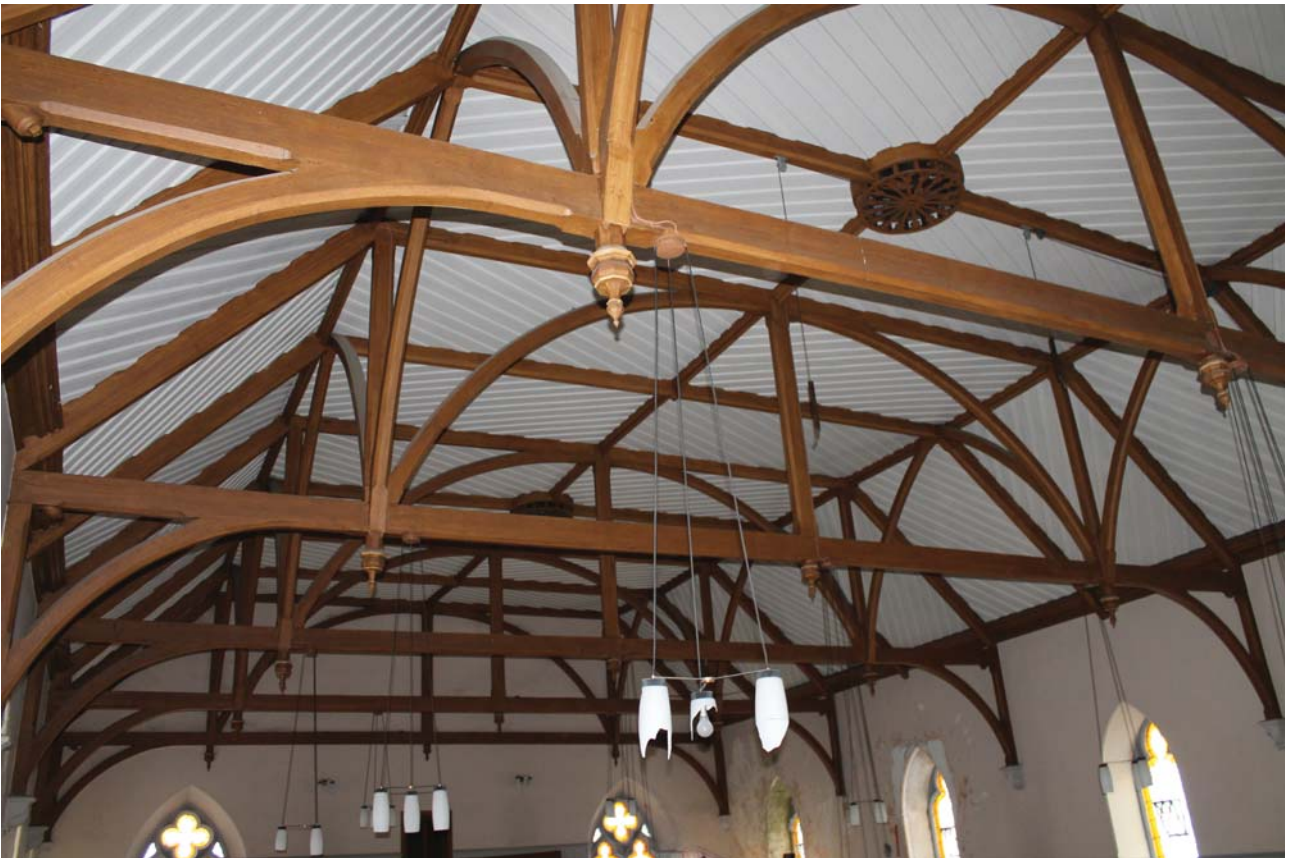
Plate 68: Room 1/1, general view of roof from the north
