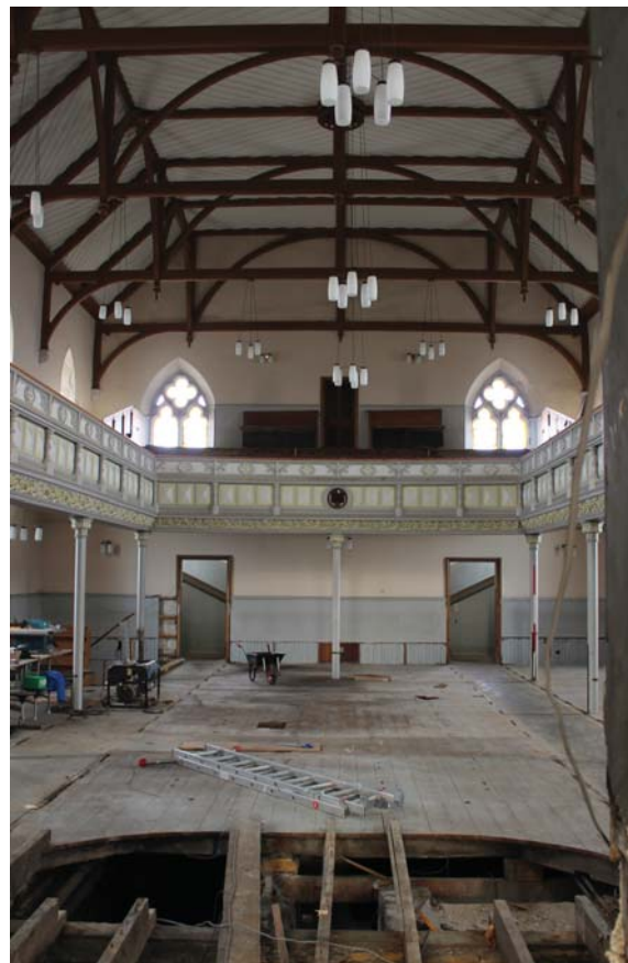
Plate 40: Room 0/1, general view from the south-east
