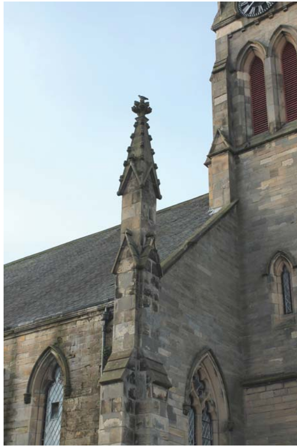
Plate 17: North-east elevation, detail of corner buttress from the north
