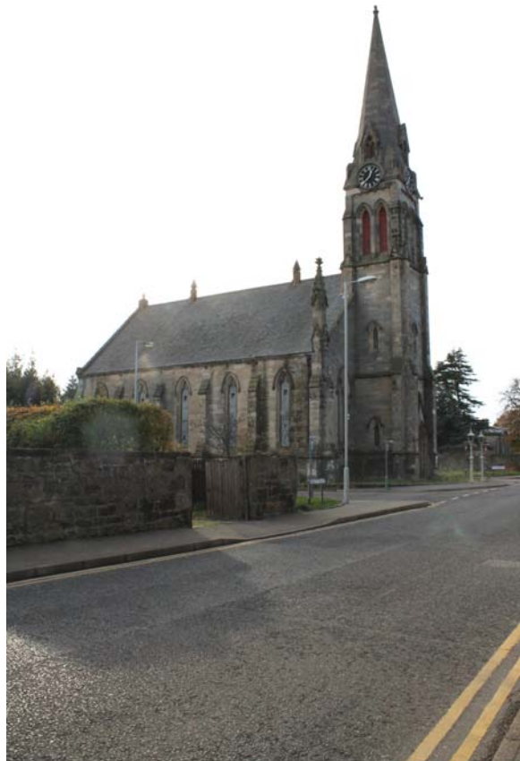
Plate 2: General view from the north
