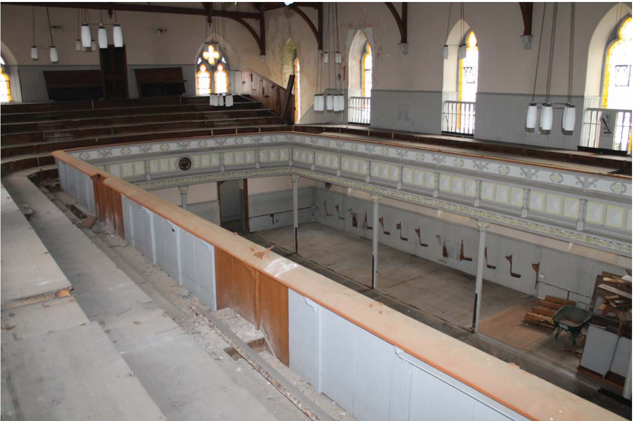
Plate 66: Room 1/1, general view from the south
