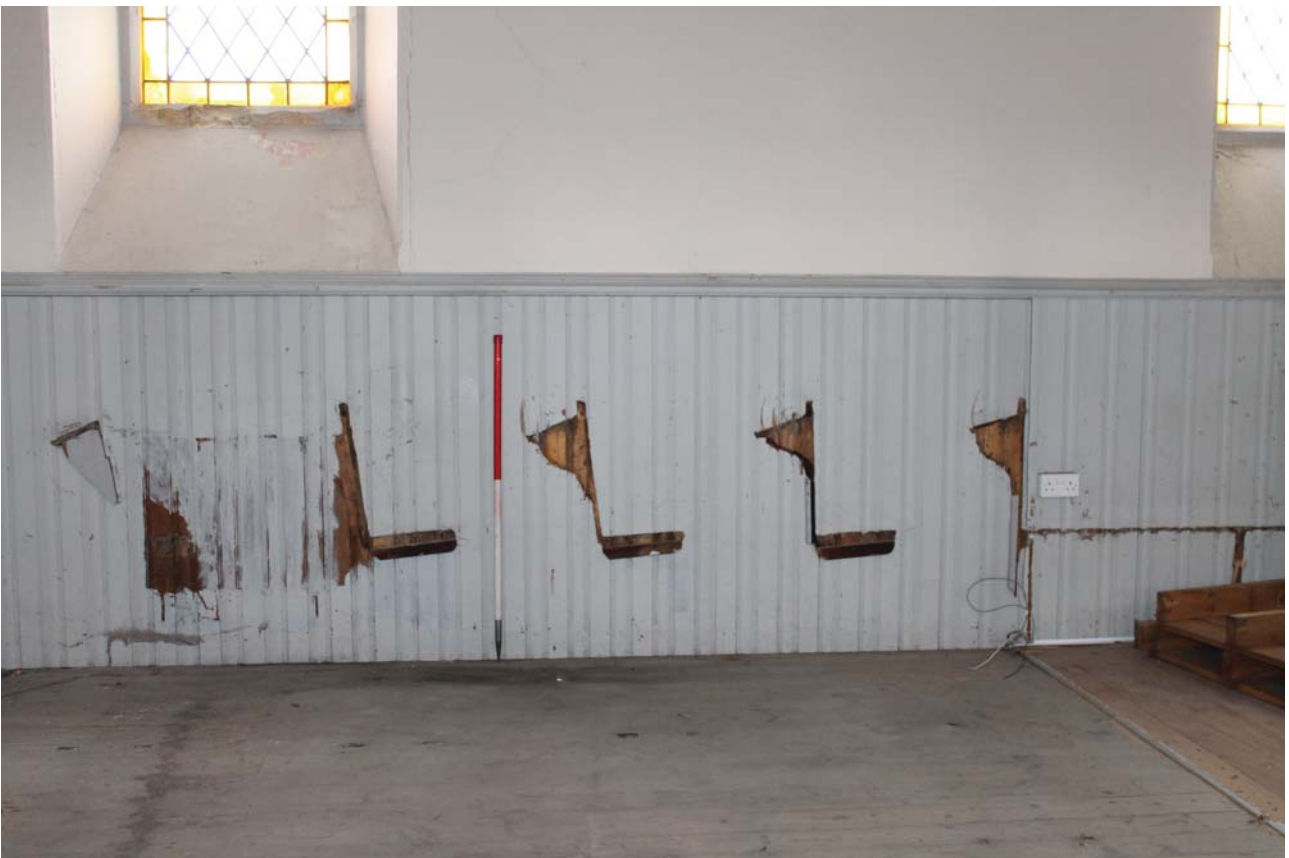
Plate 46: Room 0/1, detail of the shapes of the pews leftover after their removal on the timber panelling of the north-east wall, from the south-west
