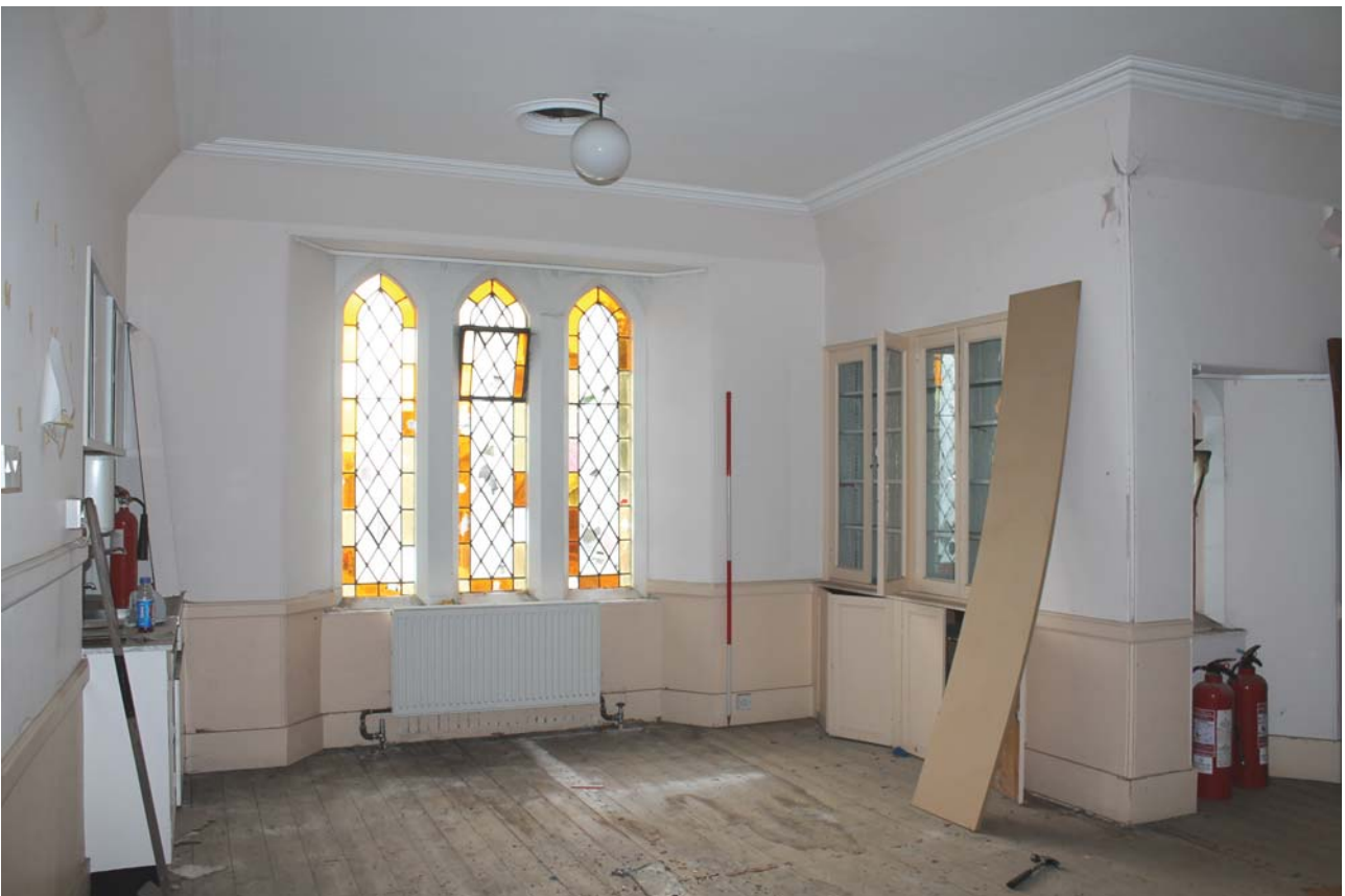
Plate 50: Room 0/3, general view from the NNW
