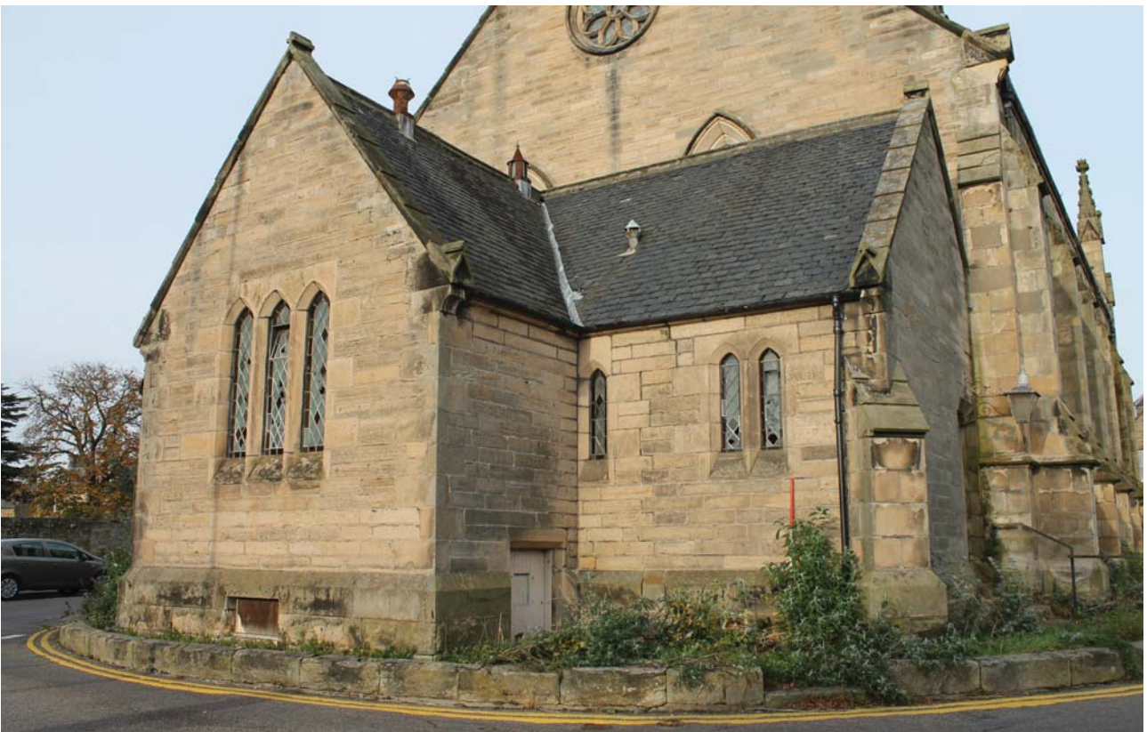
Plate 30: South-east elevation, general view from the east
