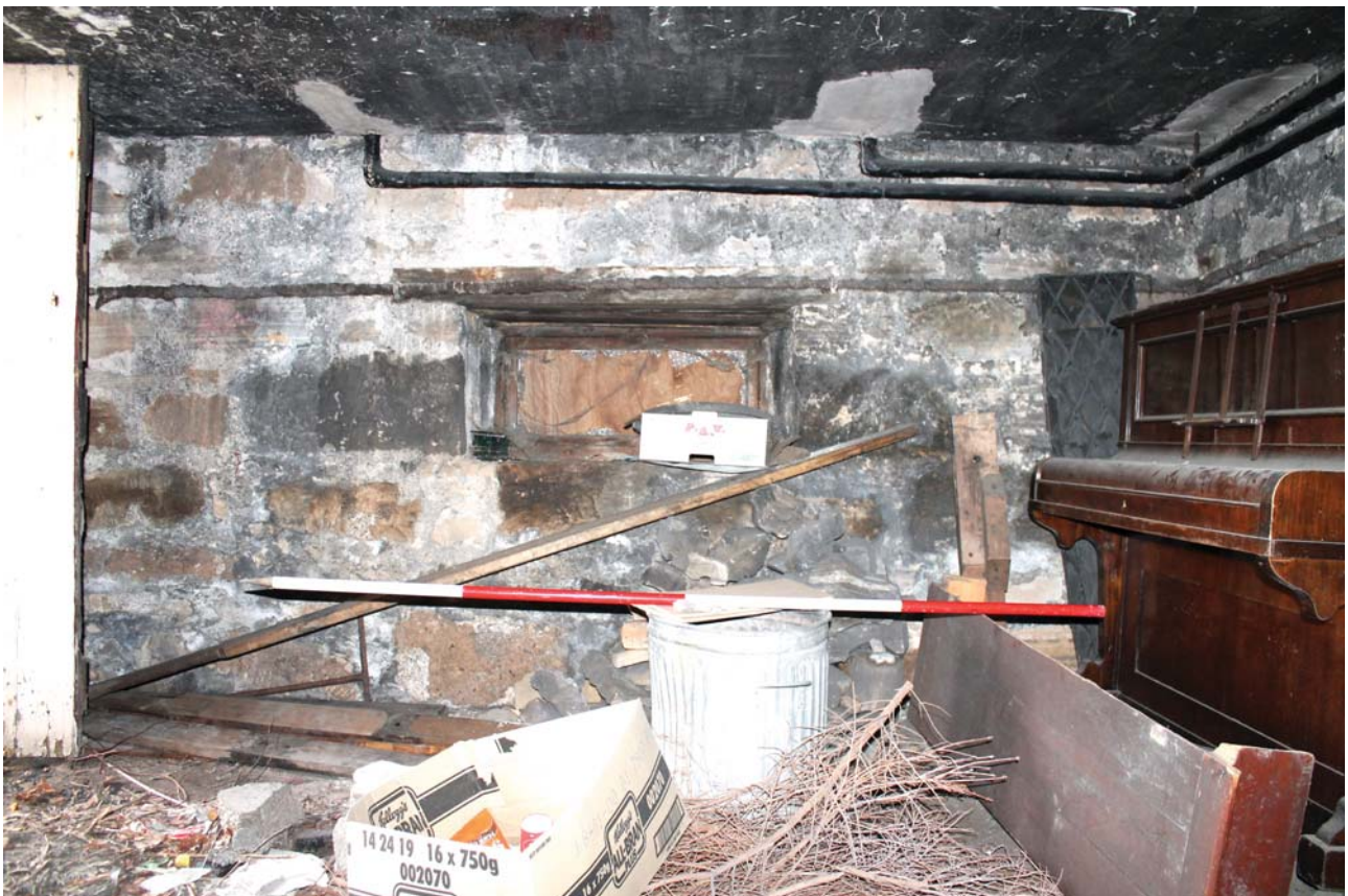
Plate 38: Room -1/1, general view showing boarded-up window from the north-west
