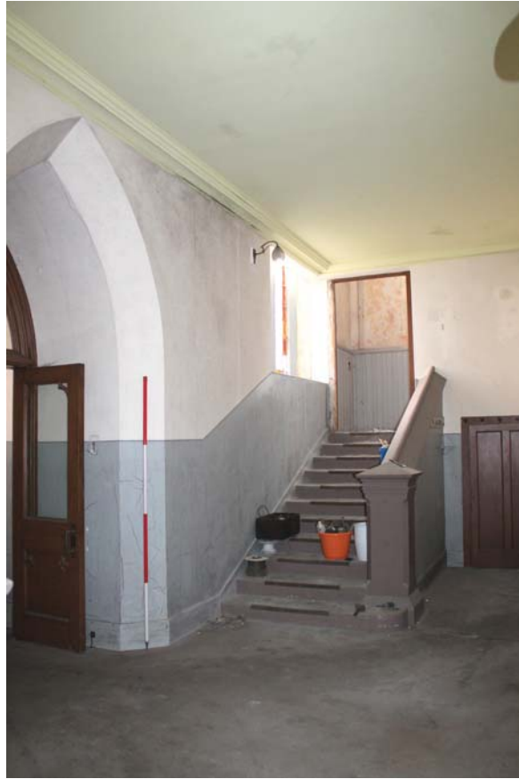
Plate 55: Room 0/5, general view from the south
