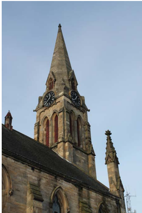
Plate 12: Detail clock tower and spire from the east
