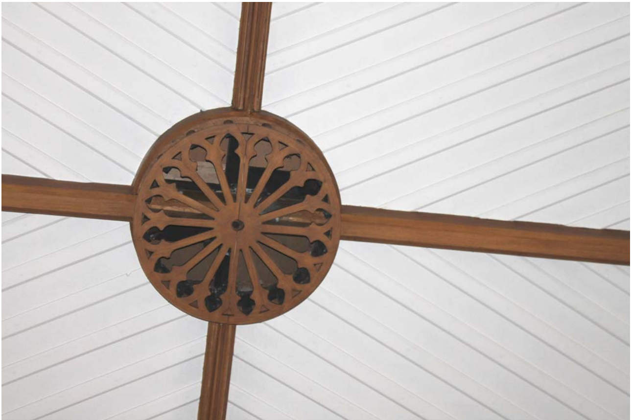
Plate 70: Room 1/1, detail of circular vent in the roof
