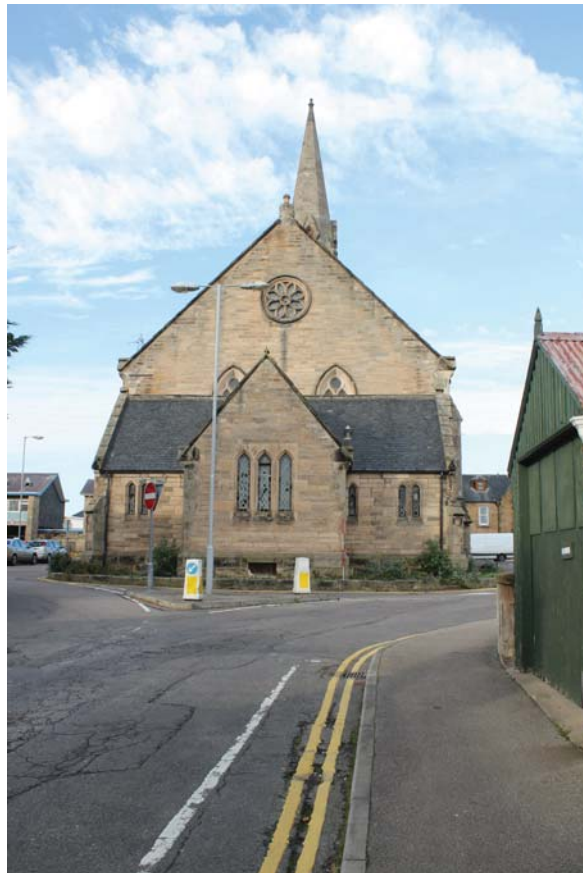
Plate 6: South-east elevation, general view from the south-east
