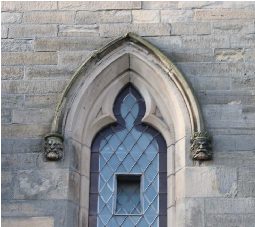
Plate 21: North-east elevation, detail of hood mould over central window from the north-east
