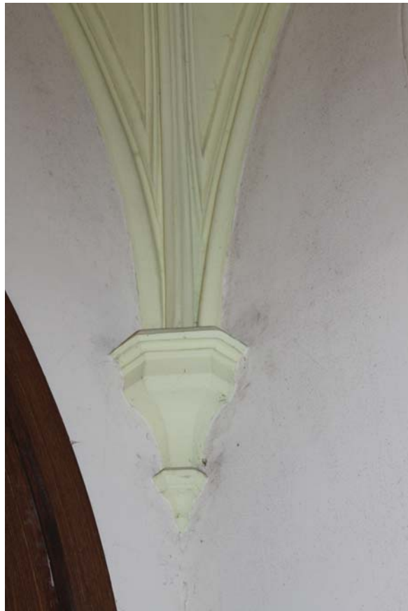
Plate 62: Room 0/5, detail of decorative moulding of porch in the north corner from the south
