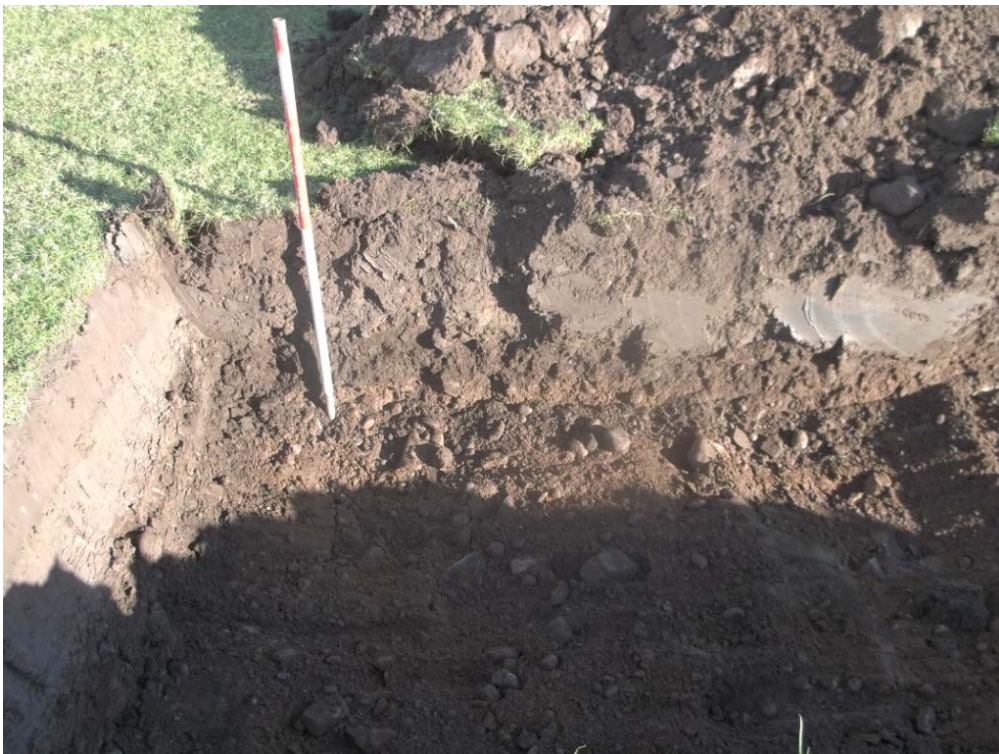
Plate 4 - Original topsoil under made ground in Trench 7
