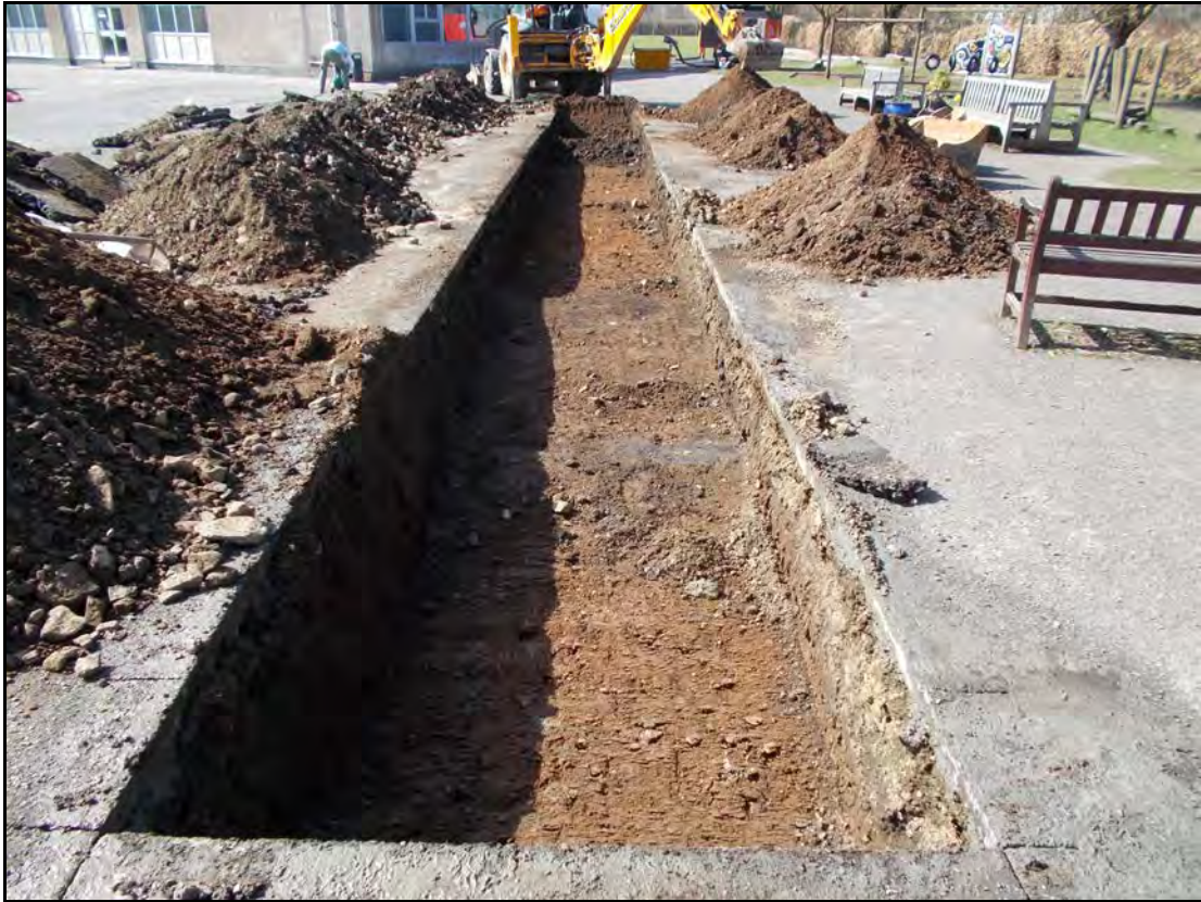
Plate 3 - General view of Trench 1
