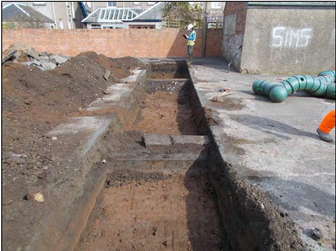
Plate 4 - General view of Trench 2
