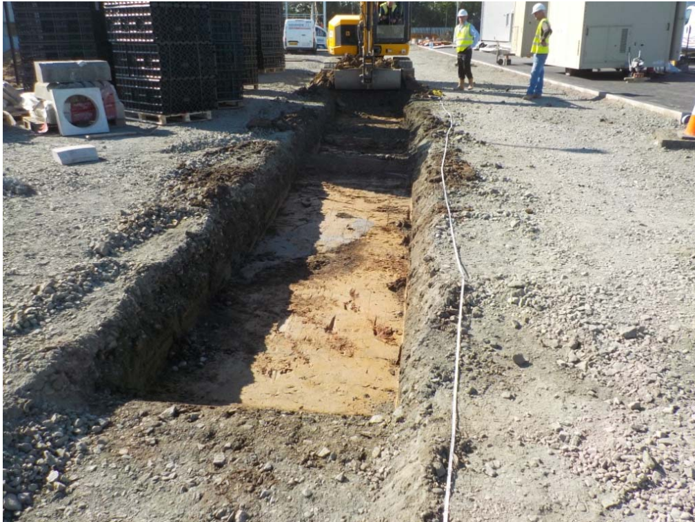
Plate 2 - General view of Trench 1
