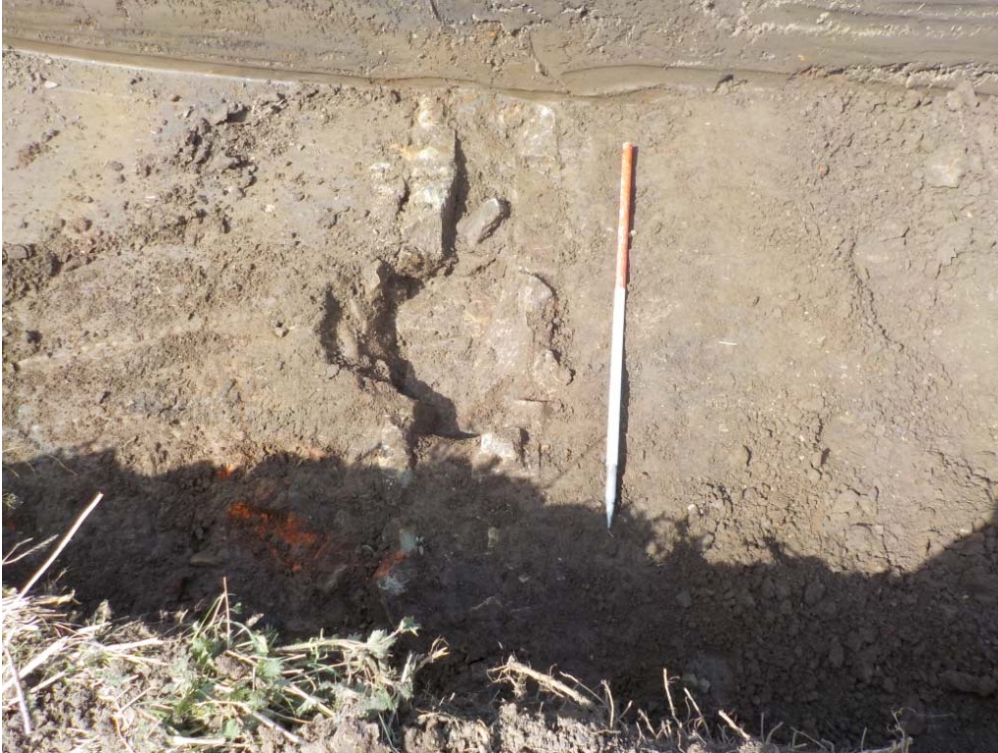
Plate 2 - General view of Culvert [1901]
