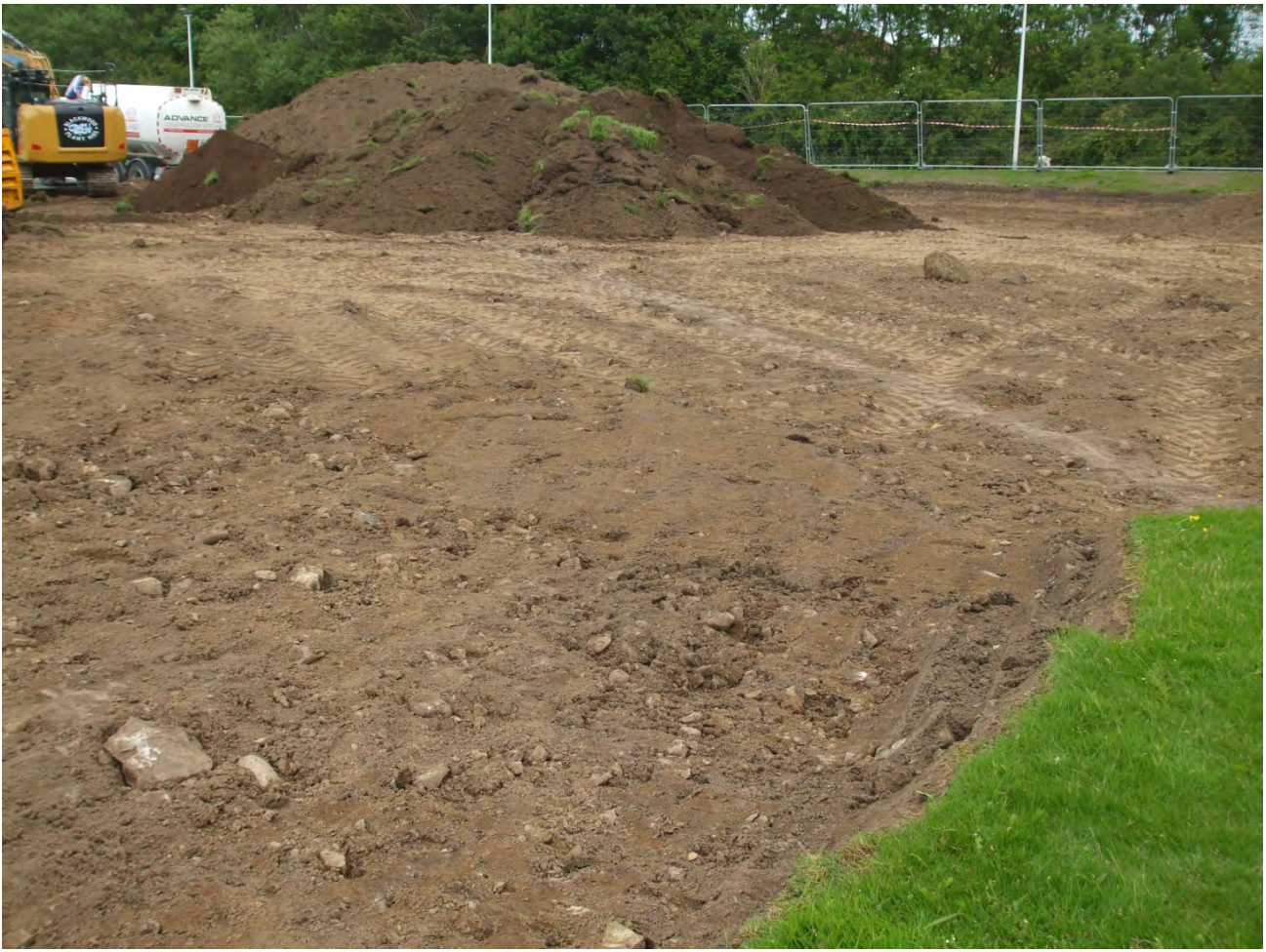
Plate 1: Stripping complete in car park area
