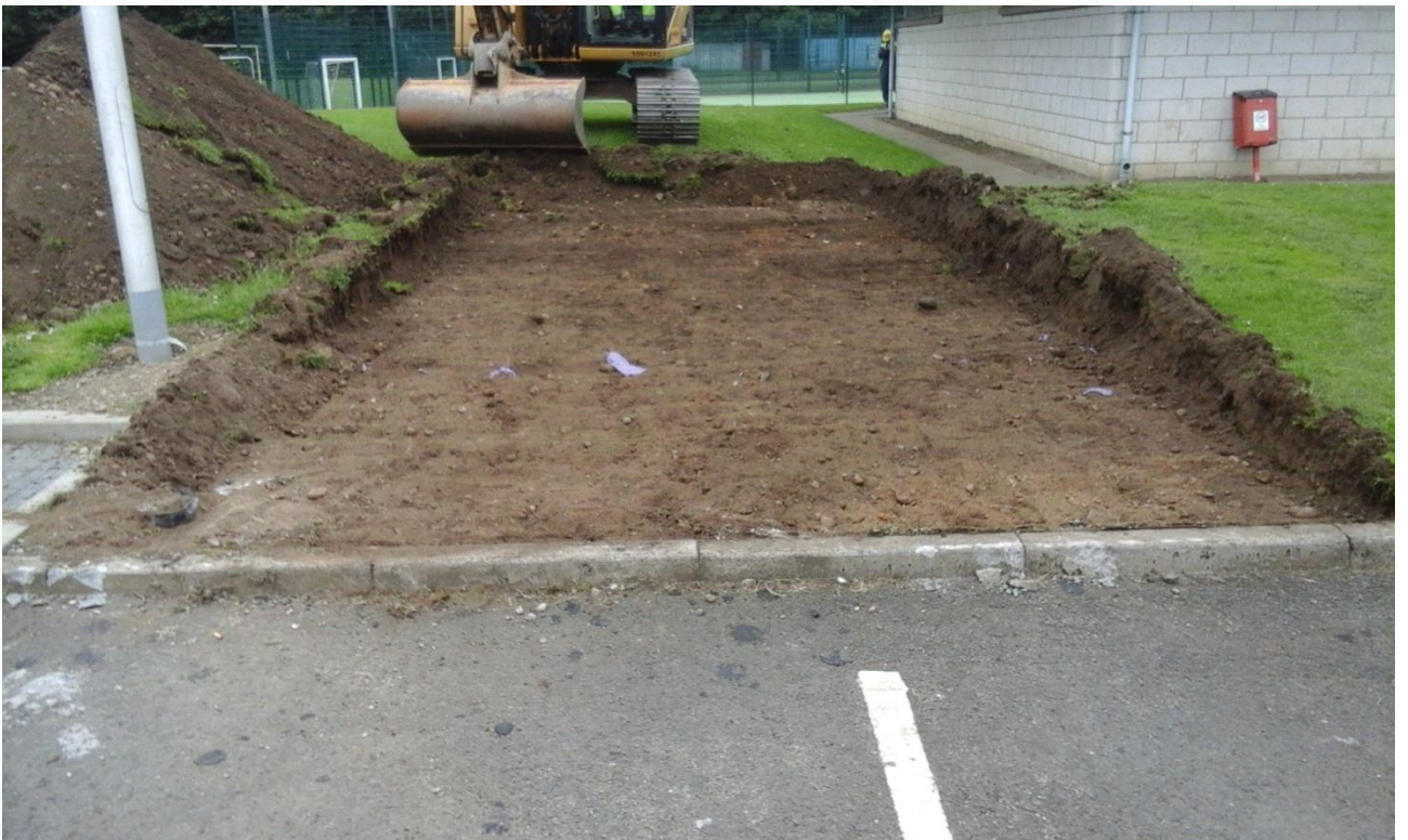
Plate 2: Stripping completed for pavilion extension (from east)
