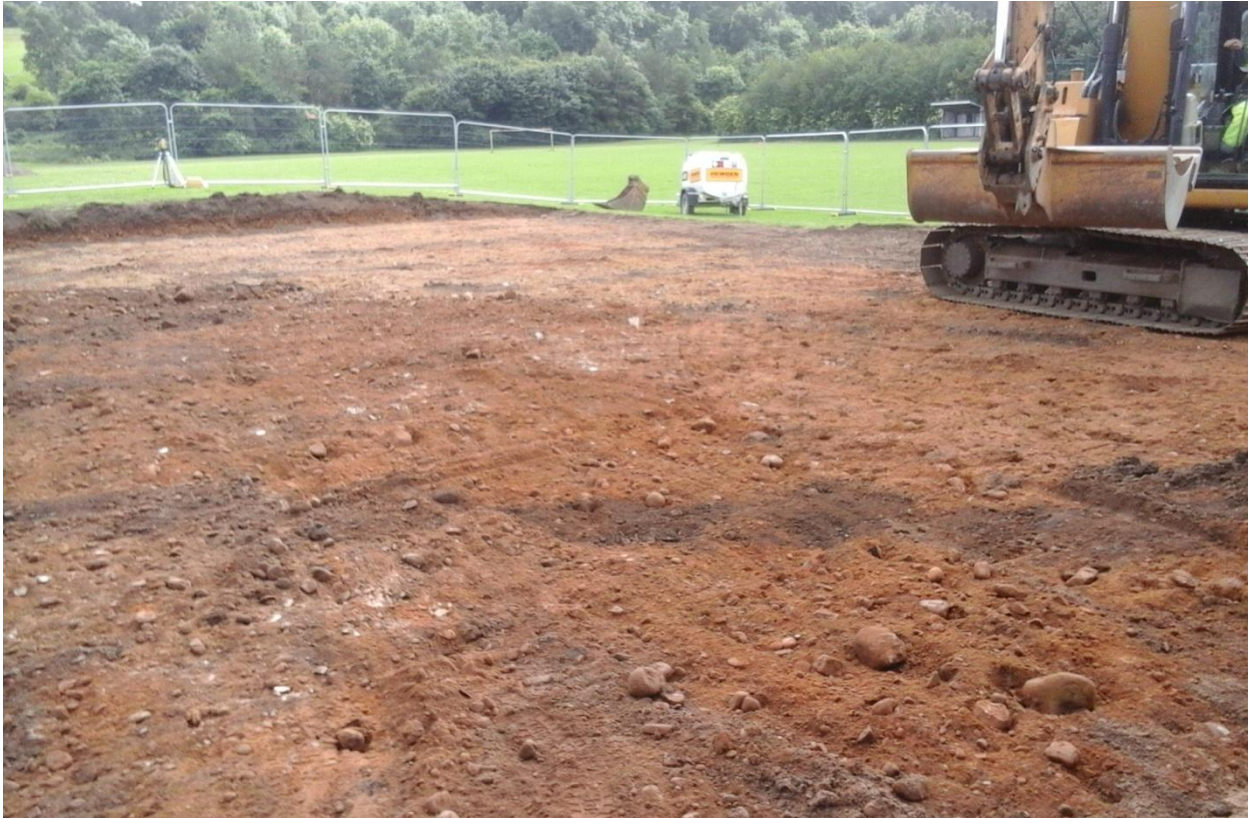
Plate 3: Stripping completed for pavilion extension (from north east)
