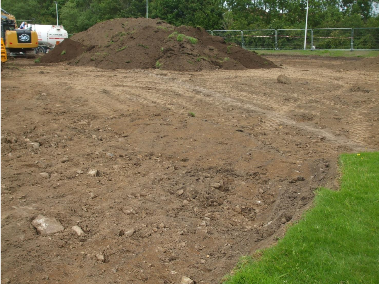
Plate 1: Stripping complete in car park area
