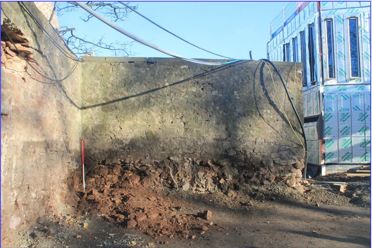
Plate 3: General view of the later added building from the south-west
