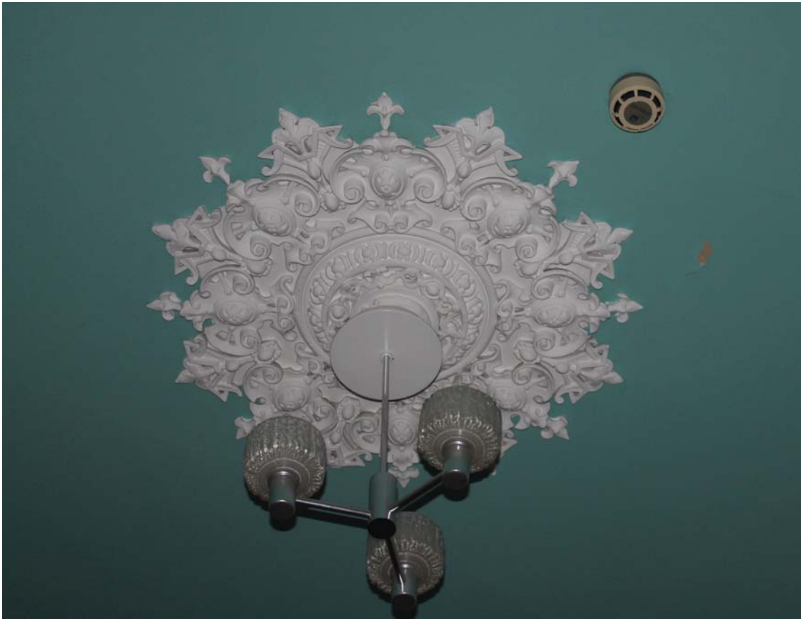
Plate 43: Room 0/1, detail of ceiling rose
