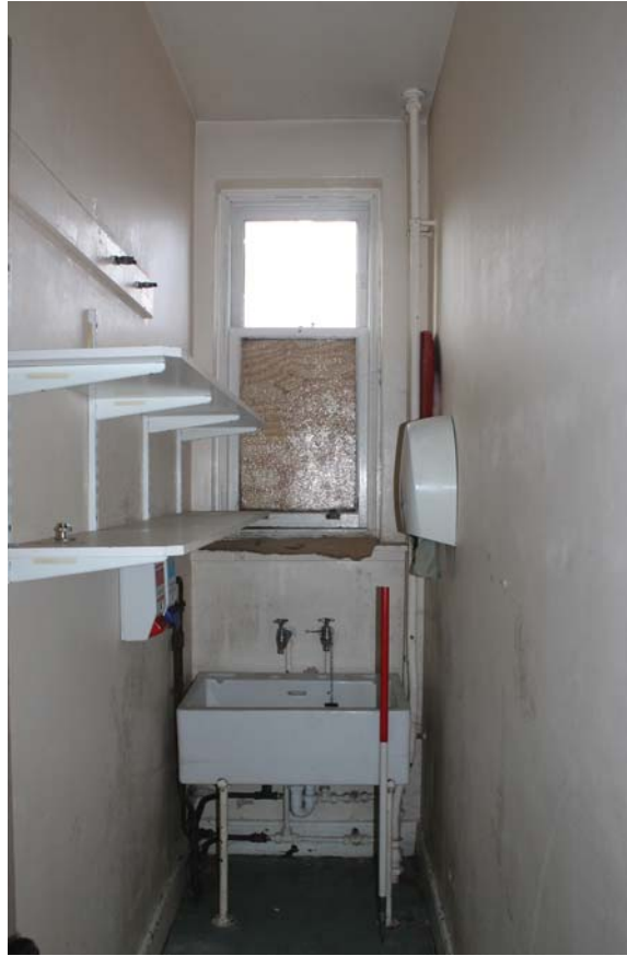
Plate 171: Room 0/30, general view from the east
