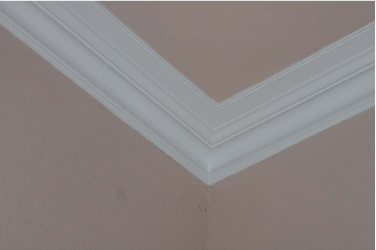
Plate 87: Room 1/3, detail of cornice
