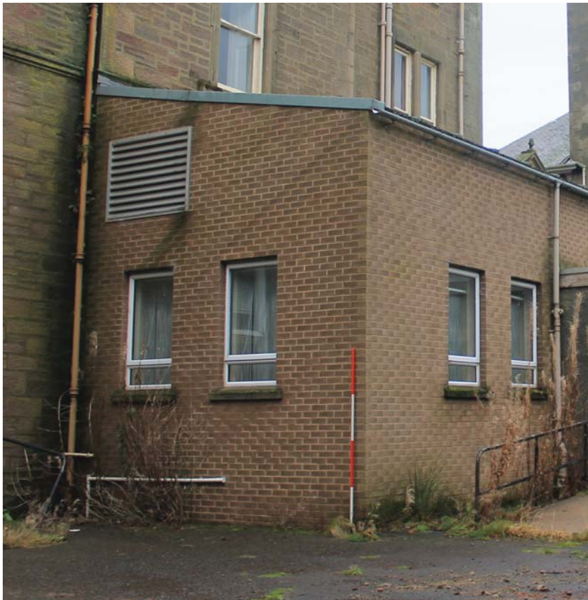
Plate 148: Building C, East Wing, general view of modern lean-to building from the south-east
