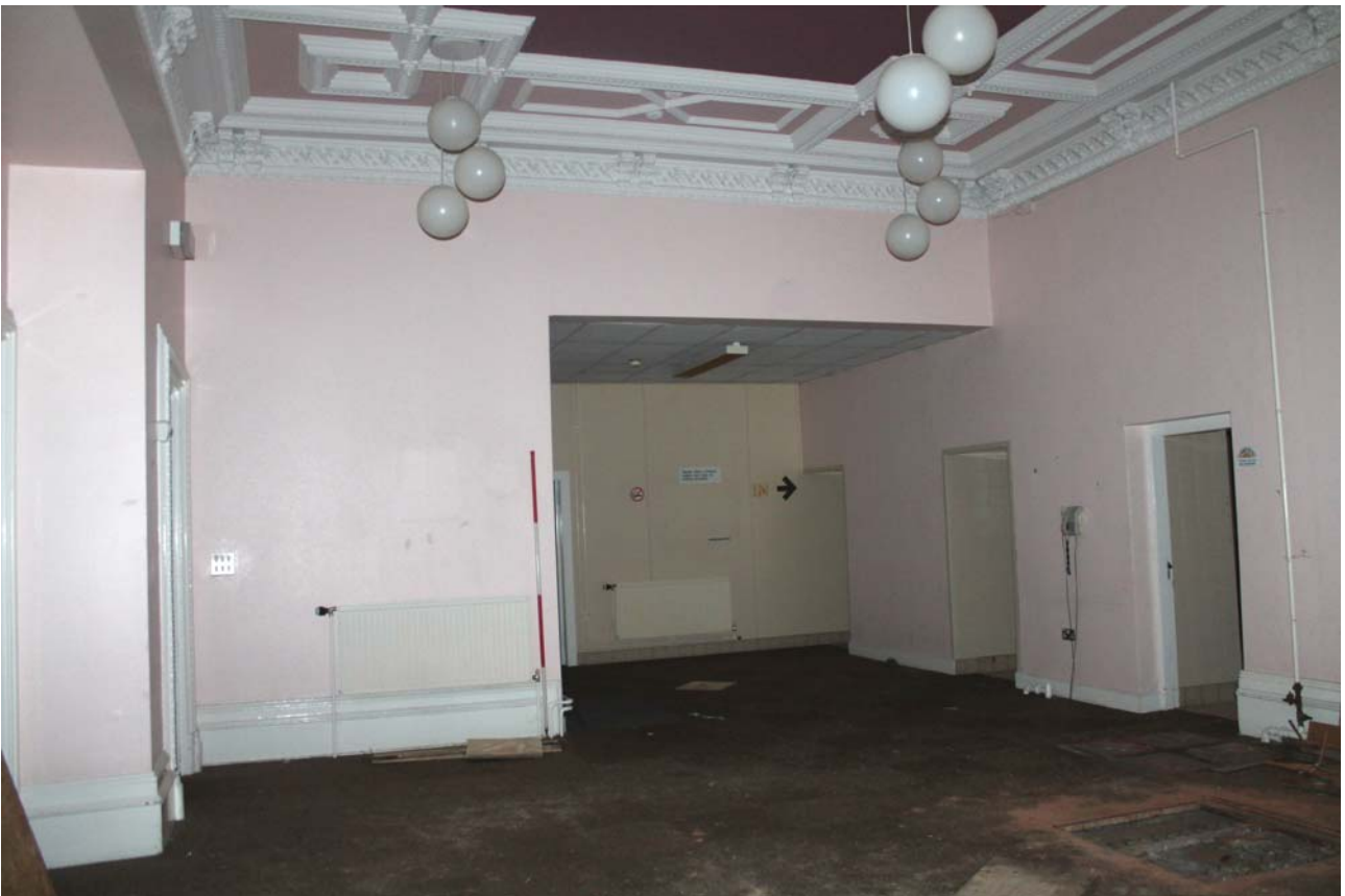
Plate 71: Room 0/7, general view from the SSW
