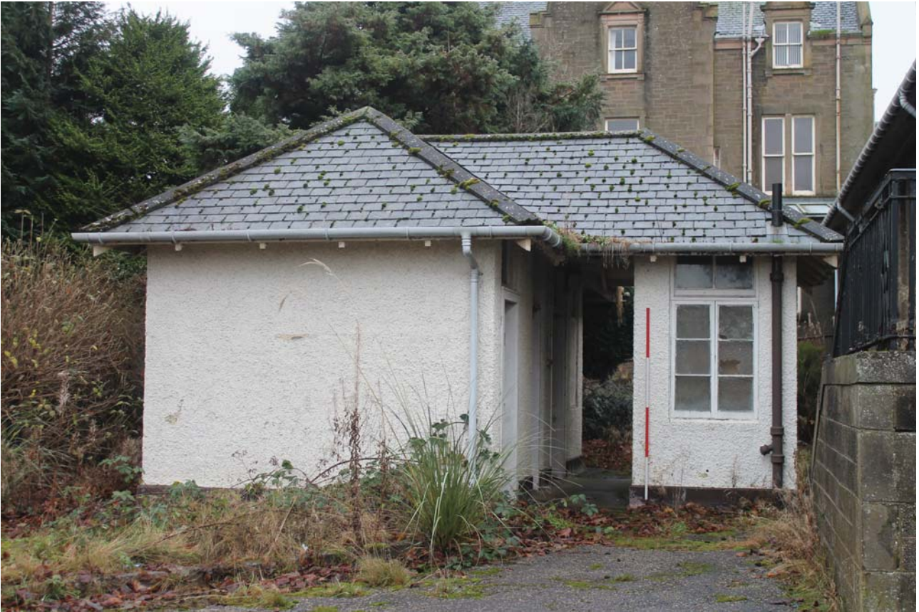
Plate 177: Building E, Toilet Block, general view from the east
