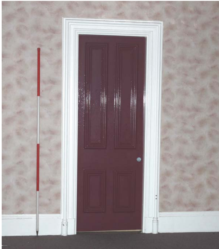
Plate 95: Room 1/7, detail of door in the west wall from the east
