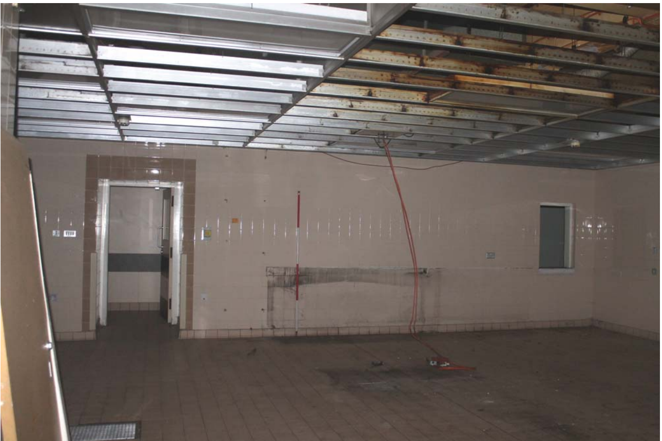
Plate 132: Room 0/11, general view from the north
