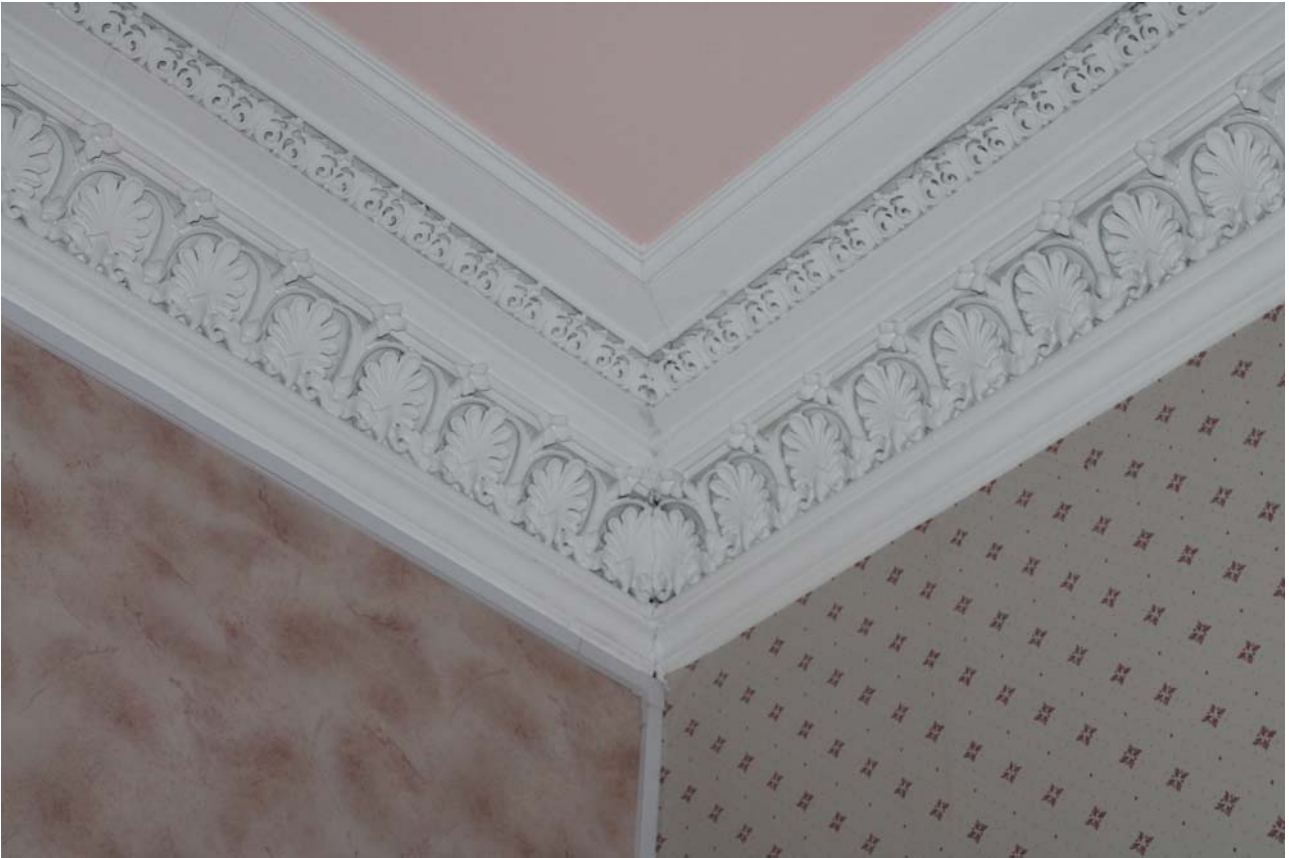
Plate 97: Room 1/7, detail of cornice
