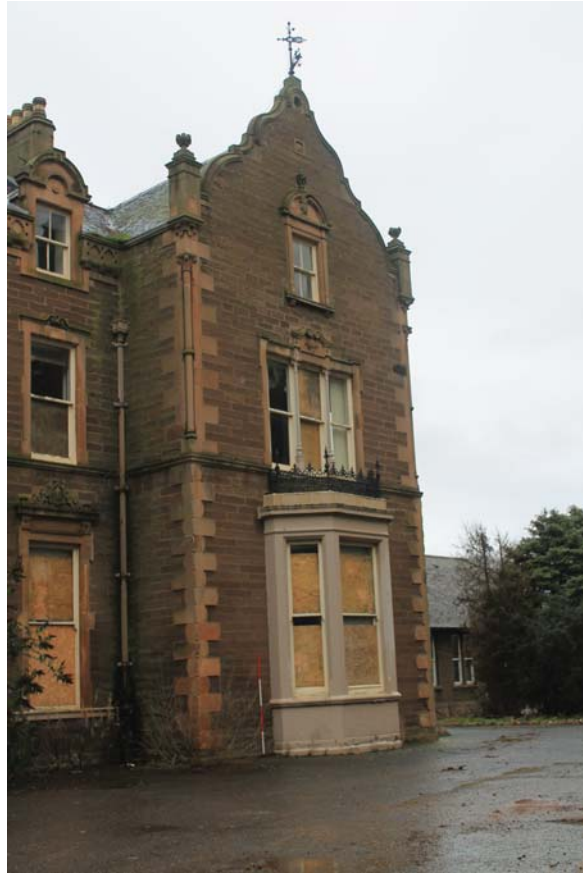
Plate 15: Ashludie House, South Elevation, general view of the eastern gable from the south-west
