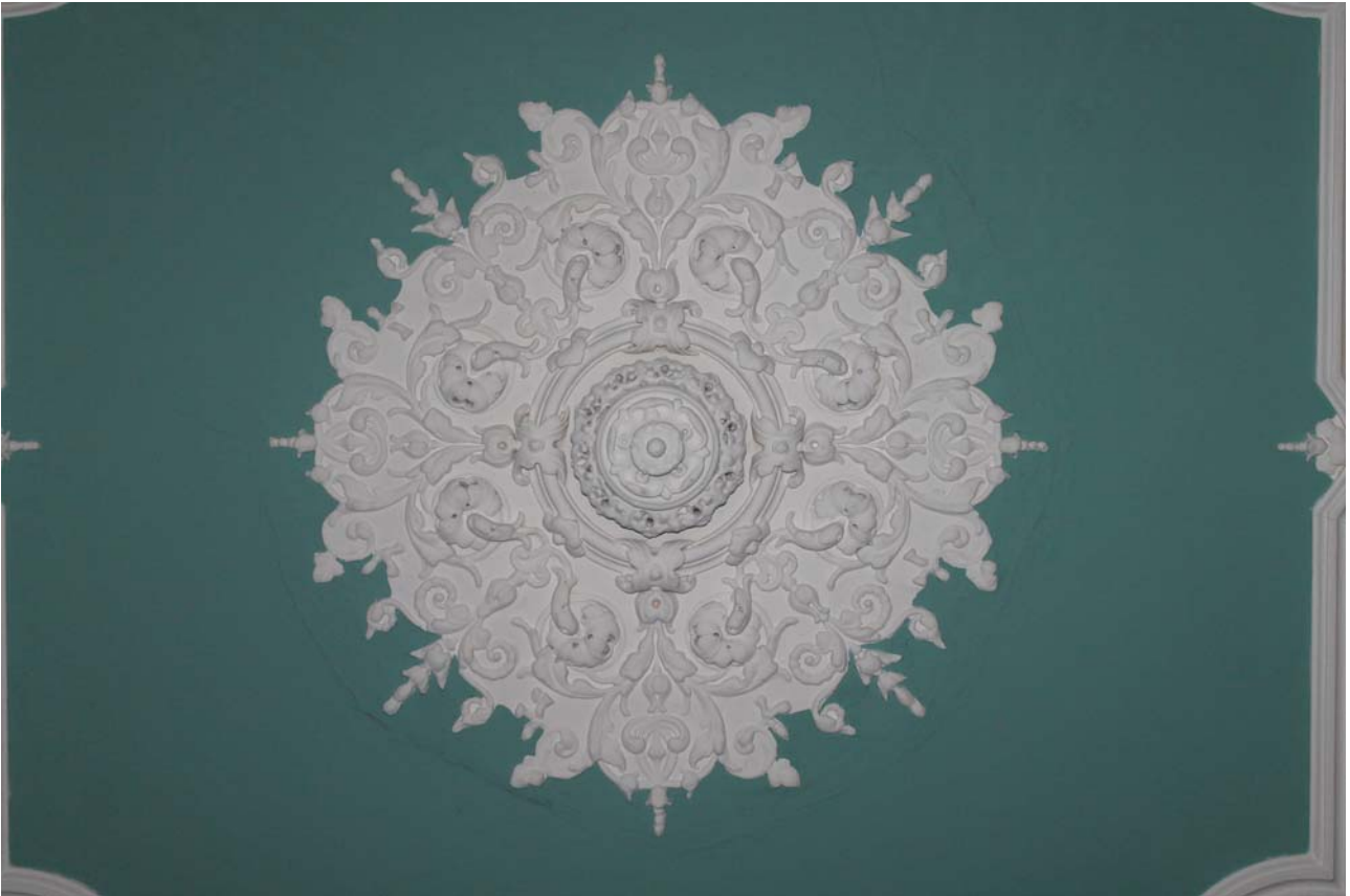
Plate 67: Room 0/6, detail of ceiling rose
