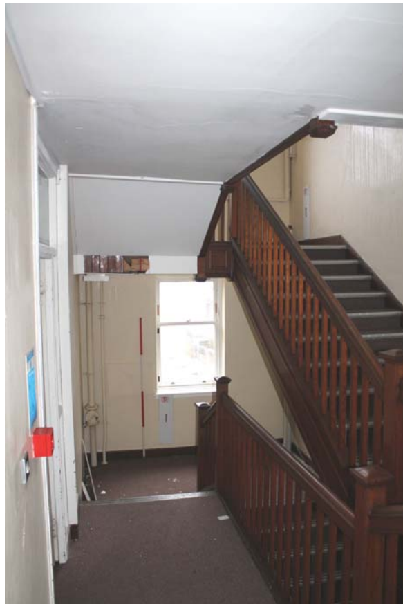
Plate 172: Room 1/20, general view from the NWW
