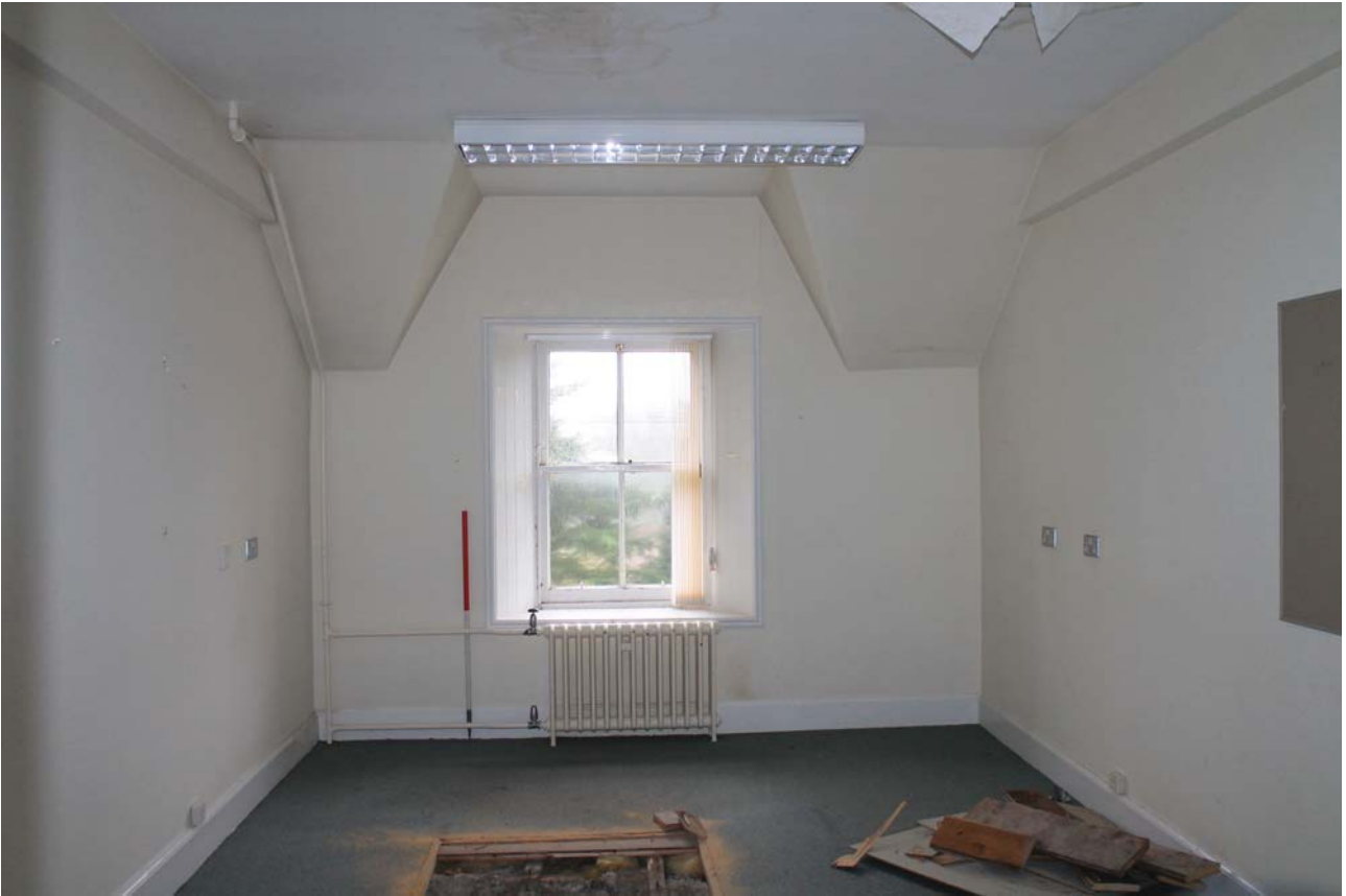
Plate 119: Room 2/13, general view from the north
