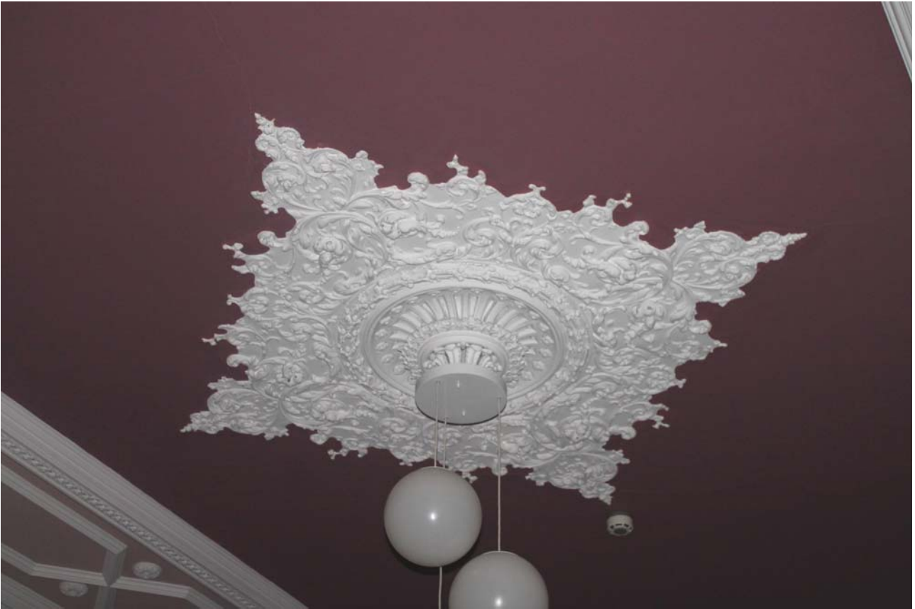
Plate 75: Room 0/7, detail of ceiling rose
