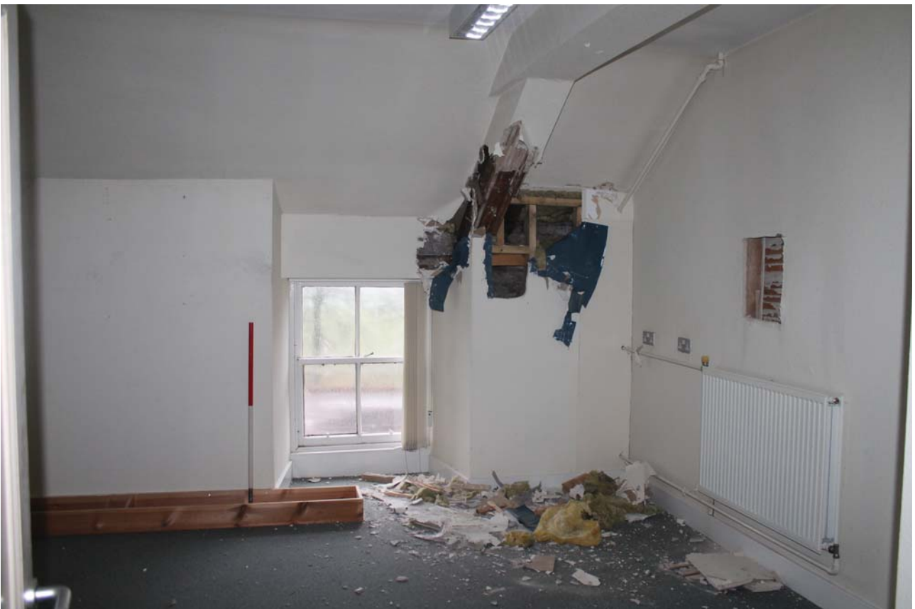
Plate 112: Room 2/5, general view from the south
