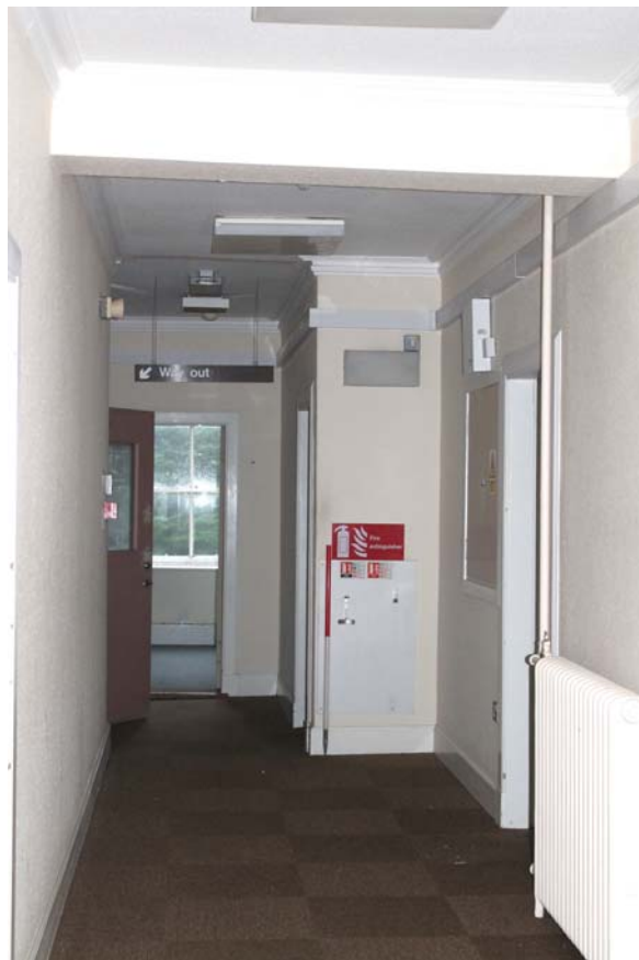
Plate 104: Room 2/1, general view from the east
