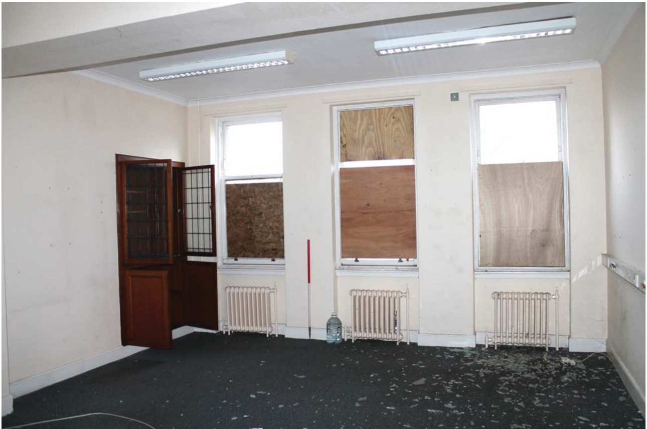
Plate 168: Room 0/24, general view from the SWW
