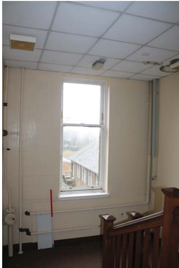
Plate 173: Room 2/15, general view from the NWW
