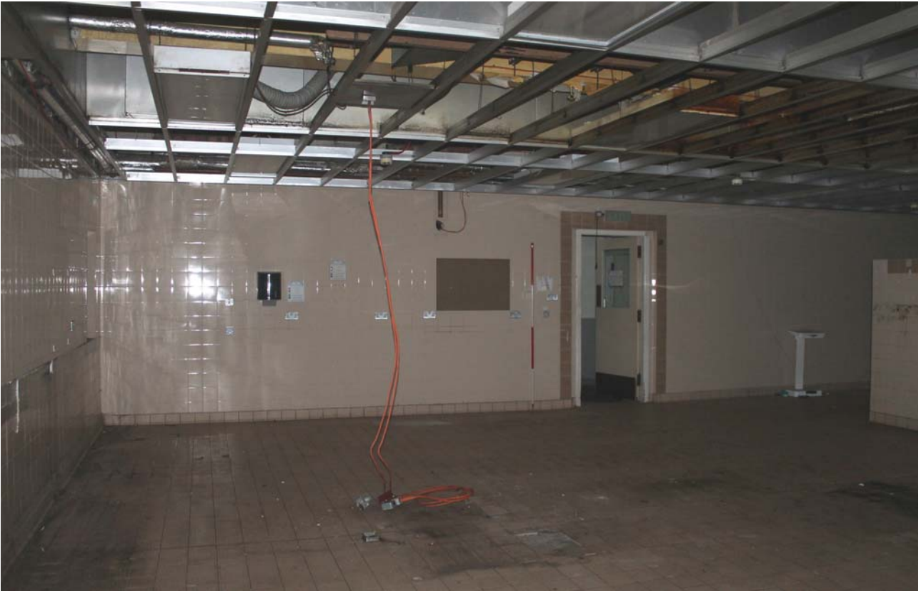
Plate 133: Room 0/11, general view from the east
