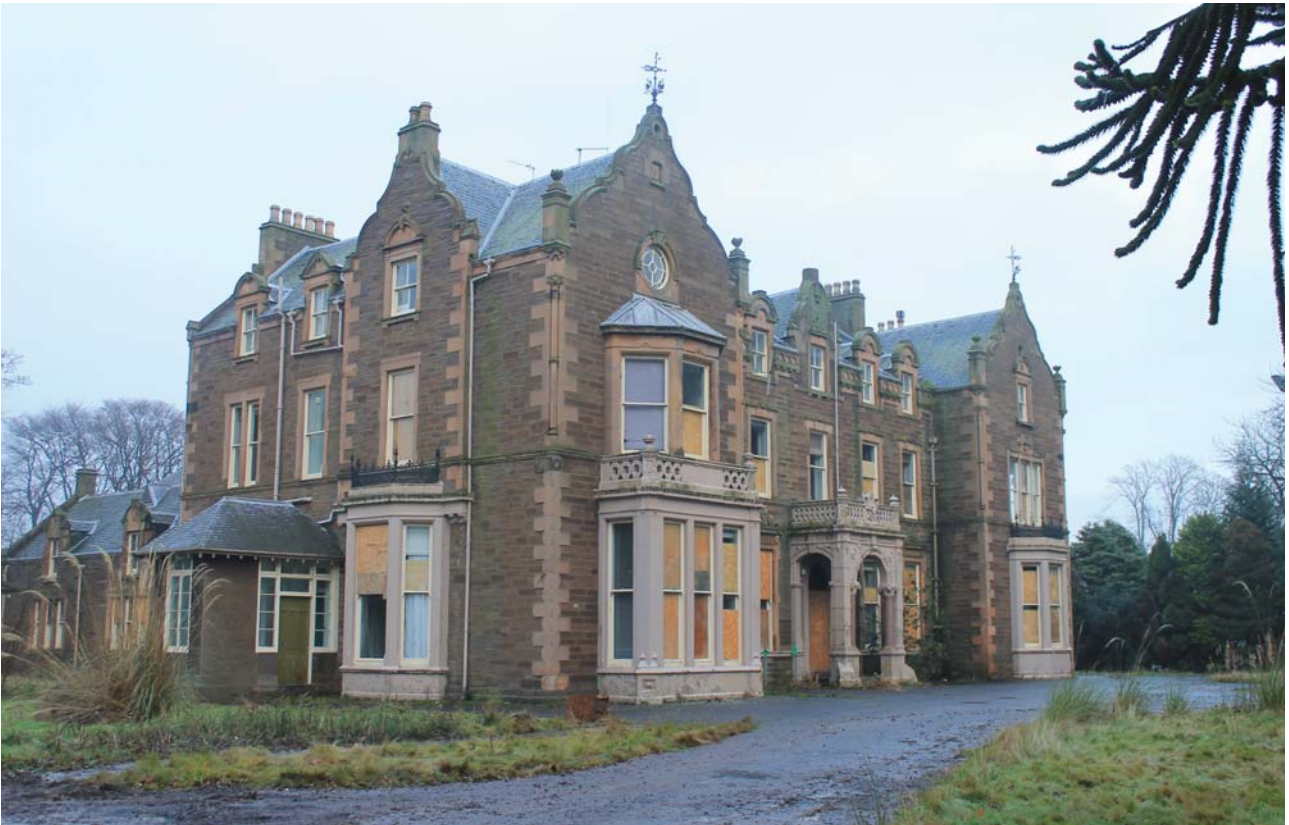
Plate 1: General view from the south-west
