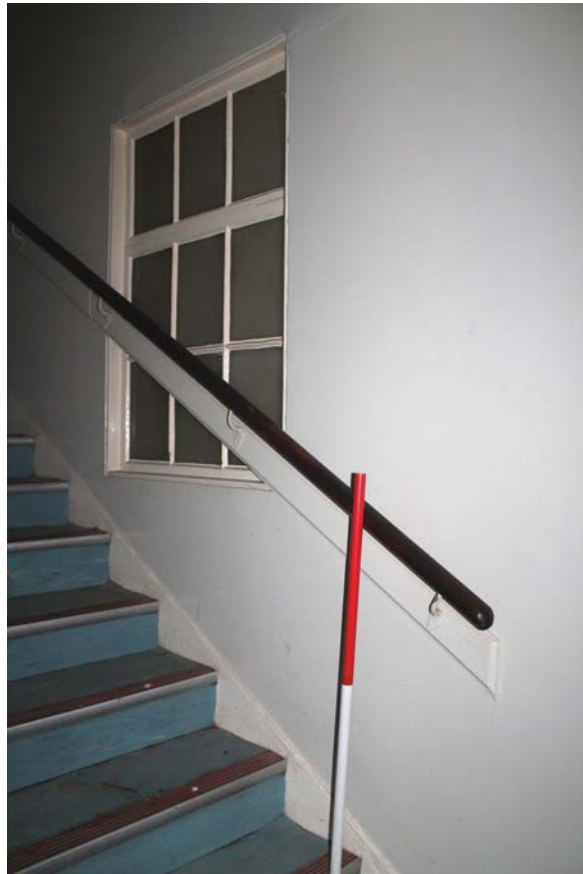
Plate 83: Room 0/10b, detail of blocked-off stair from the SSW
