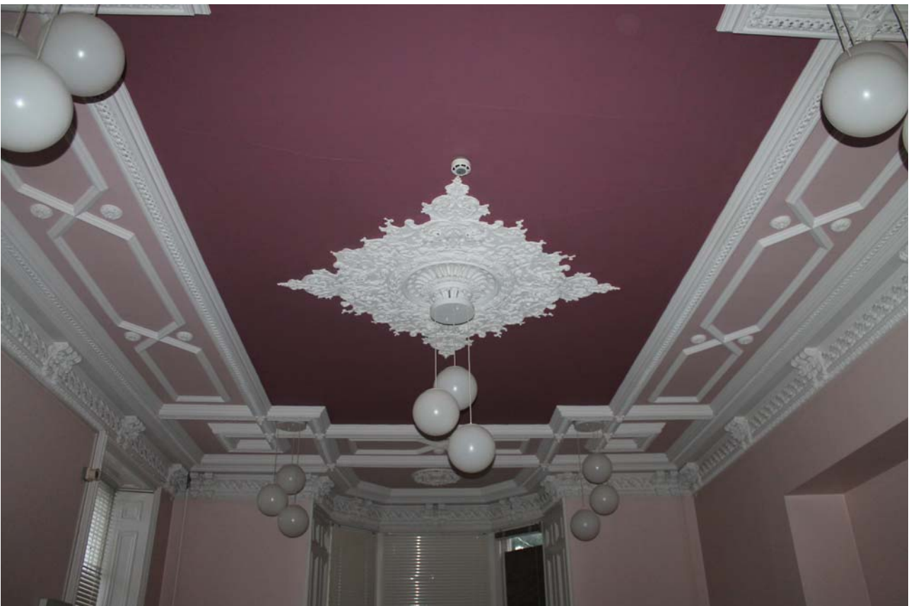
Plate 72: Room 0/7, detail of ceiling from the north
