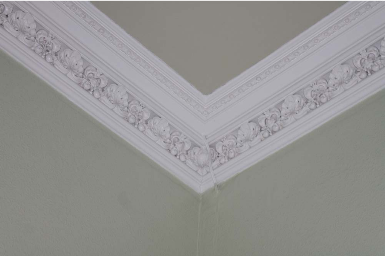
Plate 55: Room 0/5, detail of cornice
