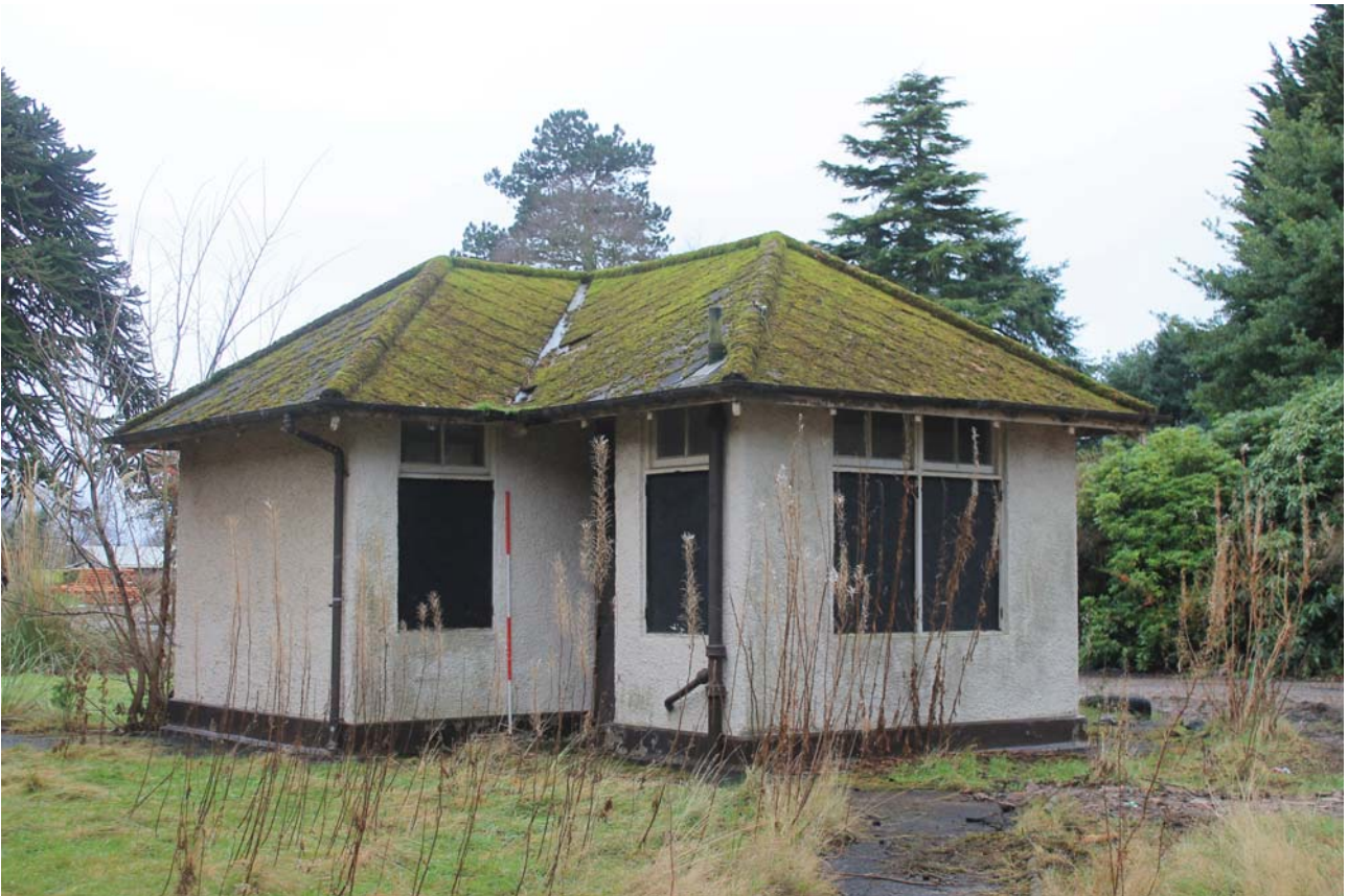
Plate 178: Building F, Toilet Block, general view from the north-east
