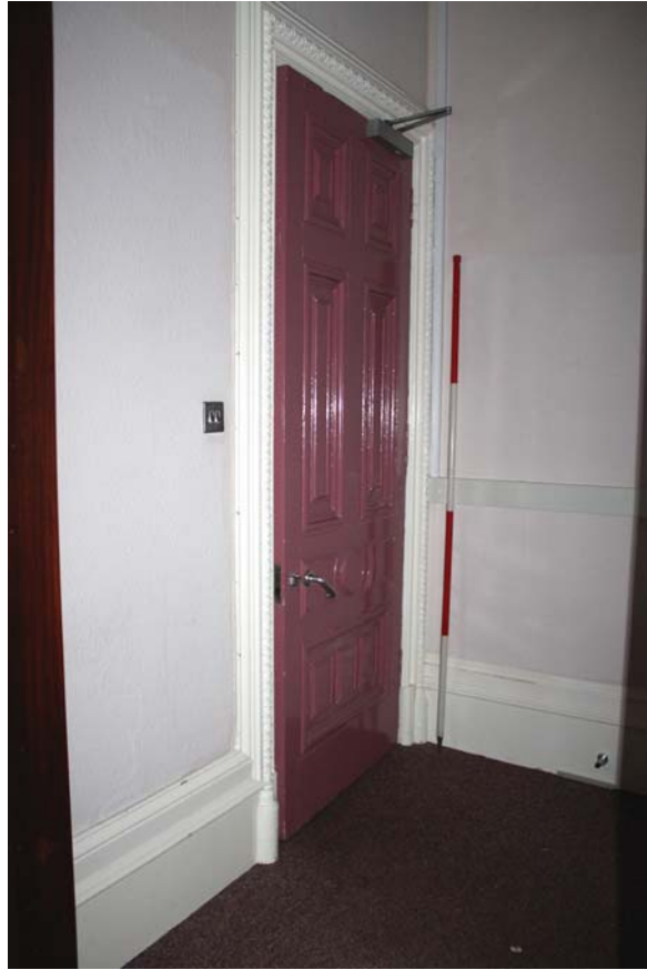
Plate 79: Room 0/8, detail of door in the east wall from the north-west
