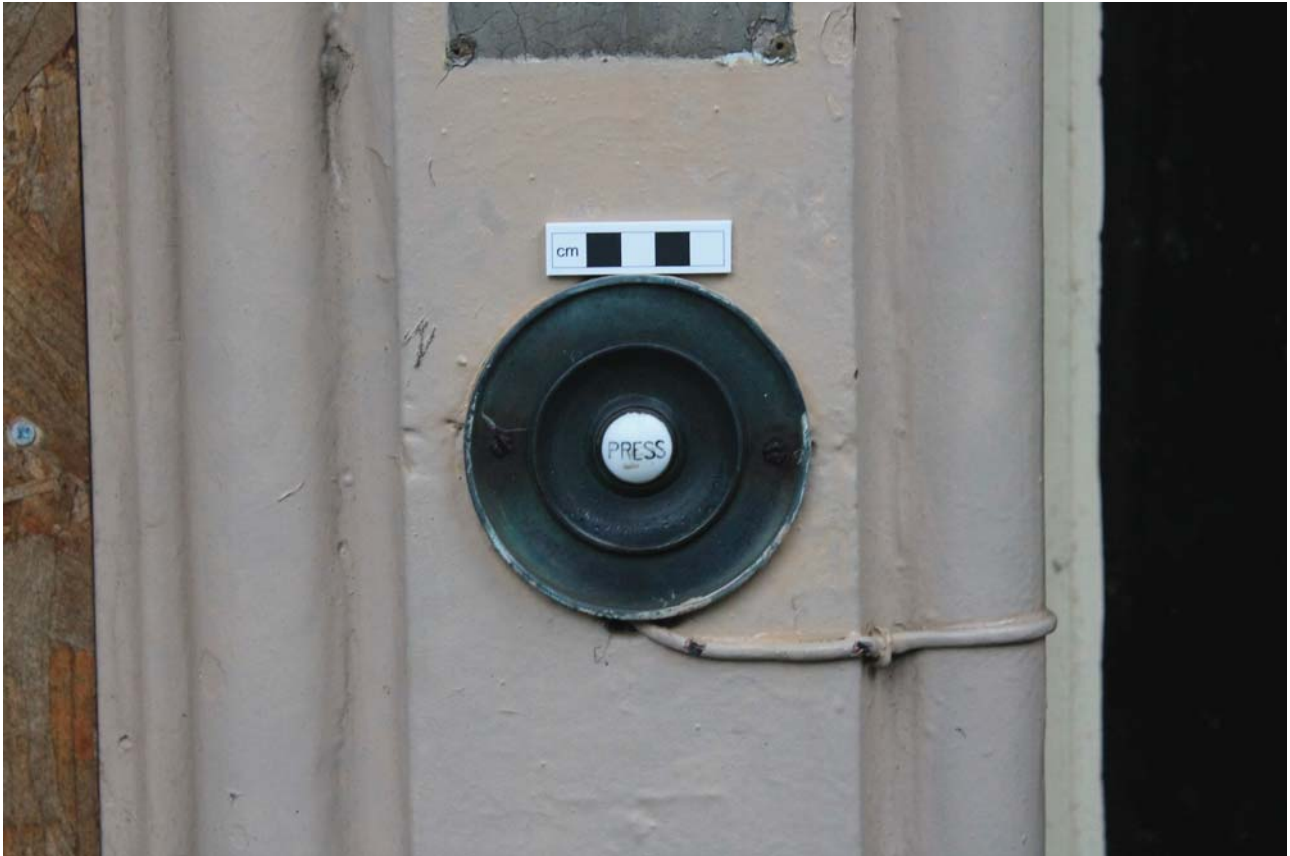
Plate 13: Ashludie House, South Elevation, detail of doorbell to the main entrance from the south
