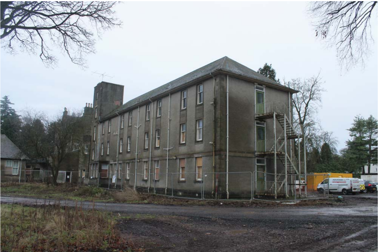
Plate 158: Building D, North Wing, general view from NNE
