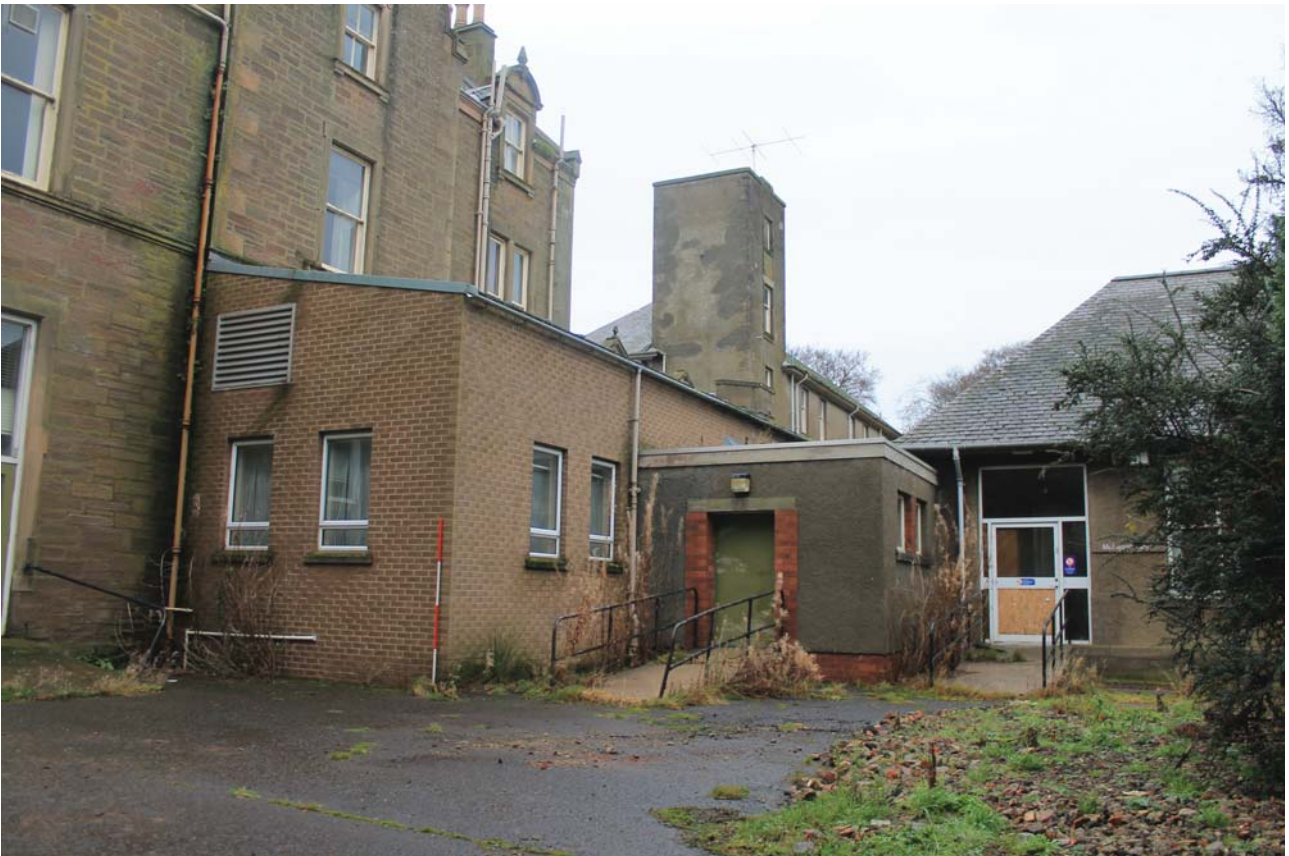
Plate 146: Building C, East Wing, South Elevation, general view of the westernmost bays showing the later brick build, from the south-east
