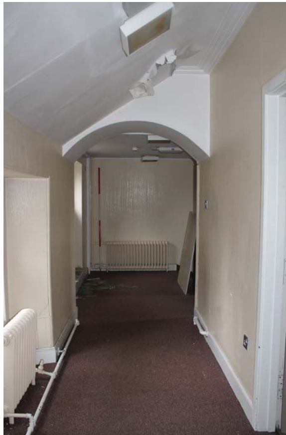
Plate 140: Room 1/19, general view from the south
