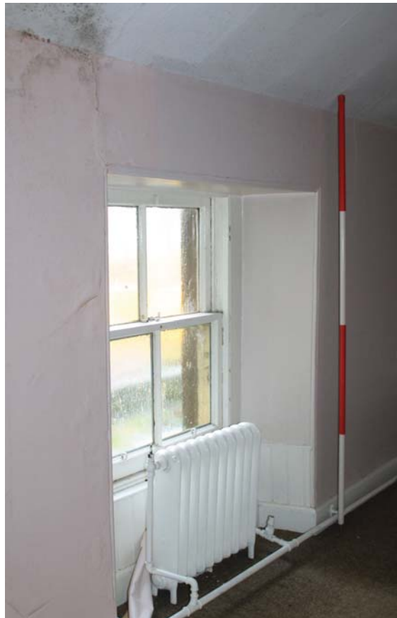
Plate 136: Room 1/15, detail of corridor window in the west wall from the south-east
