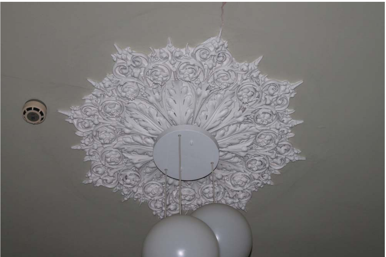
Plate 56: Room 0/5, detail of ceiling rose
