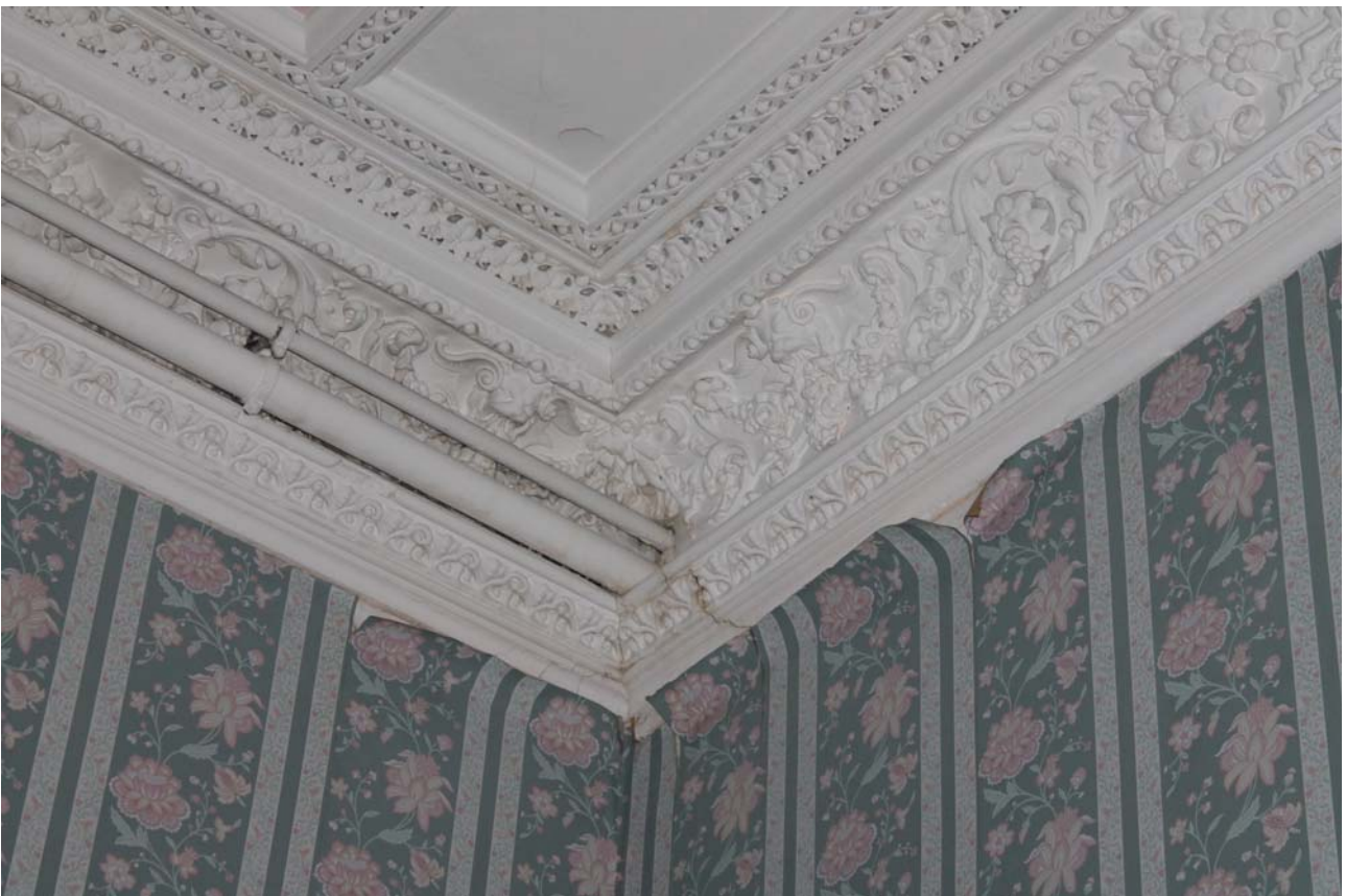
Plate 66: Room 0/6, detail of cornice
