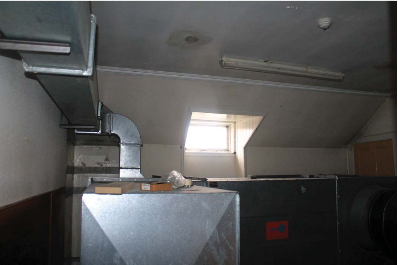
Plate 137: Room 1/16, general view from the NWW
