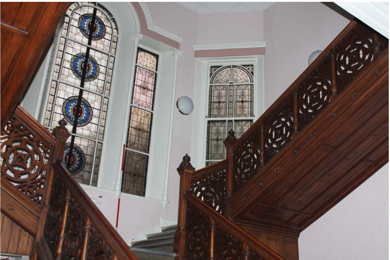
Plate 48: Room 0/2, general view of stained glass landing window in the north wall from the south-west
