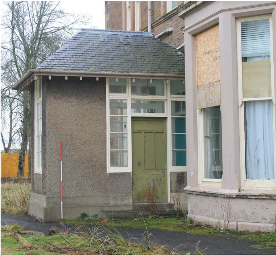
Plate 29: Ashludie House, West Elevation, detail of later porch from the SSW
