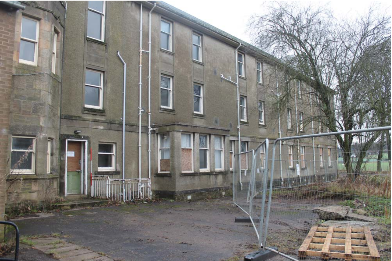
Plate 157: Building D, North Wing, East Elevation, general view from the south-east
