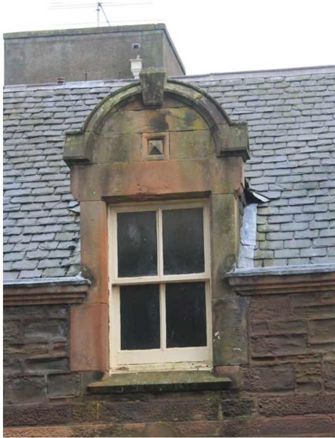
Plate 125: Building B1, West Elevation, detail of dormer window from the west
