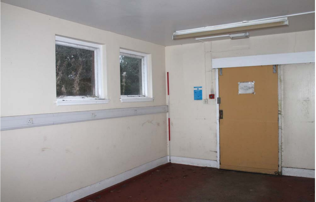
Plate 151: Room 0/16, general view from the north-west
