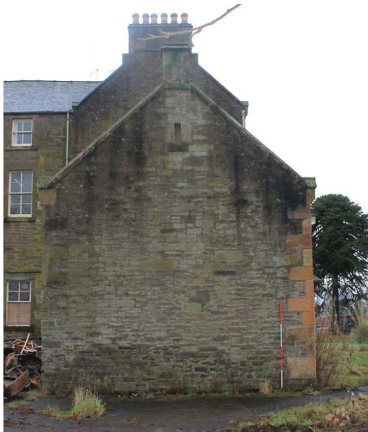
Plate 126: Building B1, North Elevation, general view from the north
