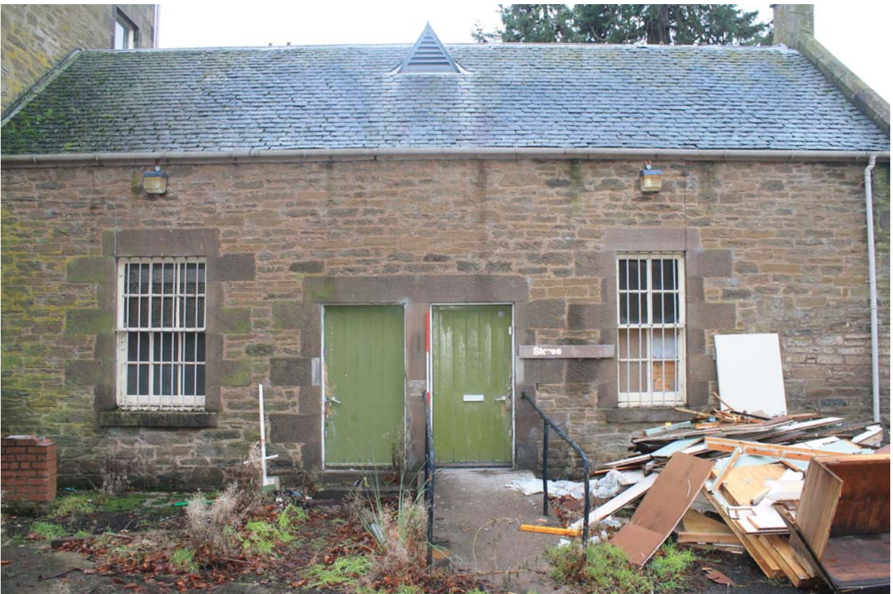
Plate 122: Building B1, East Elevation, general view from the east
