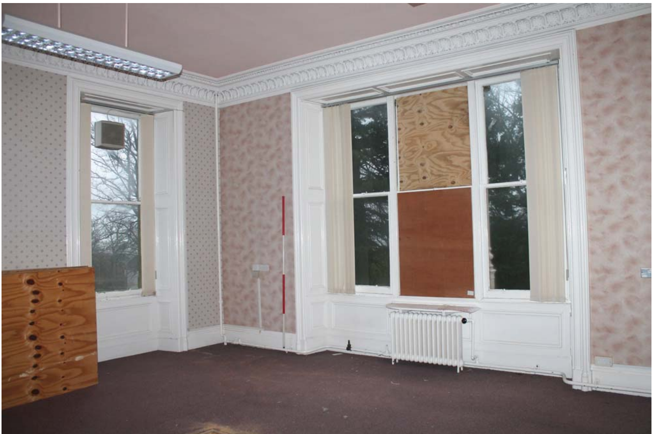
Plate 96: Room 1/7, general view from the north-west
