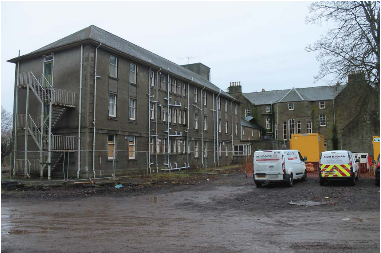
Plate 160: Building D, North Wing, general view from the north-west
