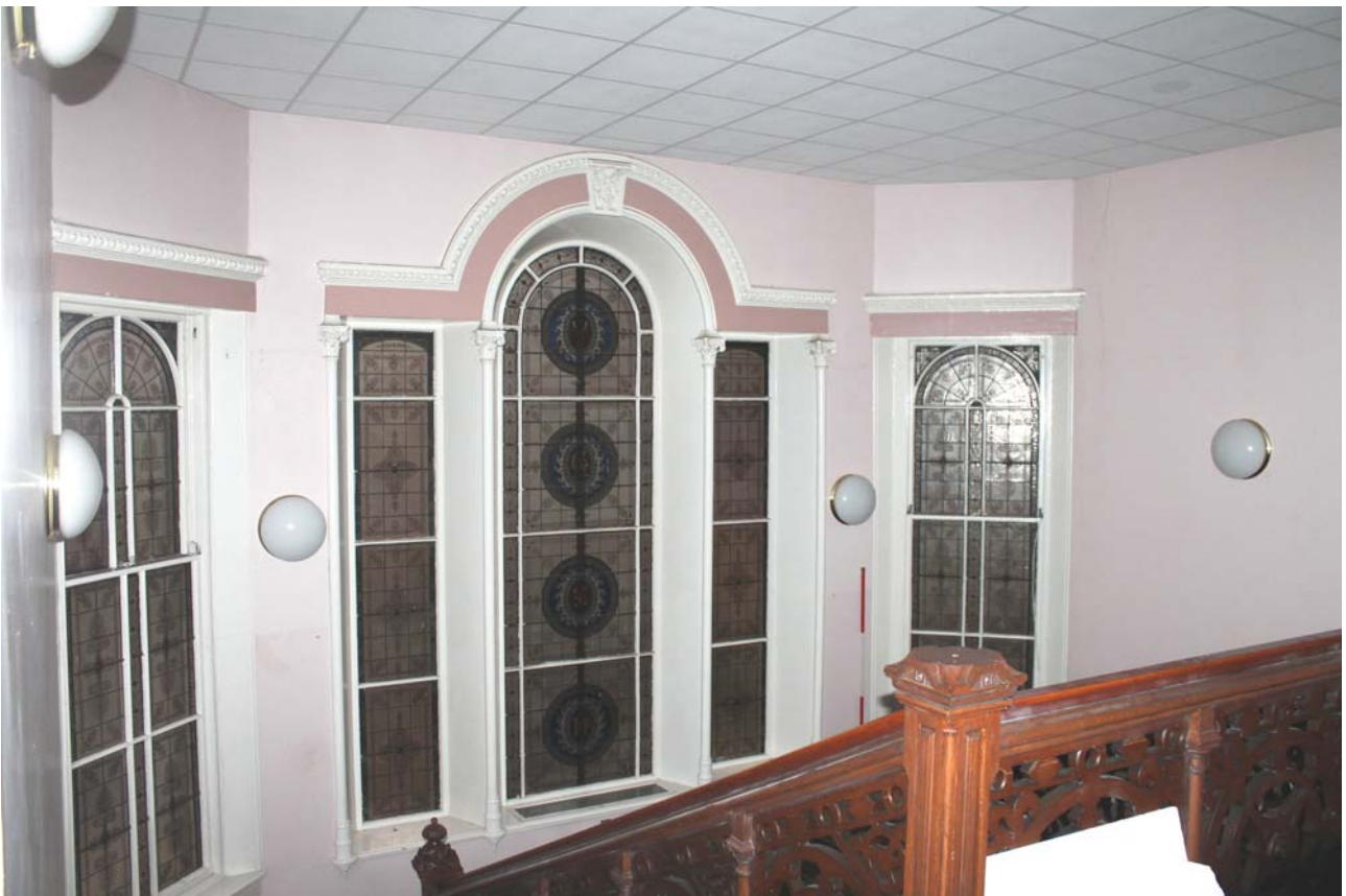
Plate 50: Room 0/2, general view of stained glass landing window in the north wall, taken from the first floor landing, from the south-west
