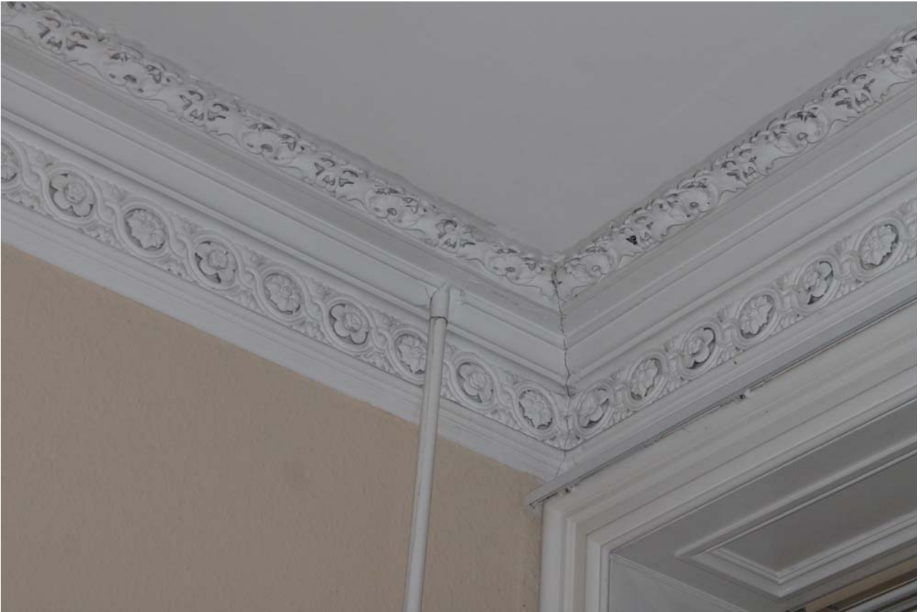
Plate 99: Room 1/8, detail of cornice
