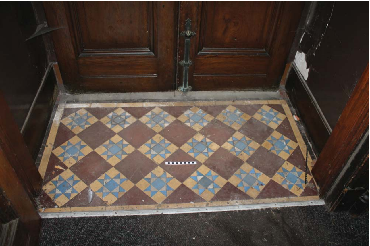
Plate 38: Room 0/1, detail of encaustic floor tiles in small porch from the north
