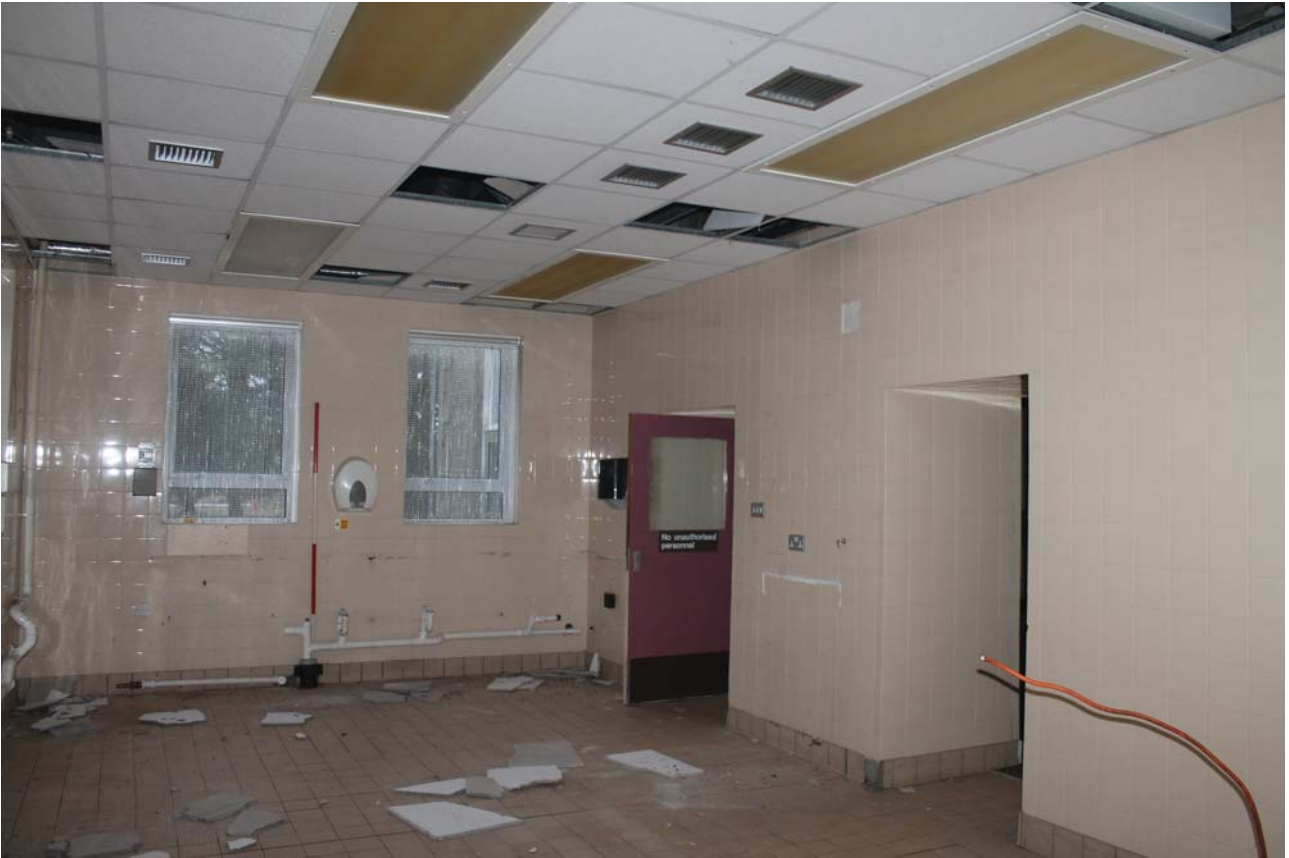
Plate 149: Room 0/12, general view from the north-east
