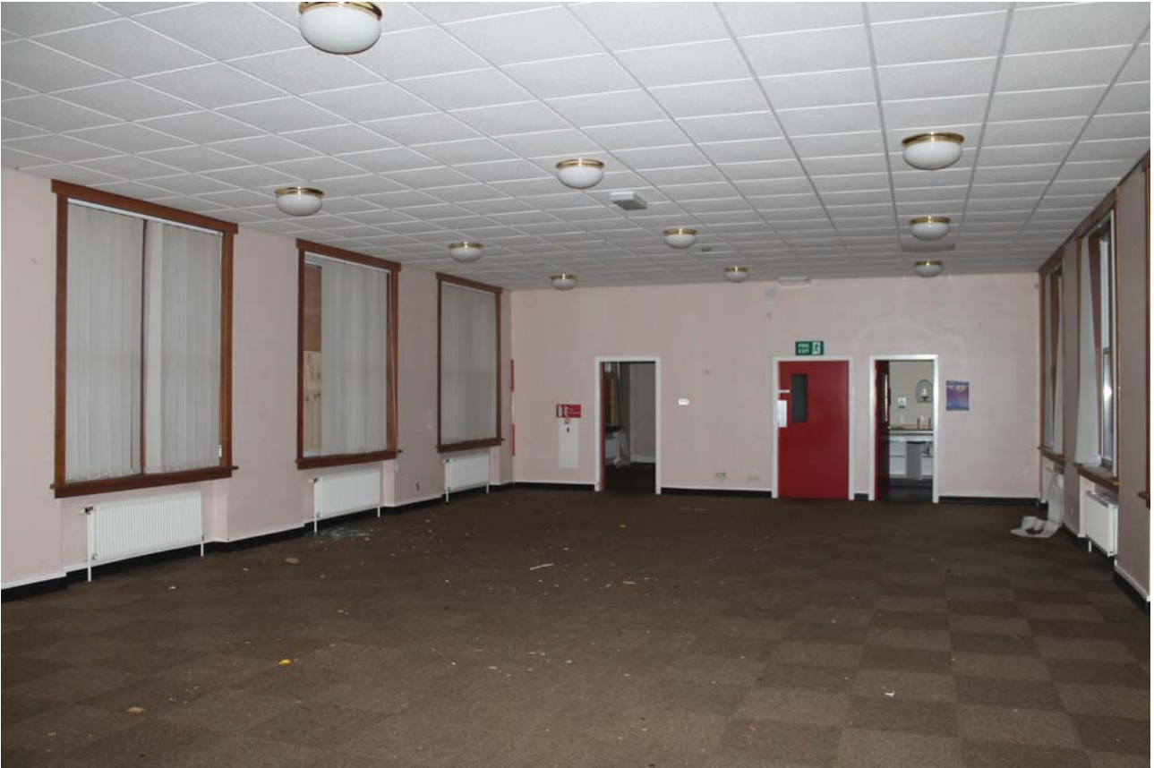
Plate 153: Room 0/17, general view from the SWW
