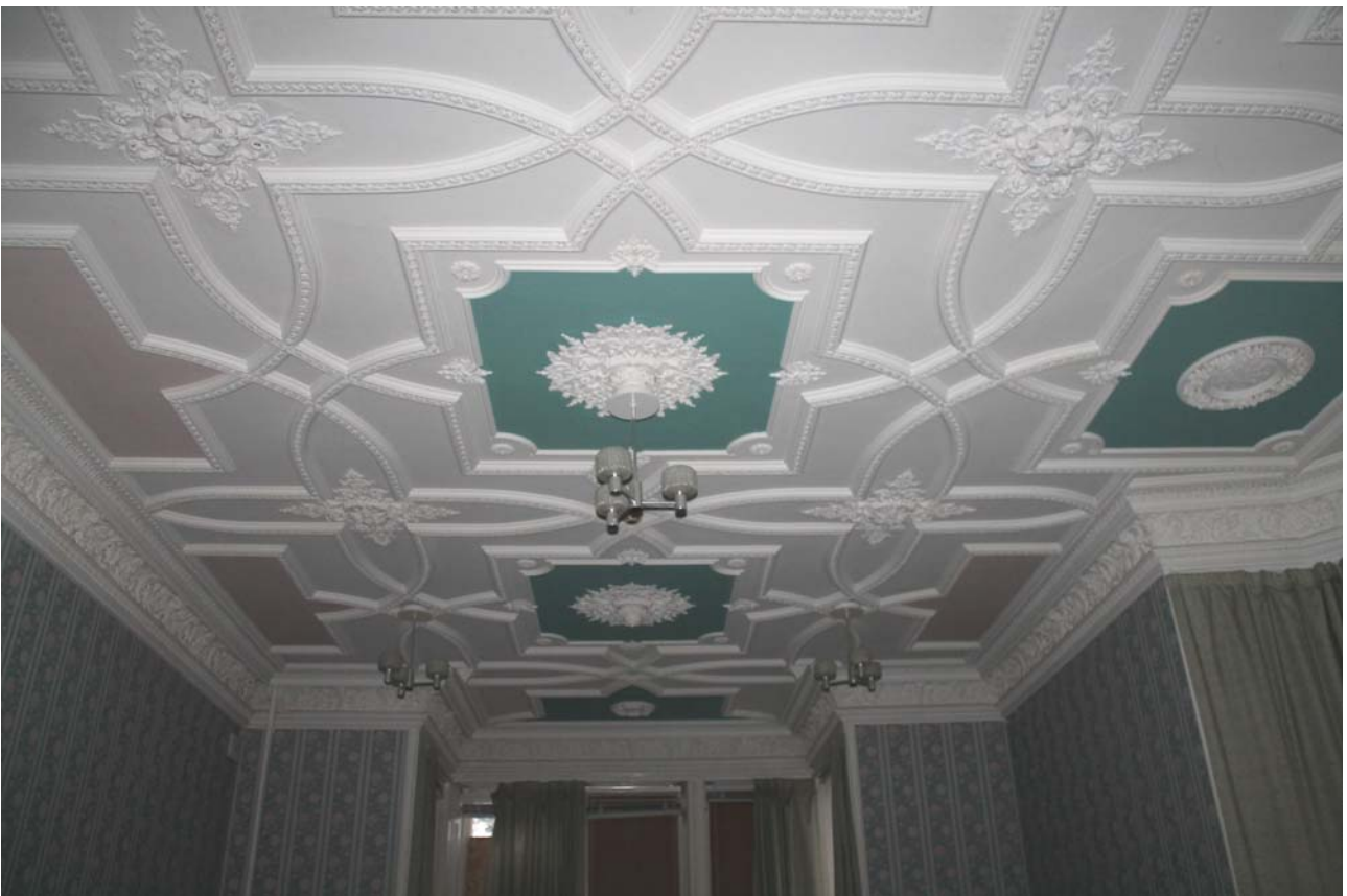
Plate 60: Room 0/6, general view of the ceiling from the north
