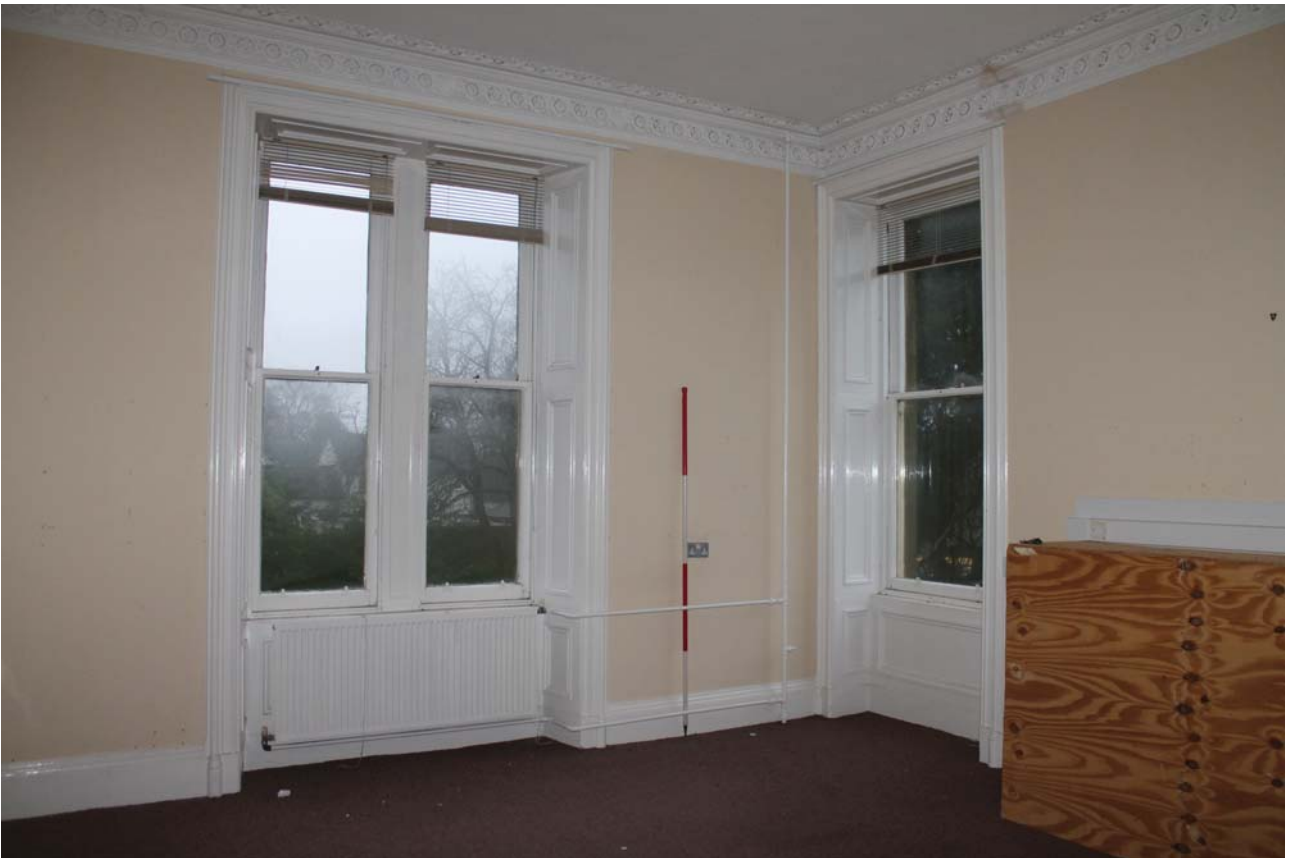
Plate 98: Room 1/8, general view from the south-east
