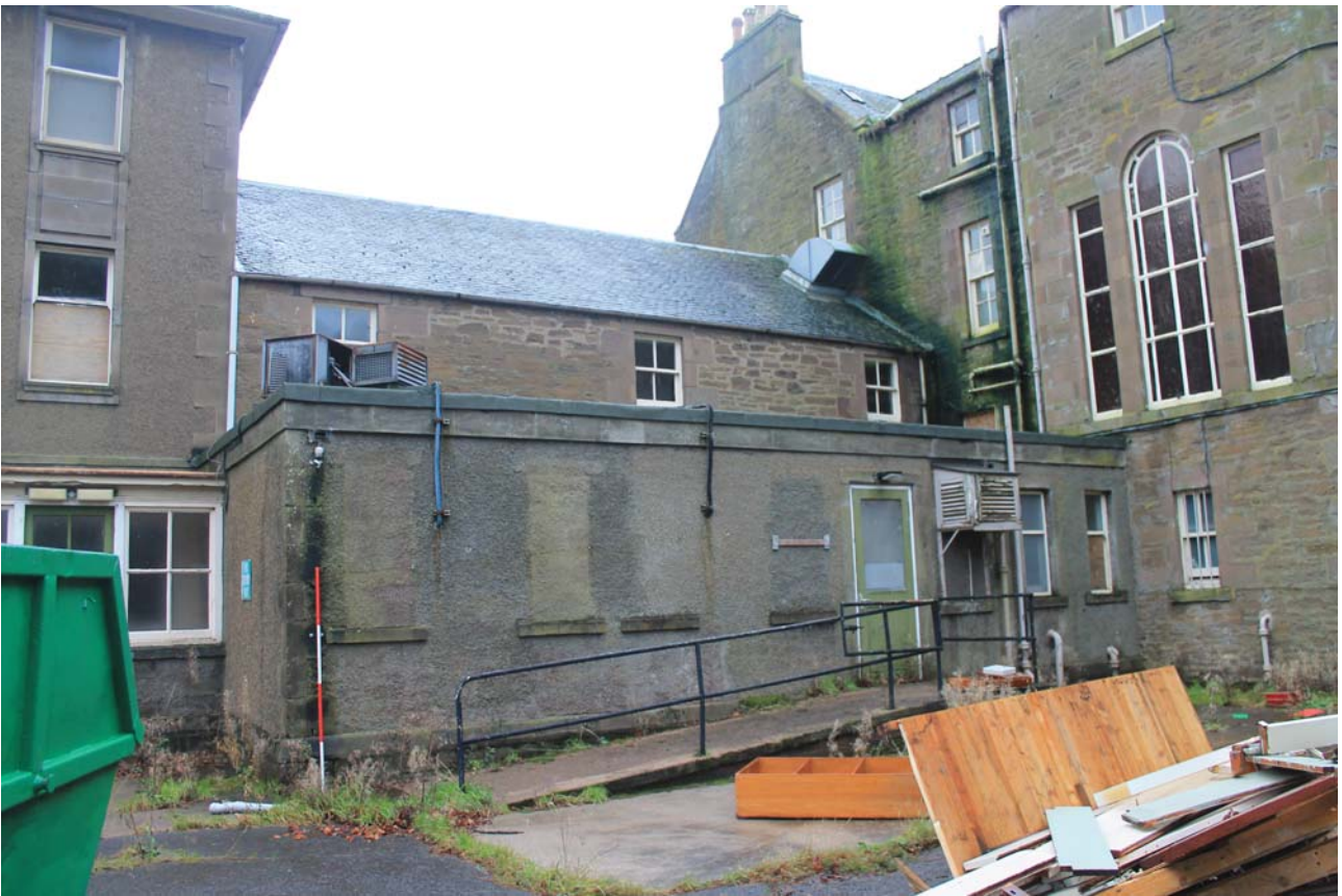
Plate 131: Building B2, West Elevation, general view from the NWW
