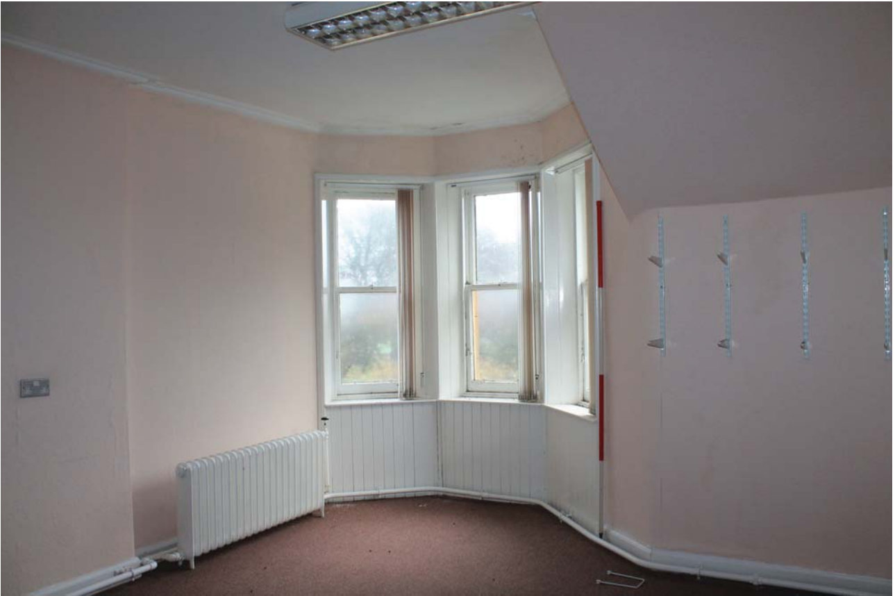
Plate 139: Room 1/18a, general view showing the bay window in the east wall from the SWW
