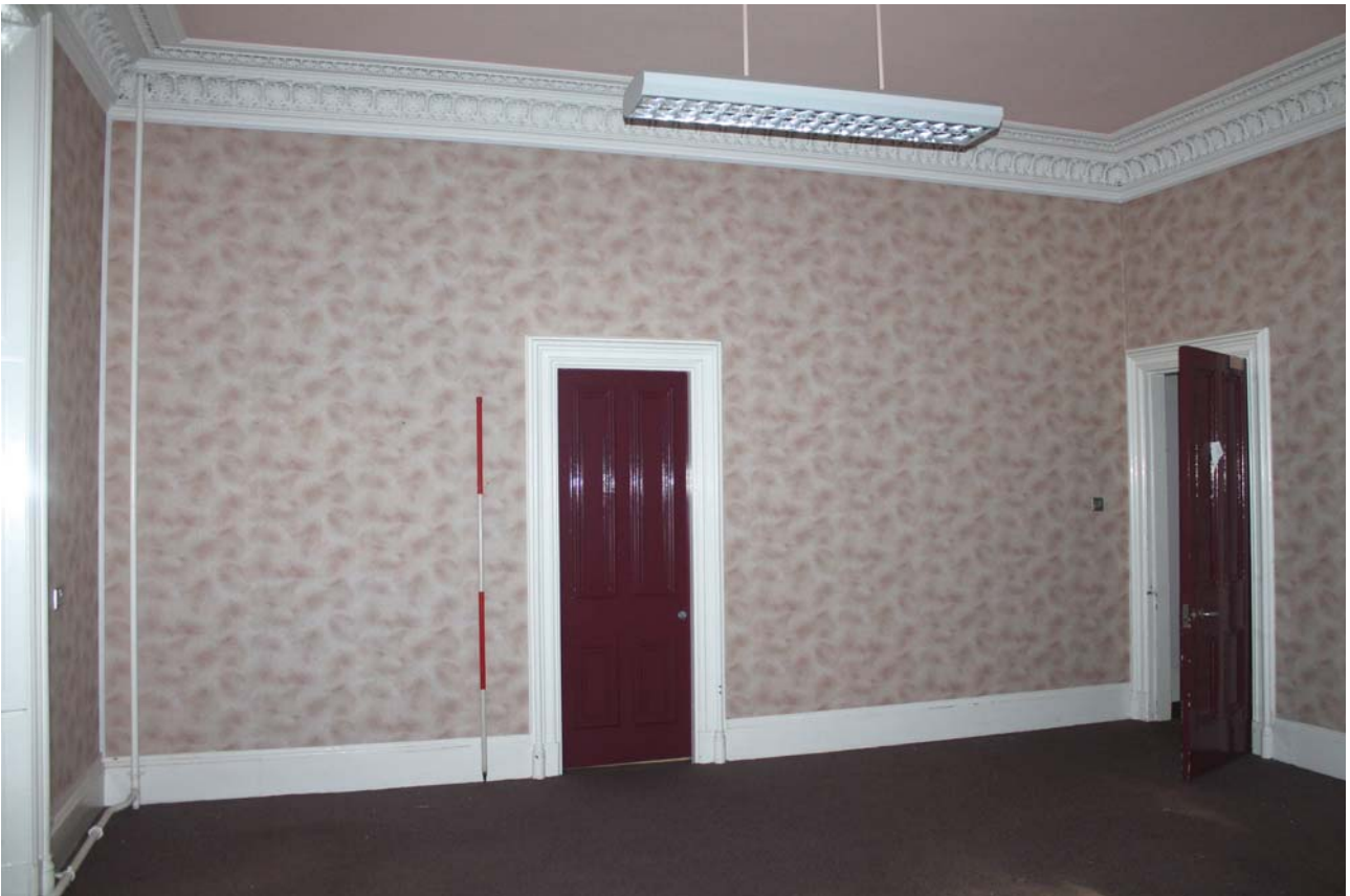
Plate 94: Room 1/7, general view of the west wall from the SEE
