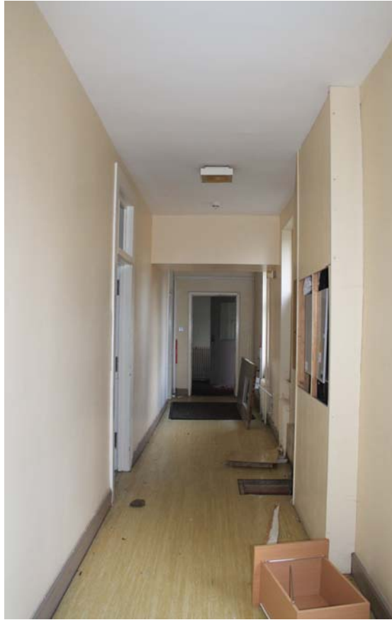
Plate 167: Room 0/22, general view from the south
