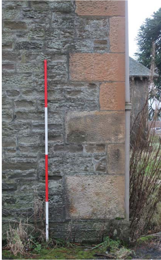
Plate 127: Building B1, North Elevation, detail of quoins from the north
