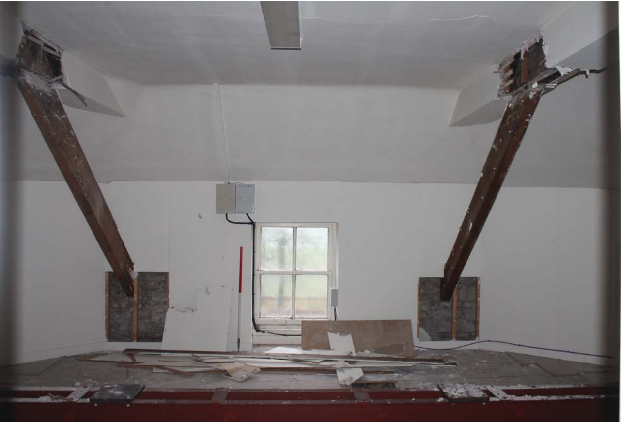
Plate 113: Room 2/6, general view from the south
