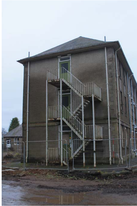
Plate 159: Building D, North Wing, North Elevation, general view from the NNW
