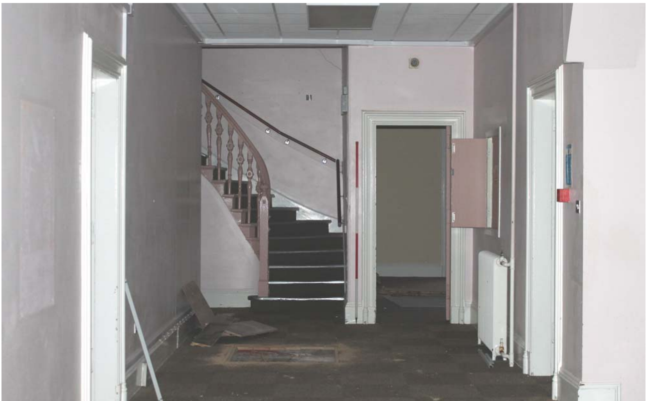
Plate 84: Room 1/1, general view from the east
