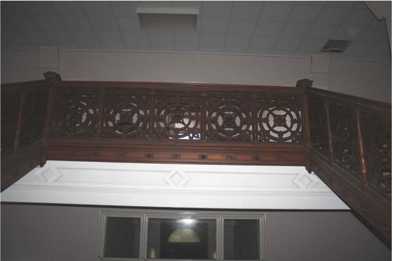
Plate 85: Room 1/1, detail of landing balustrade from the north
