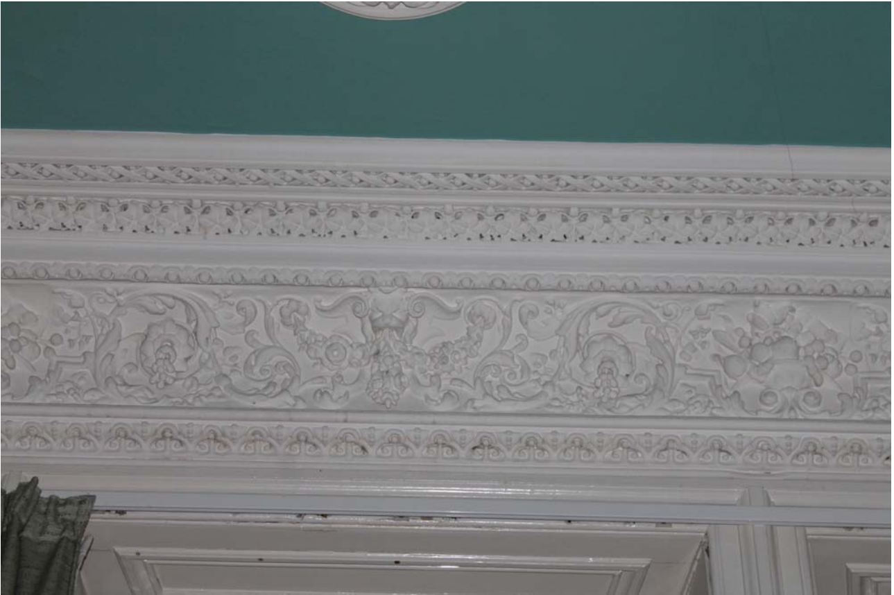
Plate 65: Room 0/6, detail of cornice
