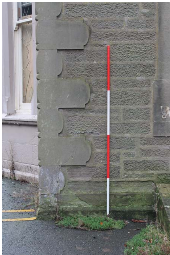
Plate 34: Ashludie House, East Elevation, detail of quoins to the south side from the east
