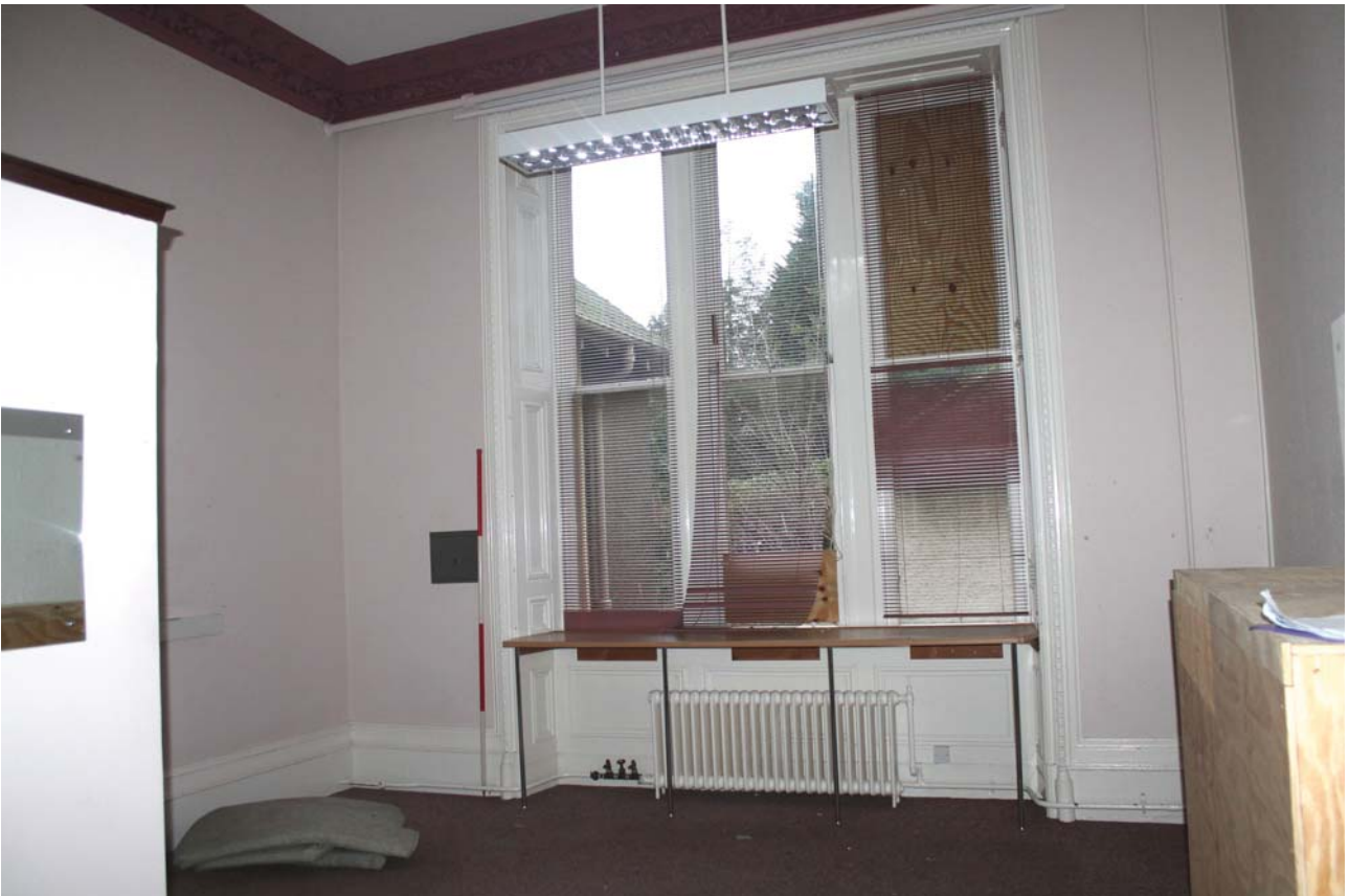
Plate 78: Room 0/8, general view from the north-east
