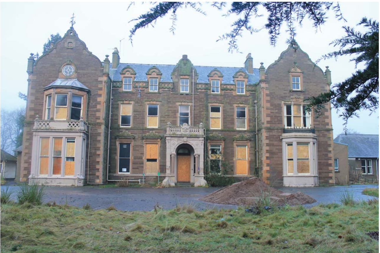
Plate 2: Ashludie House, South Elevation, general view from the south
