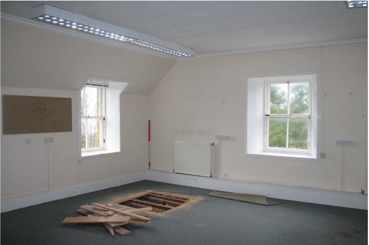
Plate 117: Room 2/11, general view from the north-west
