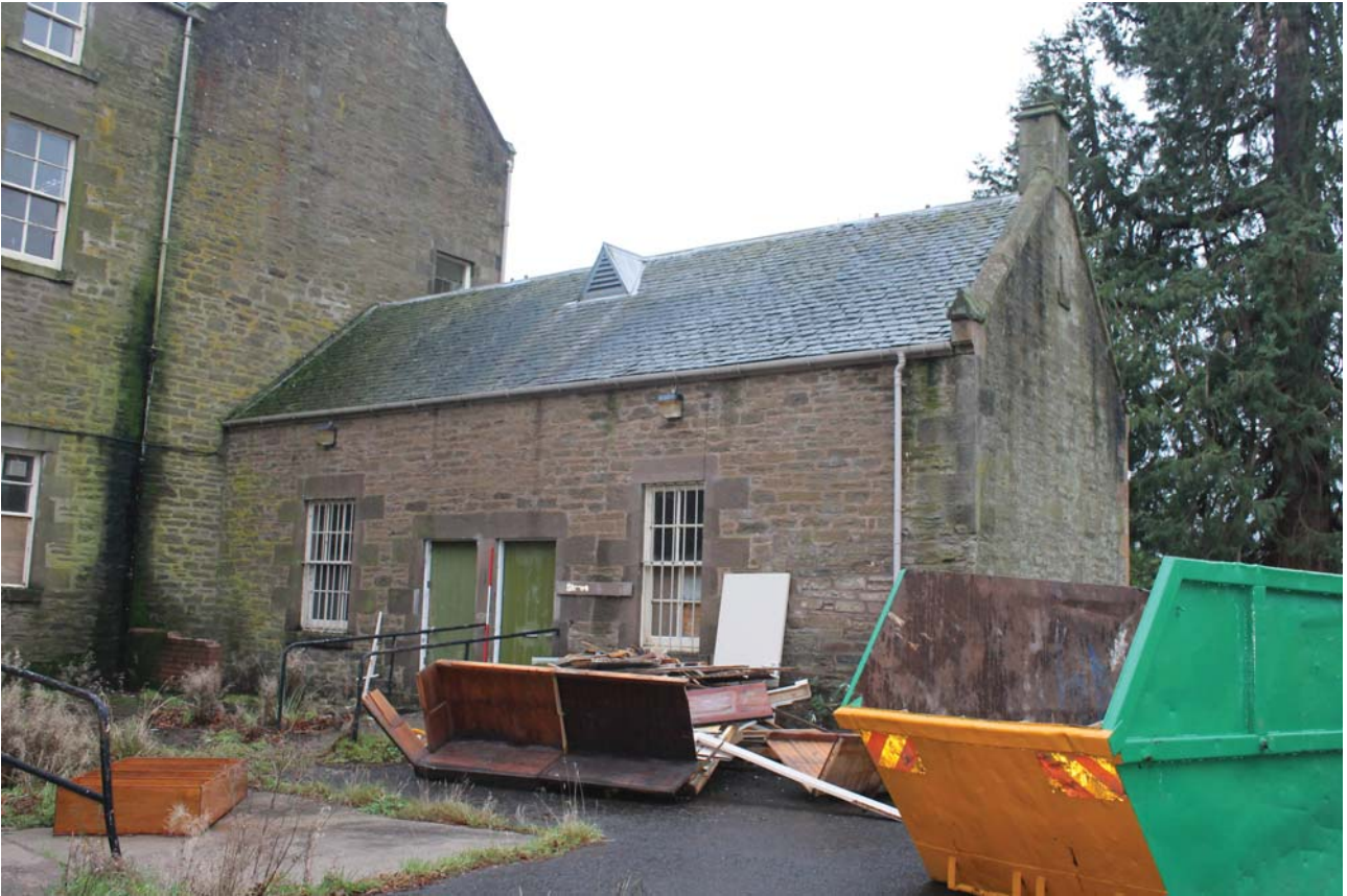
Plate 121: Building B1, general view from the north-east
