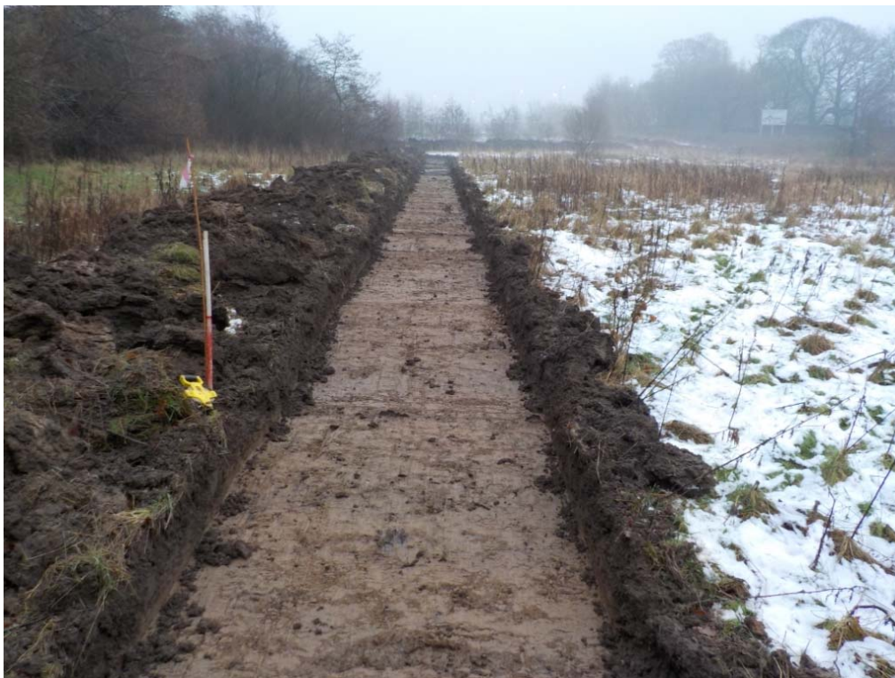
Plate 1 - Post excavation view of Trench 17
