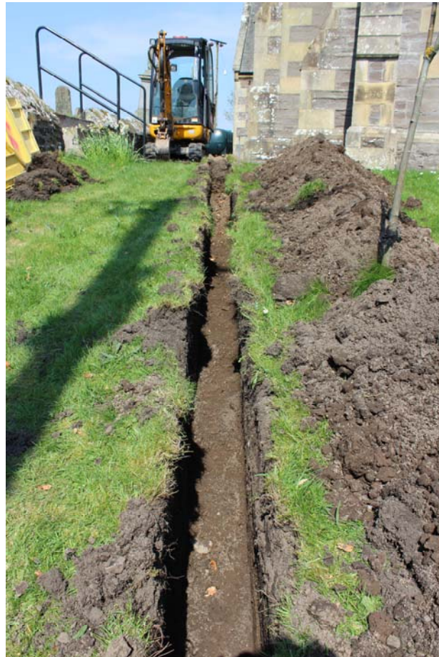
Plate 2: Cable track through grassy area at southern boundary
