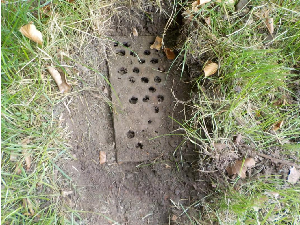
Plate 2 Modern metal grate
