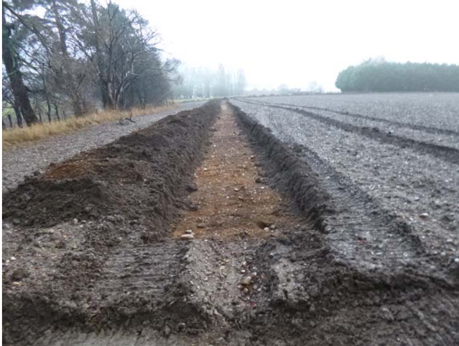
Plate 1: General view of Trench 8 showing some of existing woodland areas
