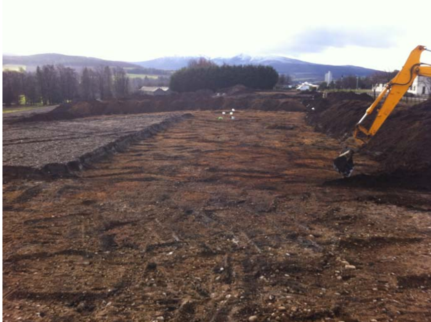
Plate 1: General view of topsoil stripping
