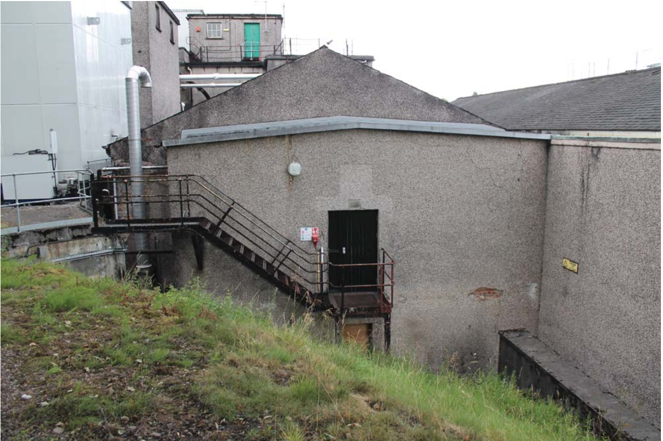
Plate 25: Mash House 1, general view from the south-west
