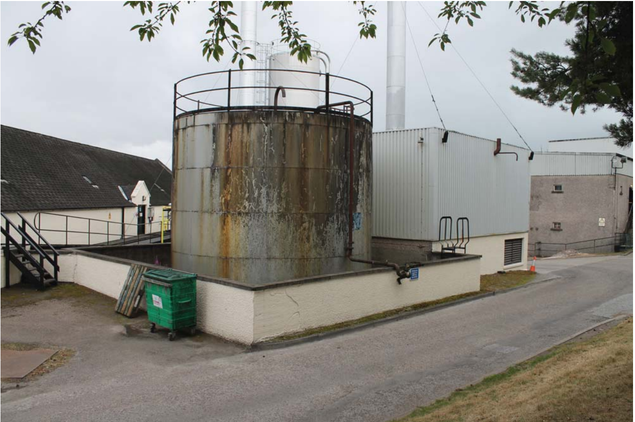
Plate 31: Boiler House 2, general view from the east
