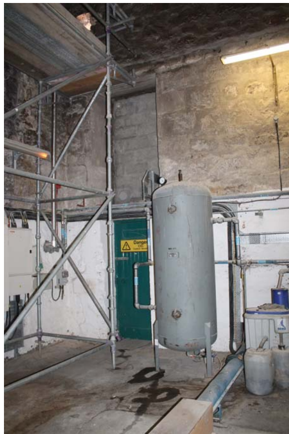
Plate 22: Malt Storage building, general view of the stone wall construction to the north corner of the building, from the north
