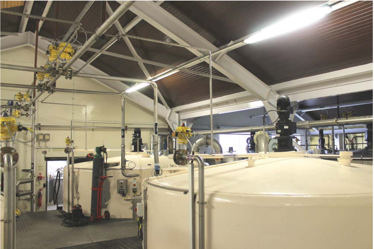
Plate 29: Mash House 1, general view of the upper level from the west
