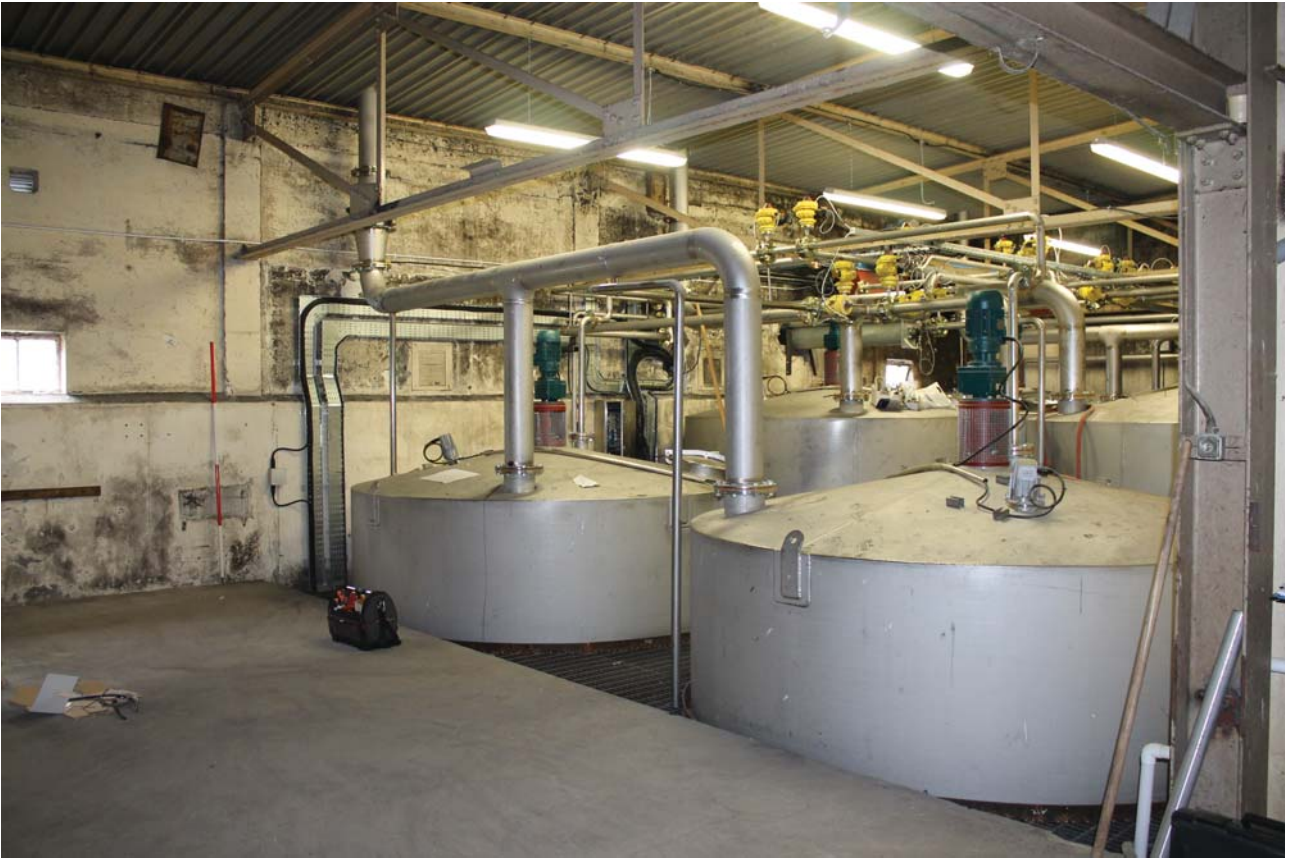
Plate 17: Hi Mac Building, general view of the attic level to the north-east side from the north
