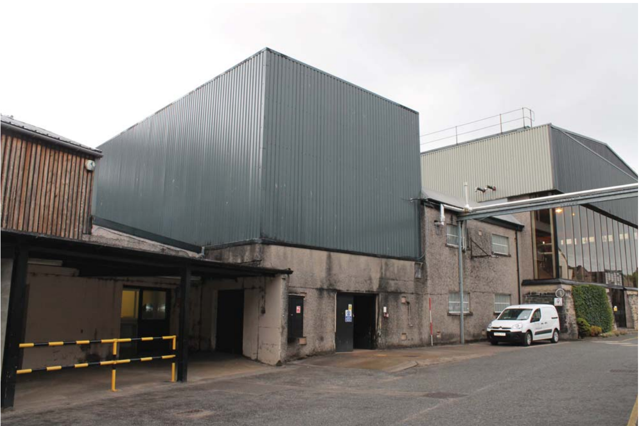
Plate 2: Still House 1, general view from the west
