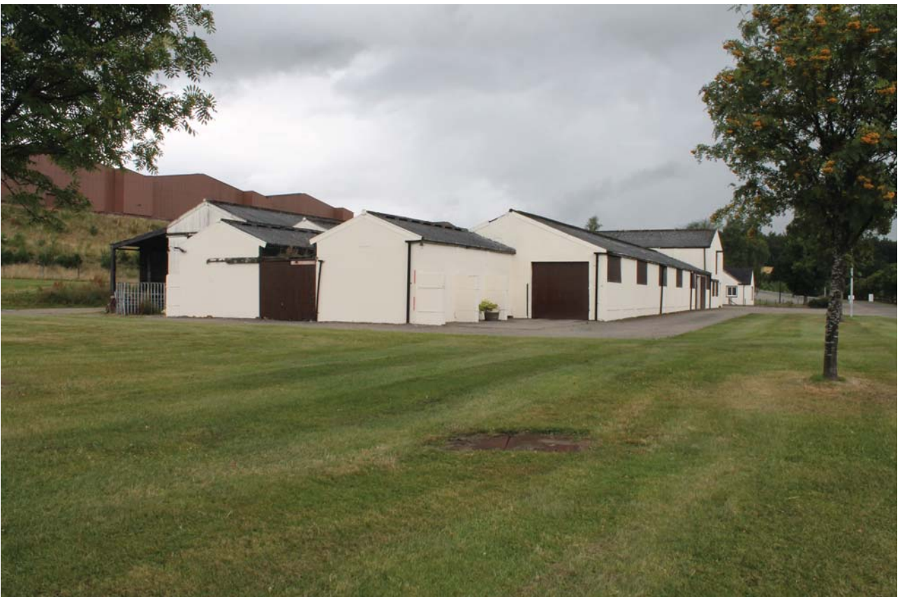
Plate 32: Farm Buildings, general view from the south
