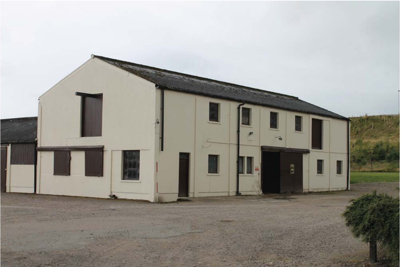
Plate 35: Farm Buildings, general view from the east
