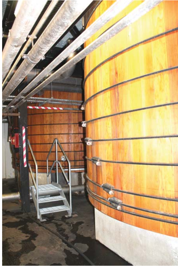
Plate 9: Still House 2, general view of the interior ground floor
