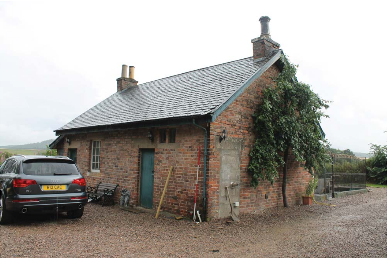
Plate 41: Kennels, general view from the west
