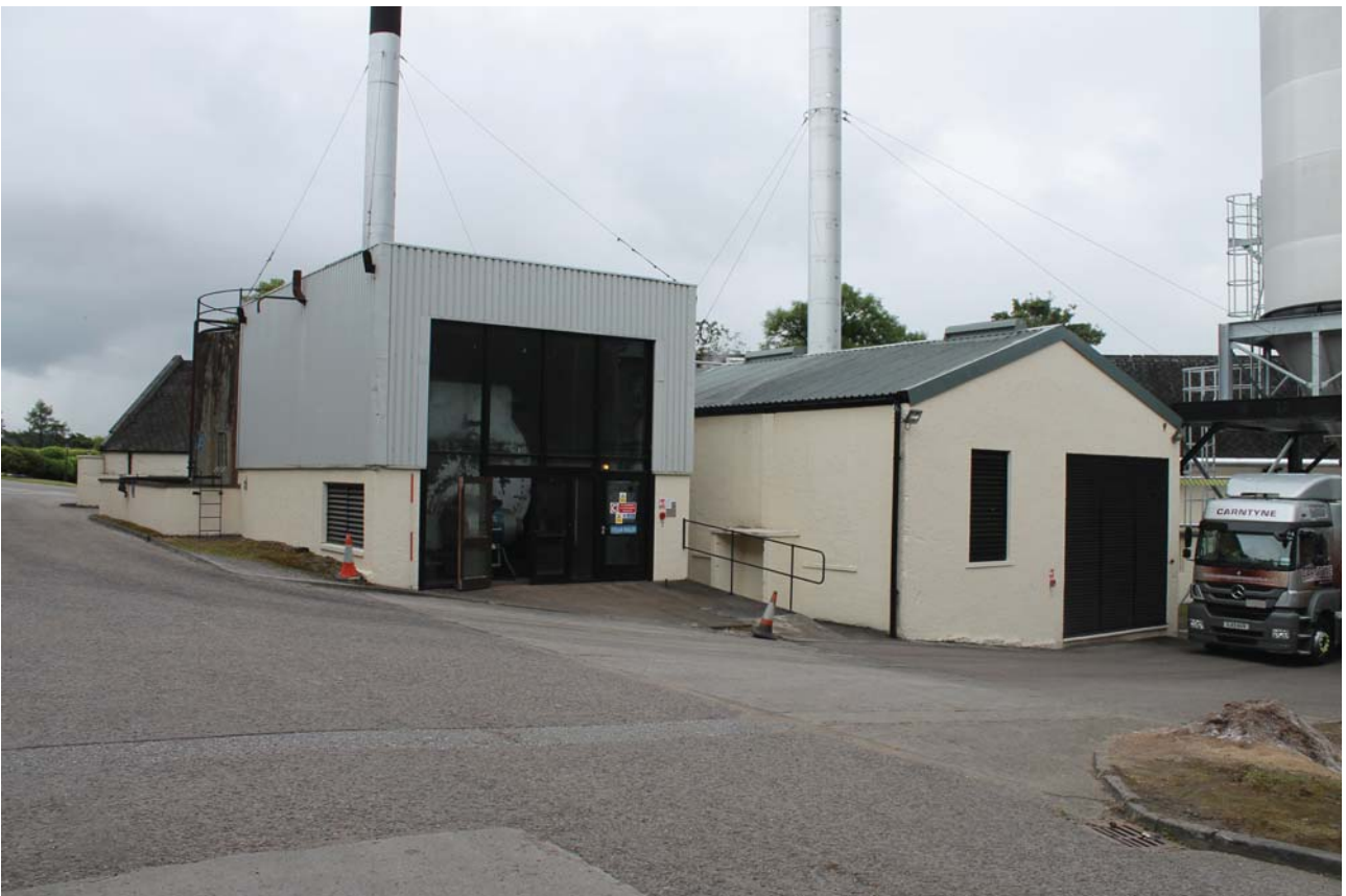
Plate 30: Boiler House 1 & 2, general view from the west
