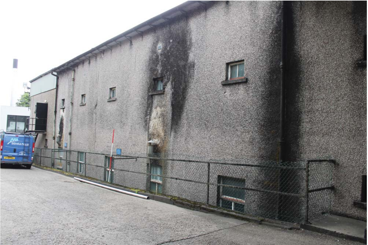
Plate 13: Hi Mac Building, general view of the north-west elevation from the west
