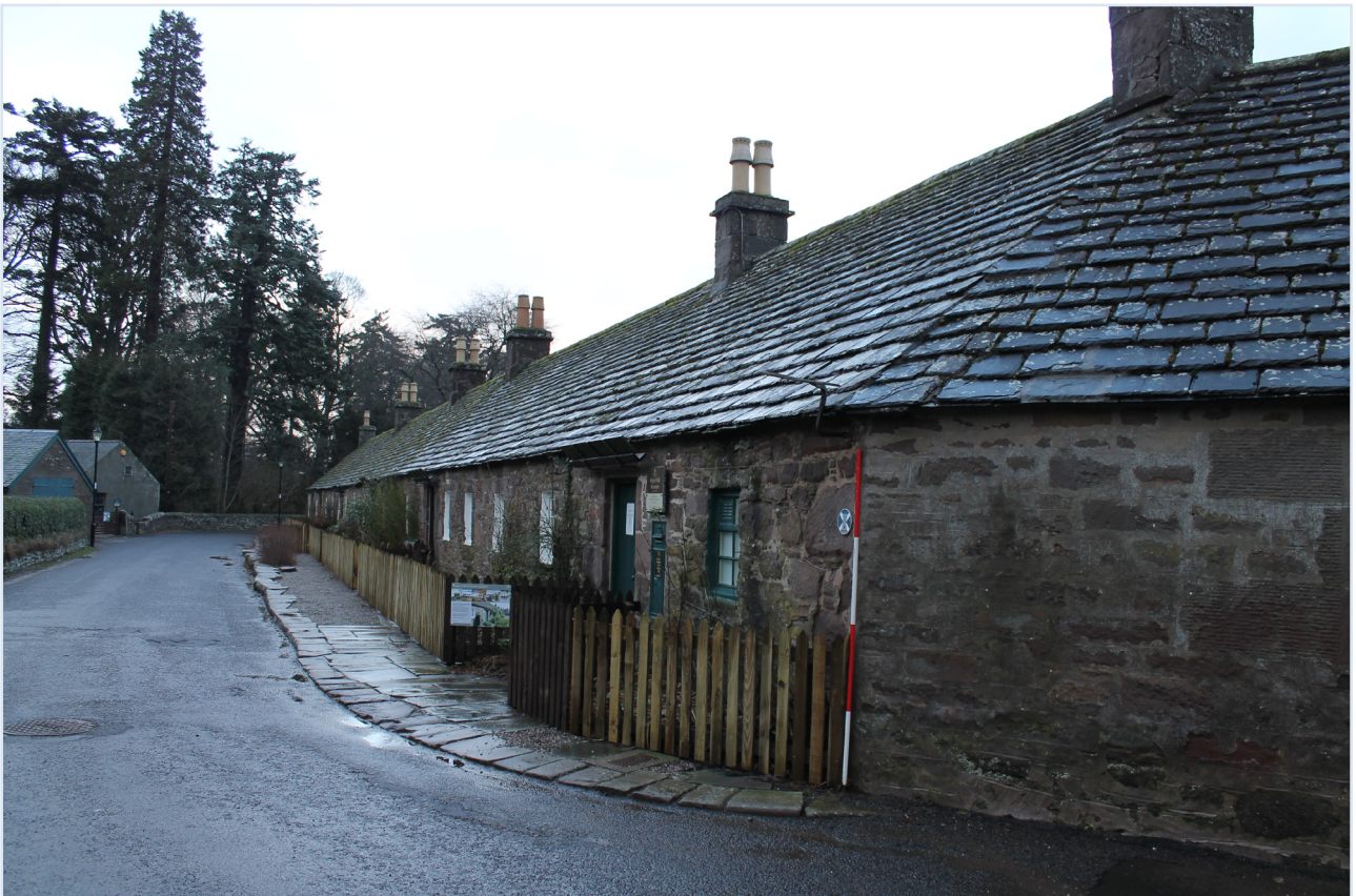
Plate 2: West elevation, general view from the south
