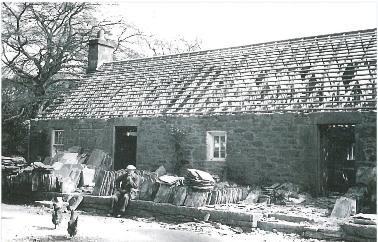
Plate 4: The re-roofing of Kirkwynd Cottages (RCAHMS References G91370 PO)
