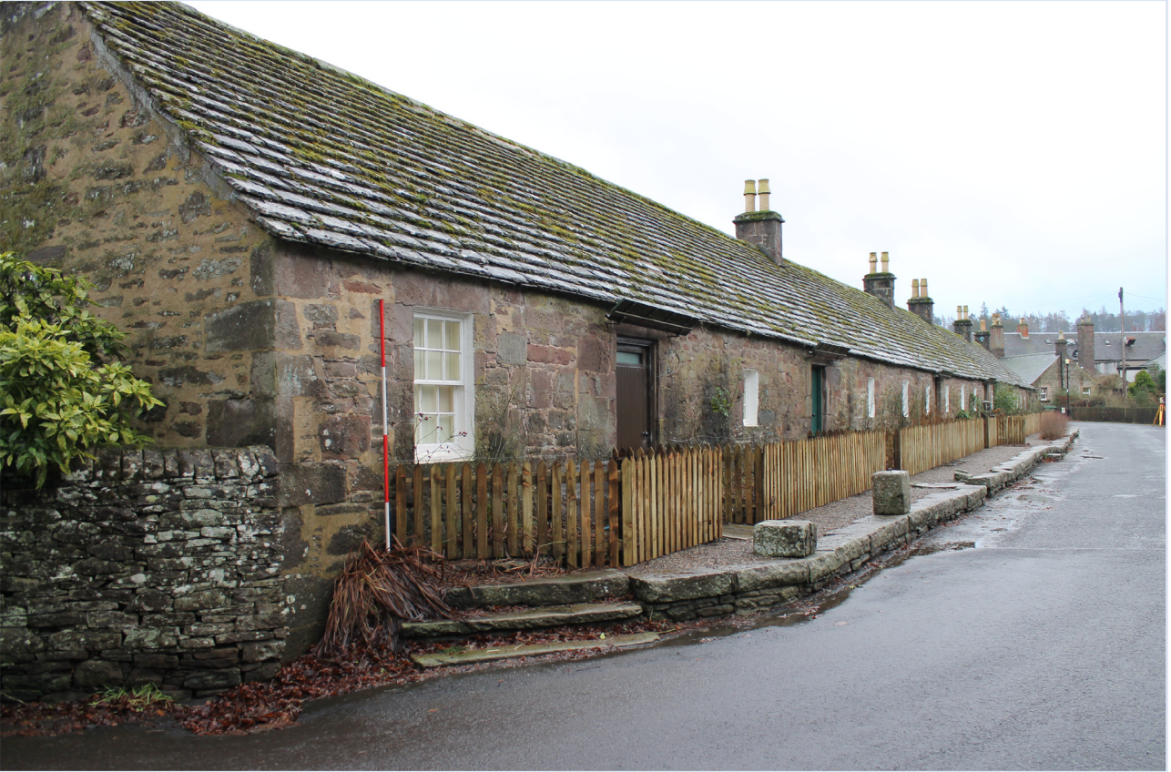
Plate 1: West elevation, general view from the north
