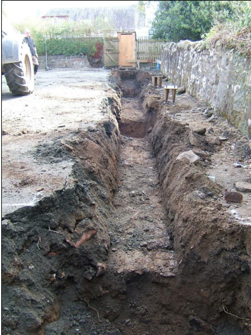
South trench viewed from the west
