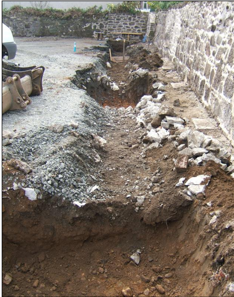
West trench viewed from the north
