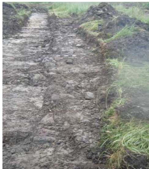
Illus 7 View of wall foundation [003] in Trench 7
