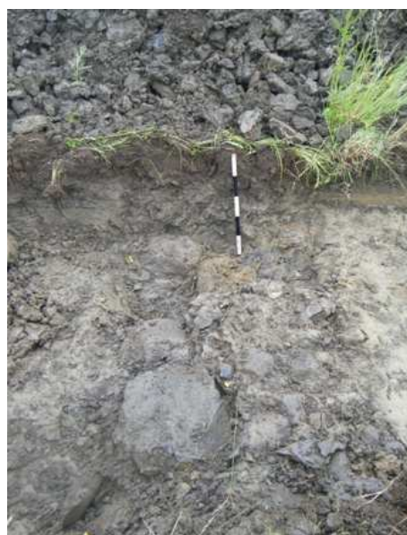
Illus 8 Detail of S facing section of wall foundation cut [003] in Trench 5
