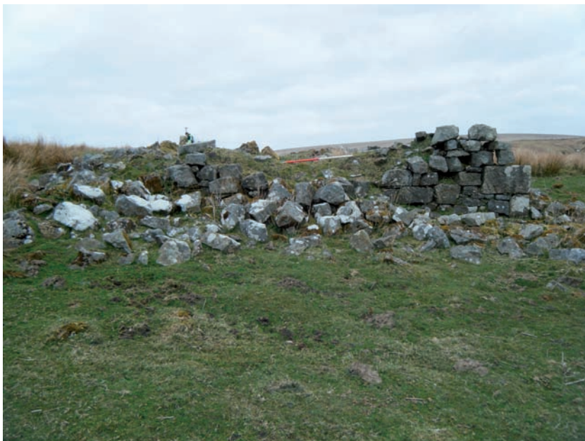
Illus 7 Byre end-wall looking northwest
