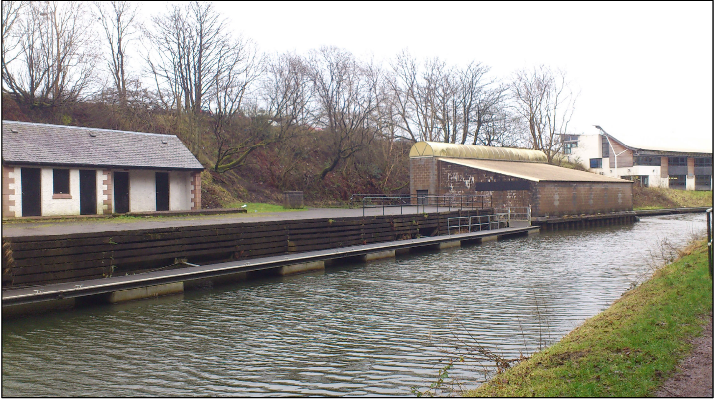
Plate 1: 1980s boatshed and a derelict facilities block, looking south.
