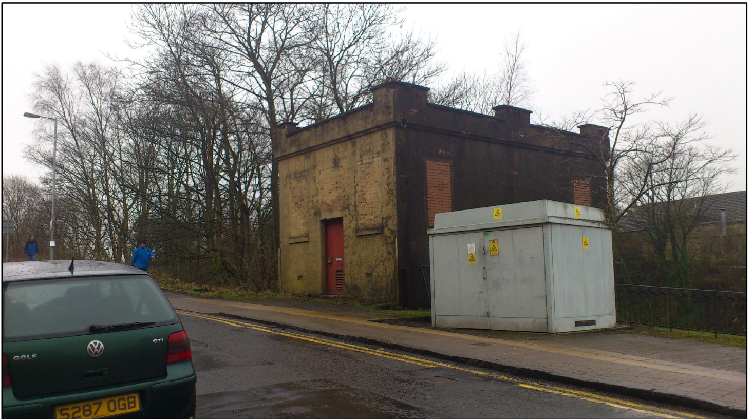
Plate 2: Utility building and electric sub-station enclosure, looking south-west.
