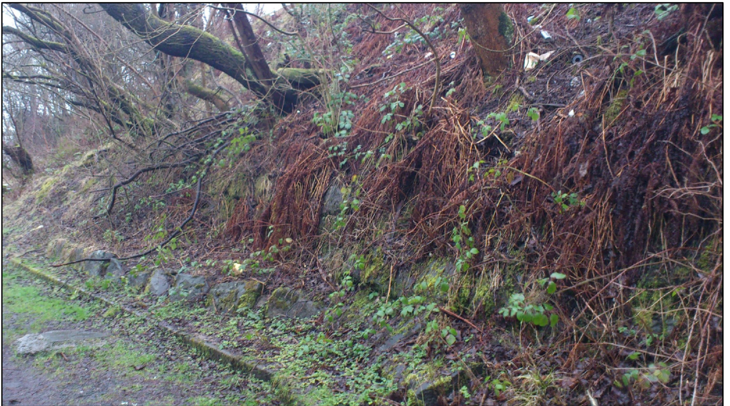
Plate 6: retaining wall in lower level of embankment, looking north-east.
