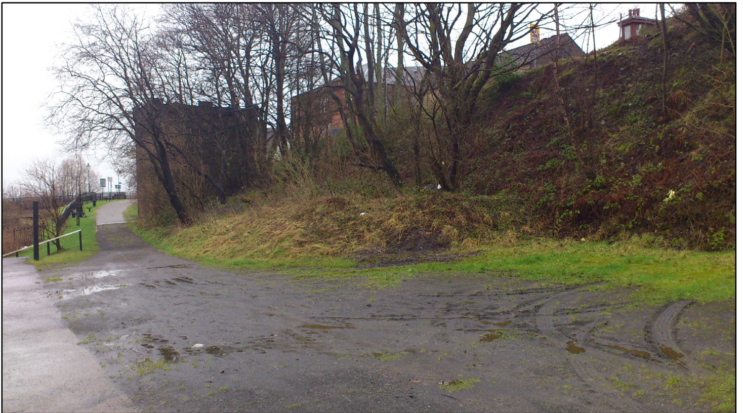
Plate 4: Terrace-like areas within northern part of embankment, looking north-east.
