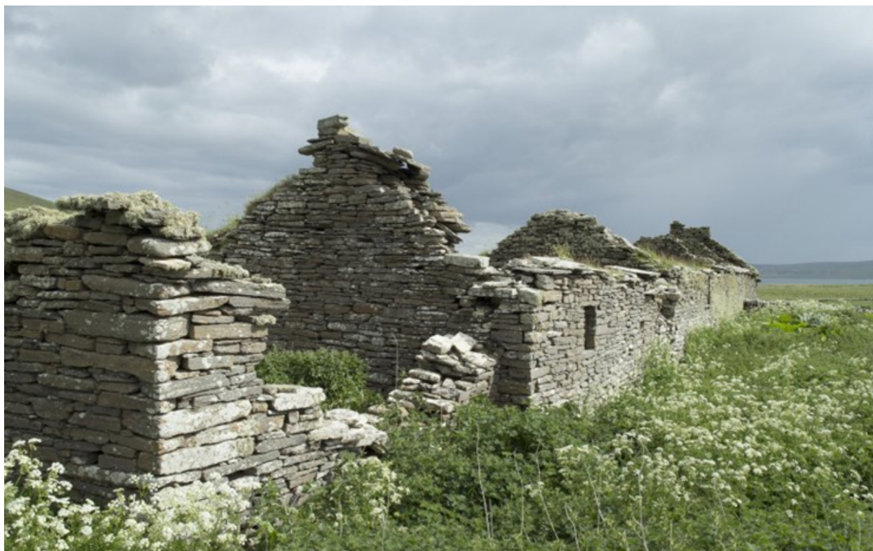
Illus 5. Farmhouse from the north-west showing the main phases of construction. DP256459.
