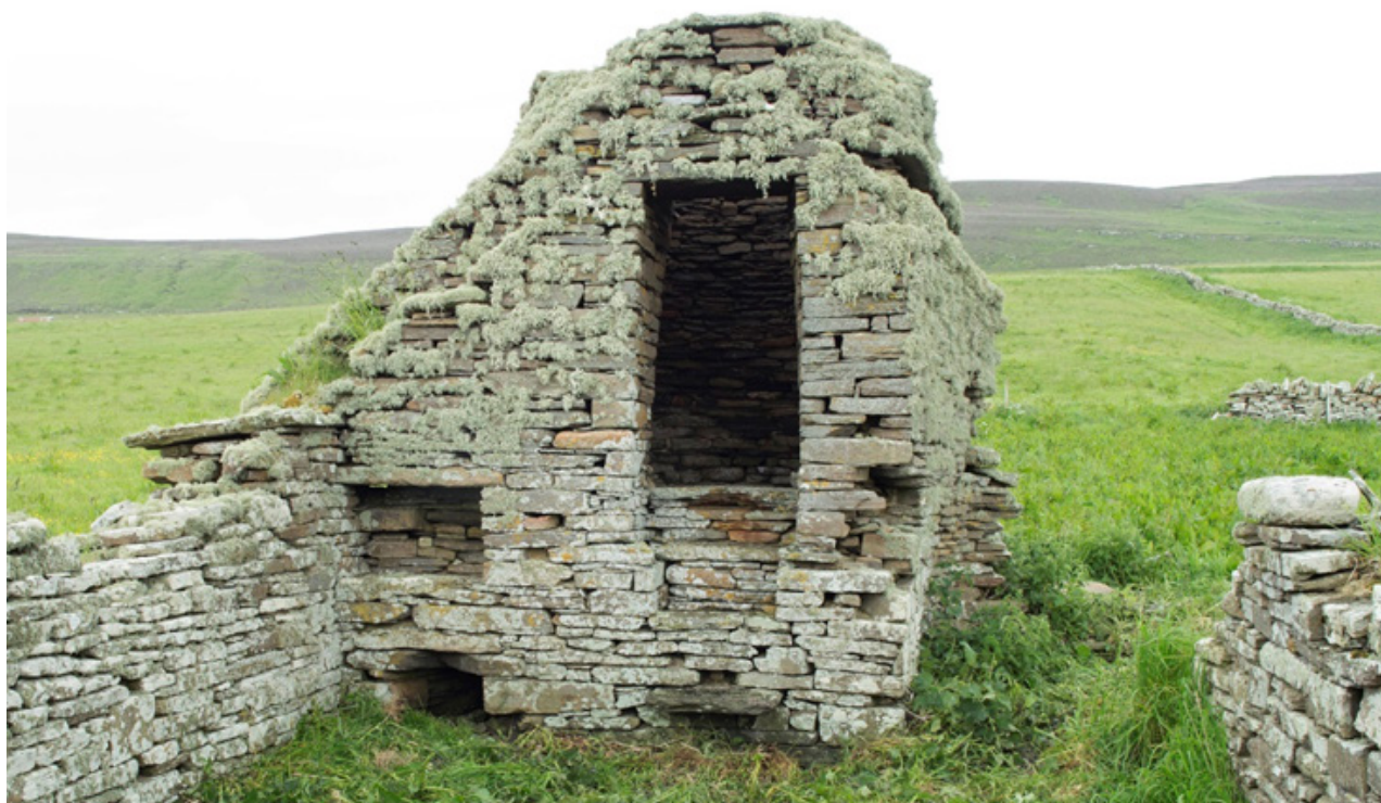
Illus 9. View from west of the east end of the kiln barn, showing the flue (bottom left) with an ambry (possible peat-store) above and the entrance into the interior of the kiln. The grain-store stood immediately to the right of the kiln, its walls now reduced to footings. DP256441.
