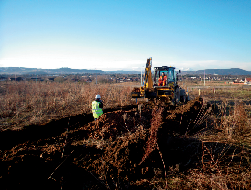
Illus 3 Excavating trench 2
