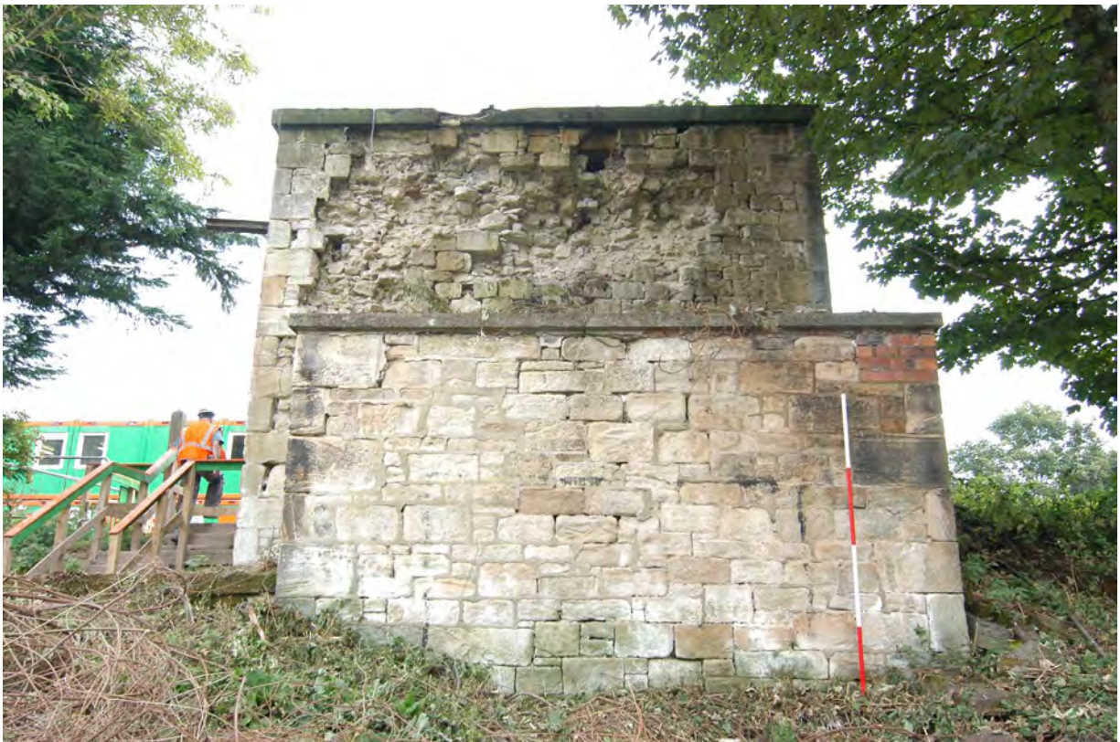
Plate 8 West-facing elevation of the water tower
