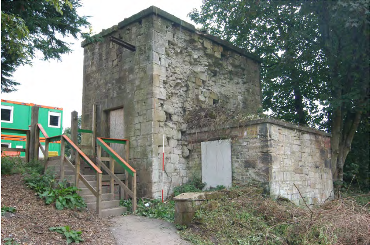
Plate 5 Oblique north-facing elevation of the water tower and outshot building
