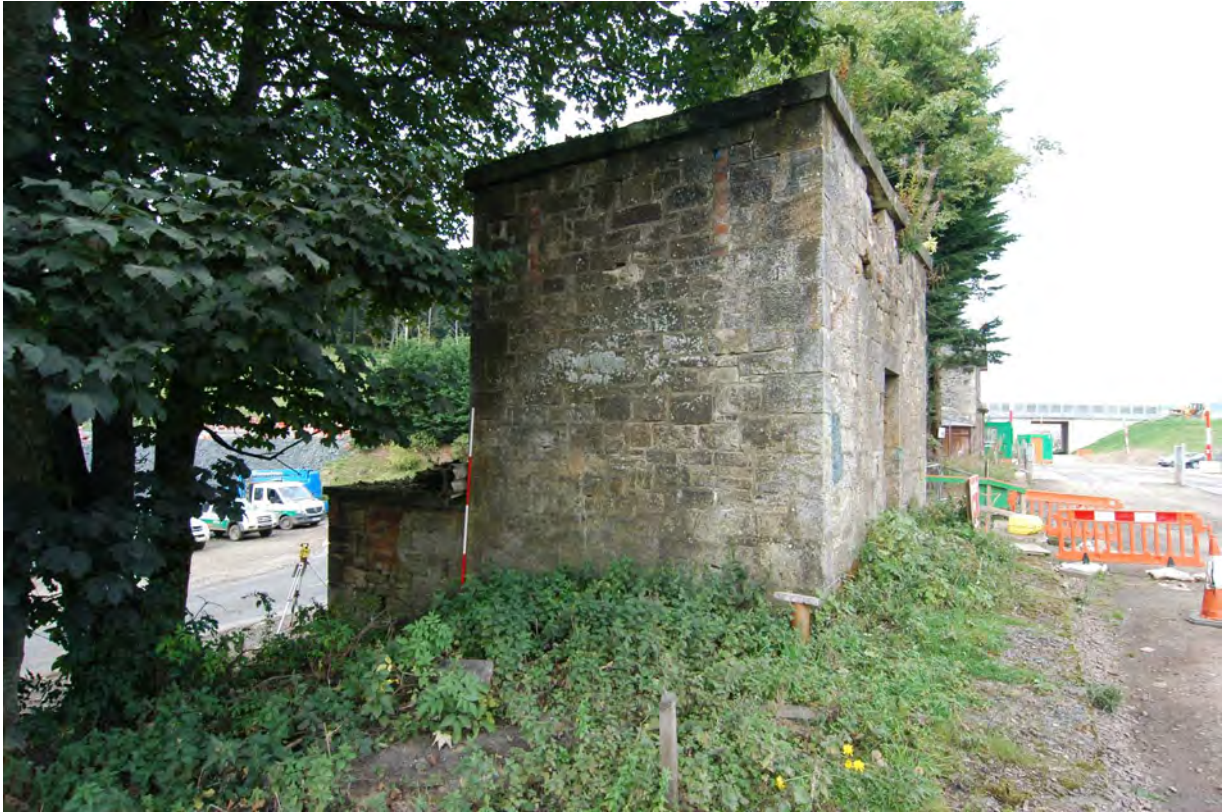
Plate 7 South-facing elevation of the water tower
