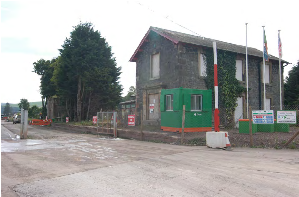
Plate 16 Northern terminus of the up platform and the former Station House
