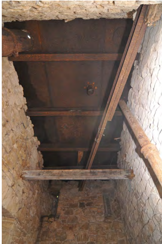
Plate 13 Interior ceiling showing iron plates and pipe work
