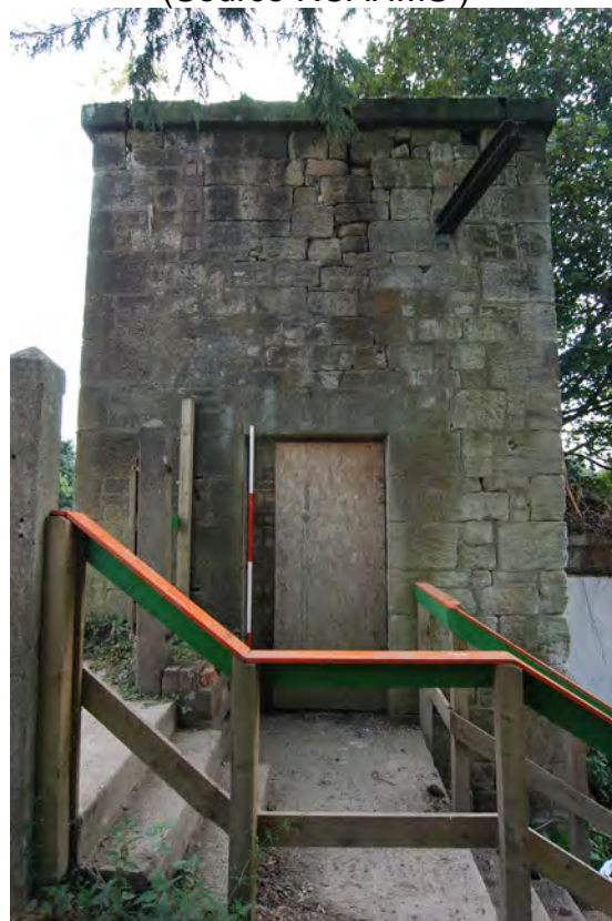
Plate 4 North-facing elevation of the water tower
