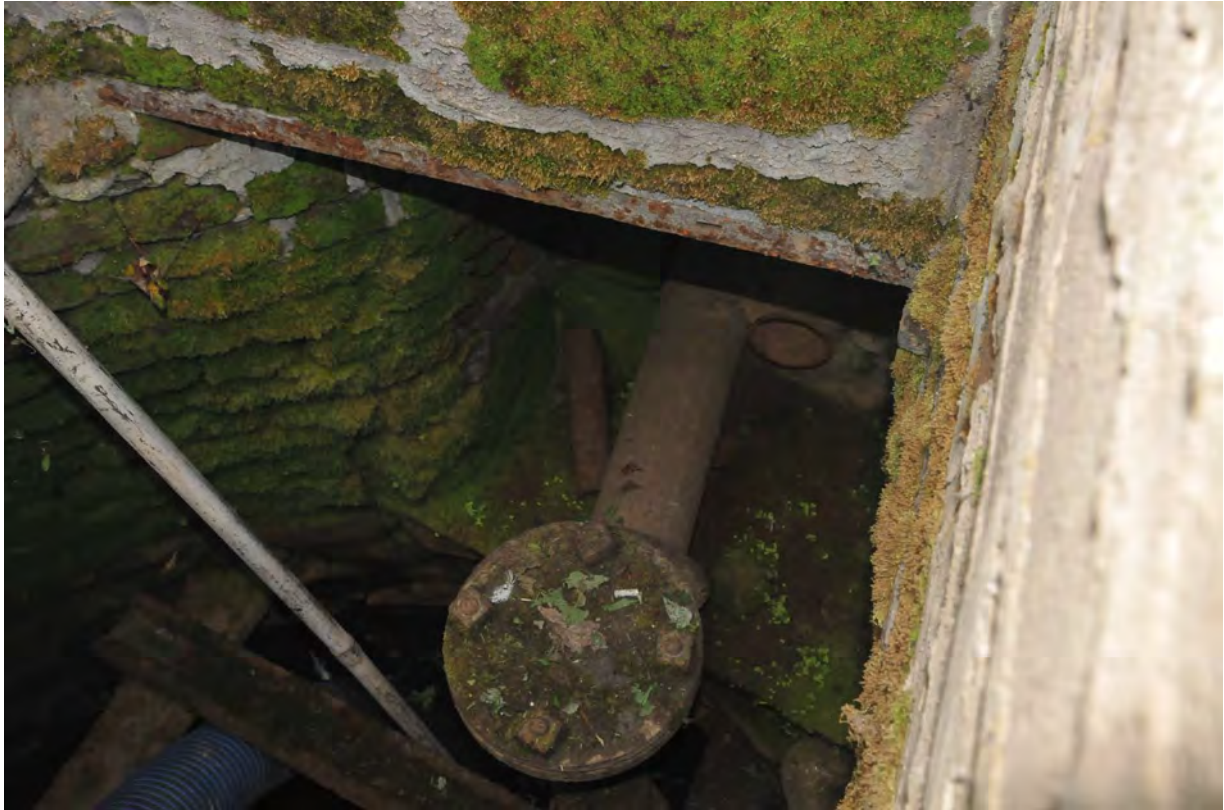
Plate 15 Well interior showing riser pipe and steel work below
