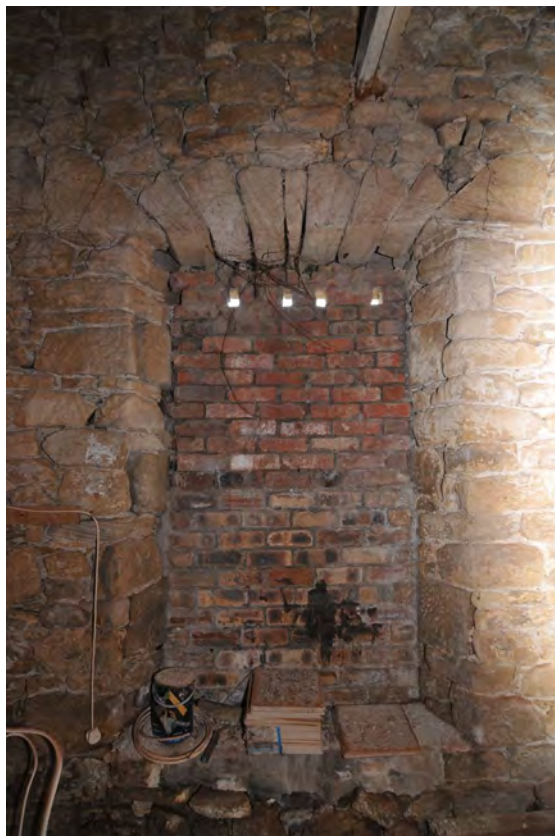
Plate 12 Interior west-facing elevation blocked opening
