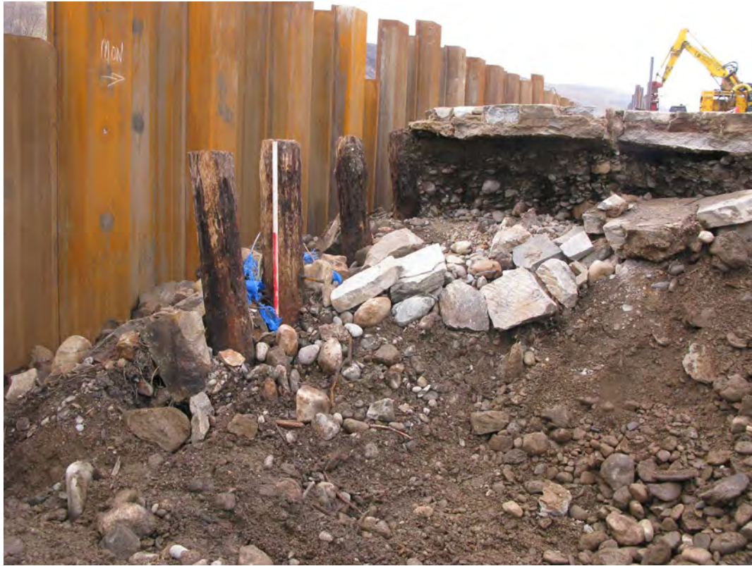
Fig. 7 Wooden piles along south-east side of weir
