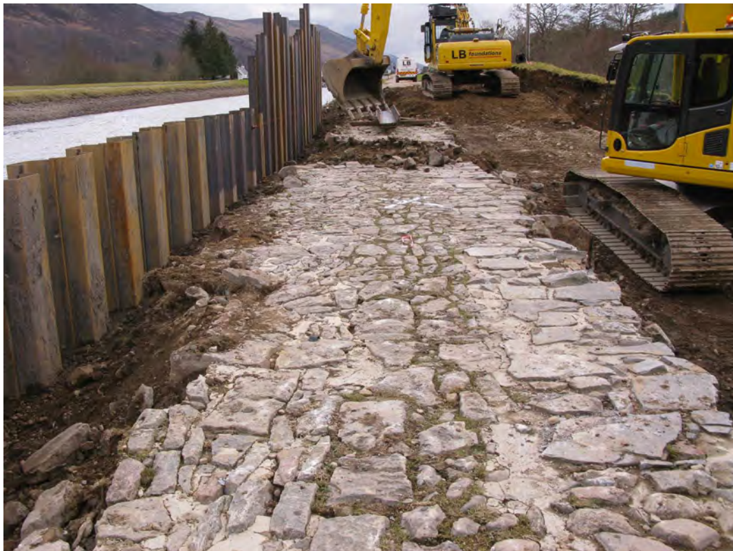
Fig. 8 Stone surface of weir
