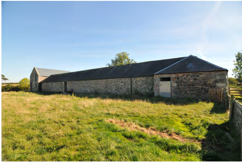
Fig. 17 North Range, north-facing elevation
