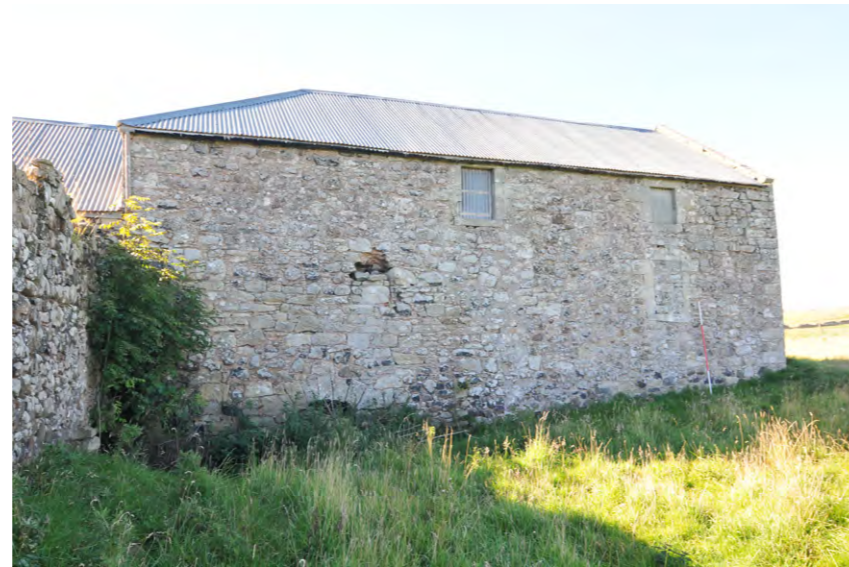
Fig. 9 East Range, east-facing elevation, north end
