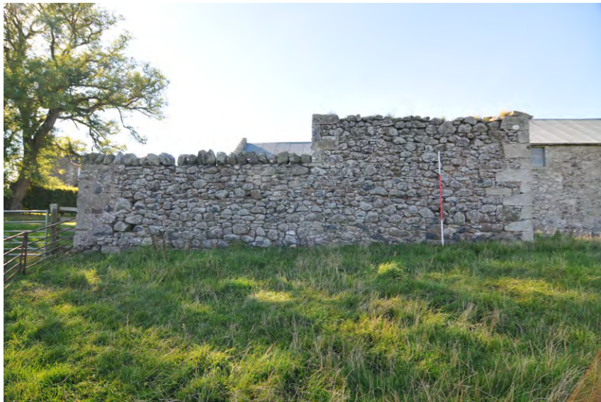
Fig. 8 East Range, east-facing elevation, south end
