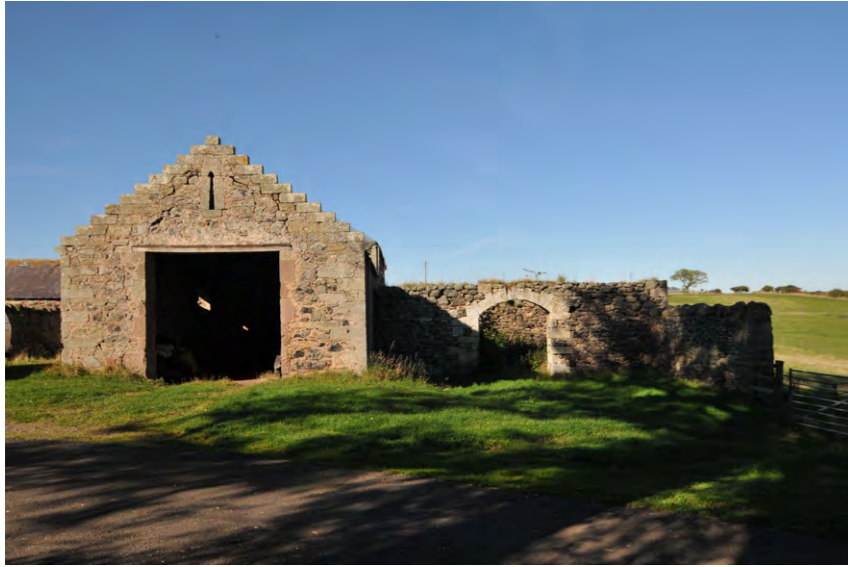
Fig. 11 East Range, south-facing crow stepped gable
