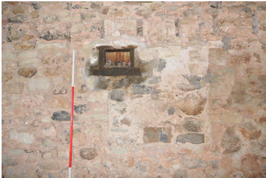
Fig. 14 East range, west-facing elevation bearing box and first floor joist sockets
