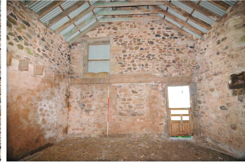
Fig. 13 East Range, interior south-facing elevation
