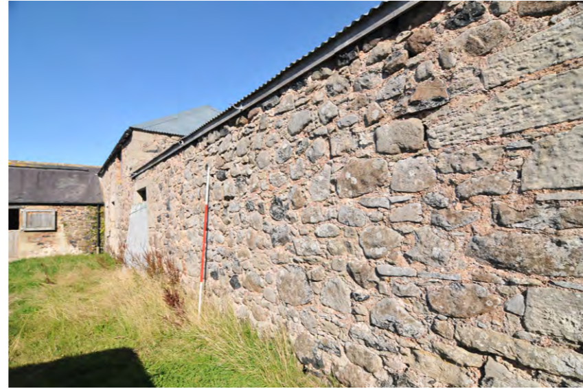
Fig. 12 East Range, west-facing elevation
