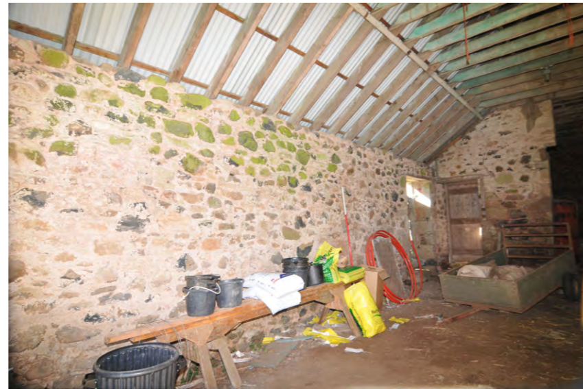
Fig. 15 East Range, east-facing elevation with surviving section of a partition wall
