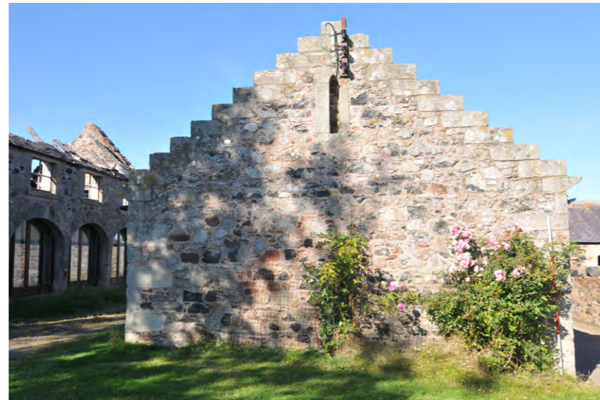
Fig. 21 West Range, south-facing gable
