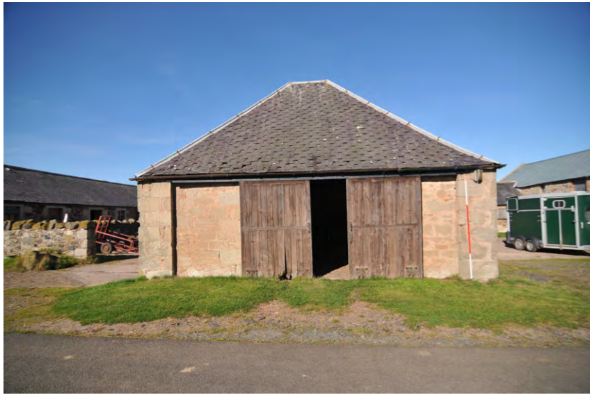
Fig. 5 Exterior view of the Turnip Shed, Unit 1
