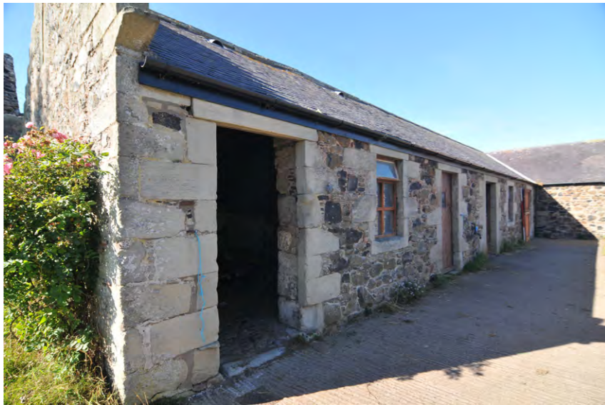
Fig. 20 West Range, east-facing elevation
