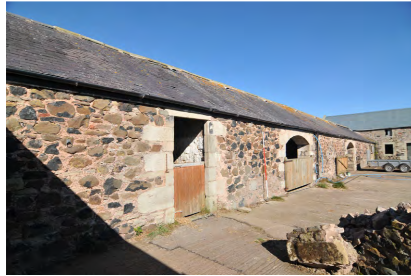
Fig. 18 North Range, south-facing elevation
