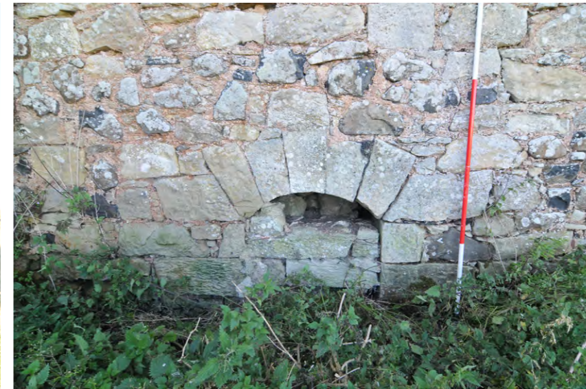
Fig. 10 East Range, east-facing elevation, segmented arched opening
