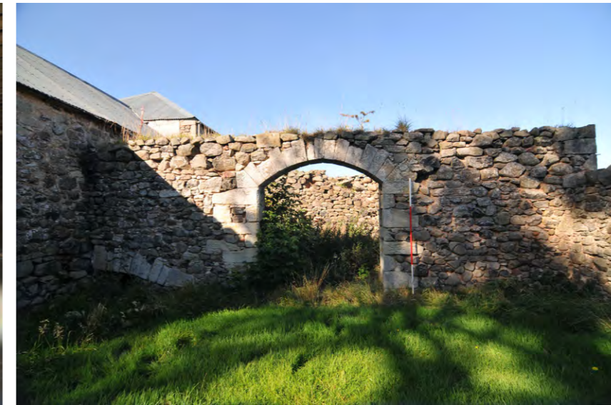
Fig. 16 East range outshot building, south-facing elevation
