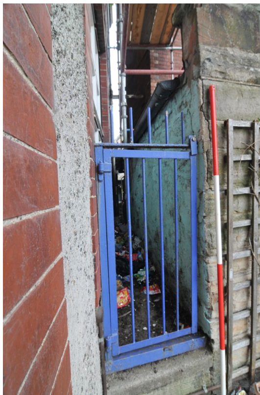
Fig. 9 - Part of the south-facing elevation of the boiler house
