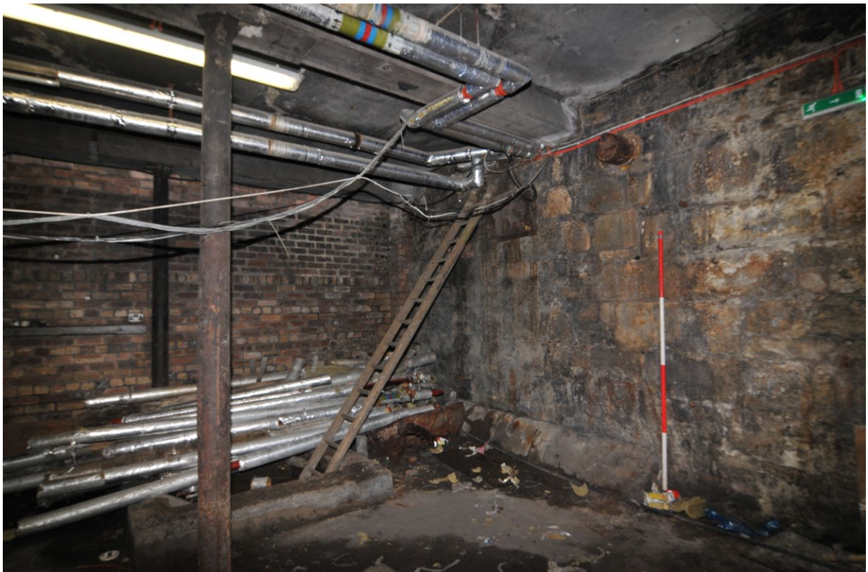
Fig. 12 - Interior north-facing elevation of the boiler room
