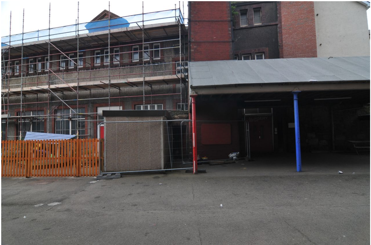
Fig. 5 - North-facing elevation of the boiler house partially hidden behind a modern shed
