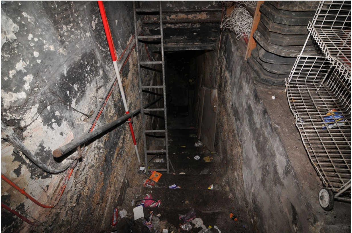
Fig. 11 - Boiler room, interior stone steps
