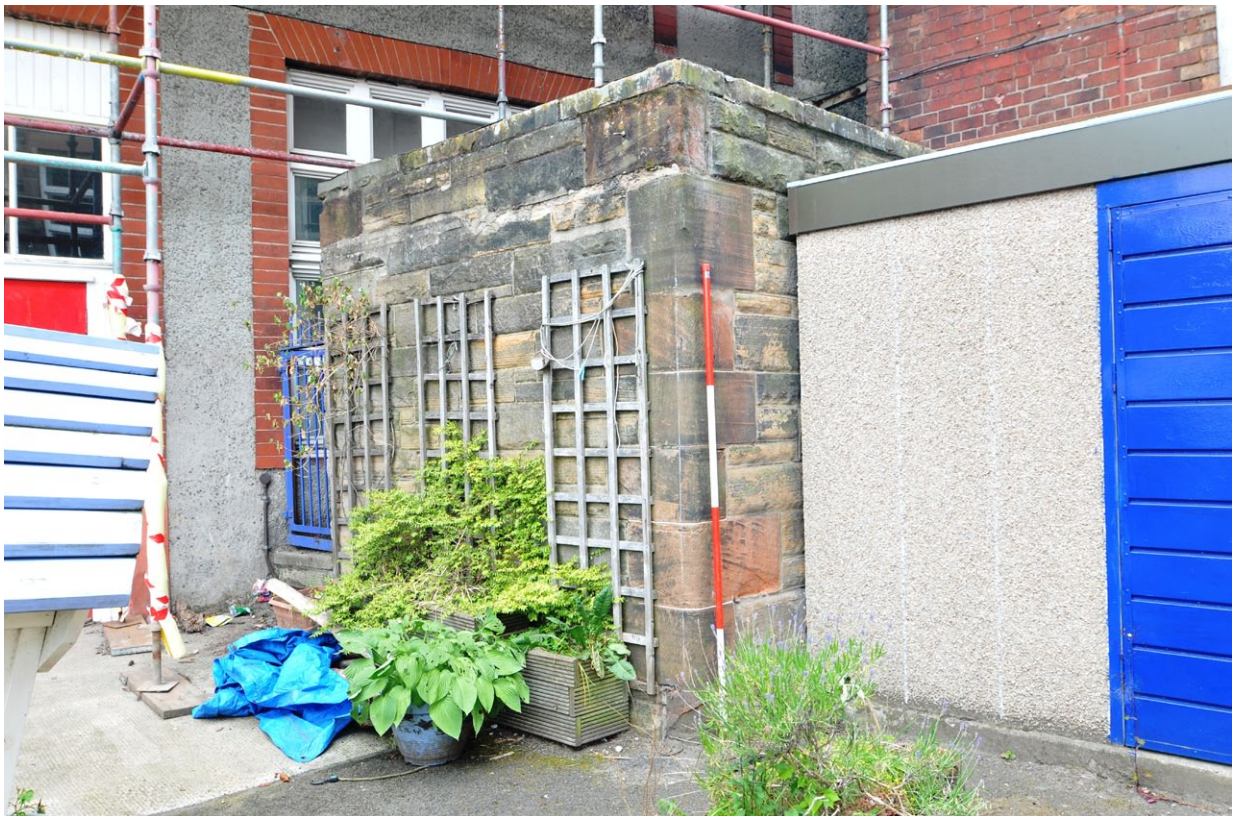
Fig. 8 - Detailed shot of the east-facing elevation of the boiler house
