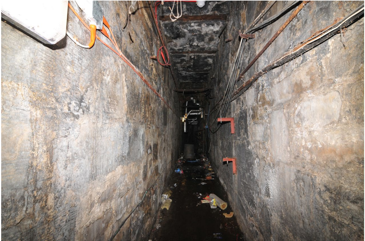
Fig. 15 - The passage interior leading north from the boiler room
