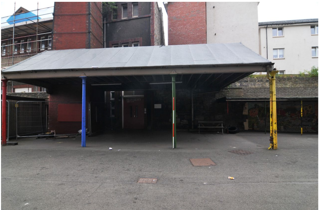
Fig. 6 - North-facing elevation with canopy and chimney
