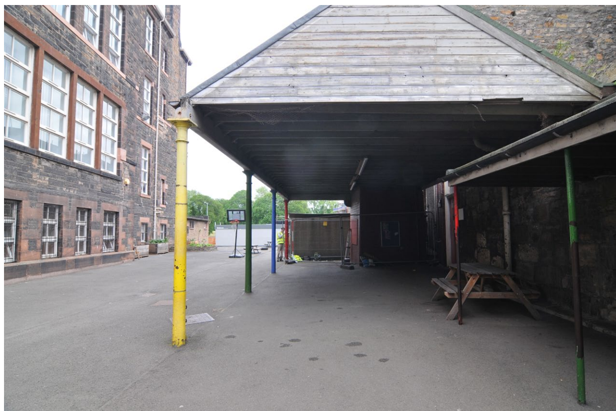
Fig. 10 - West-facing elevation of the canopy
