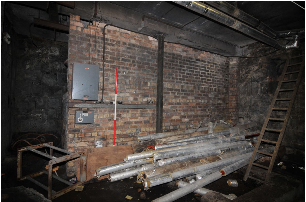
Fig. 14 - Interior west-facing elevation of the boiler room bunker
