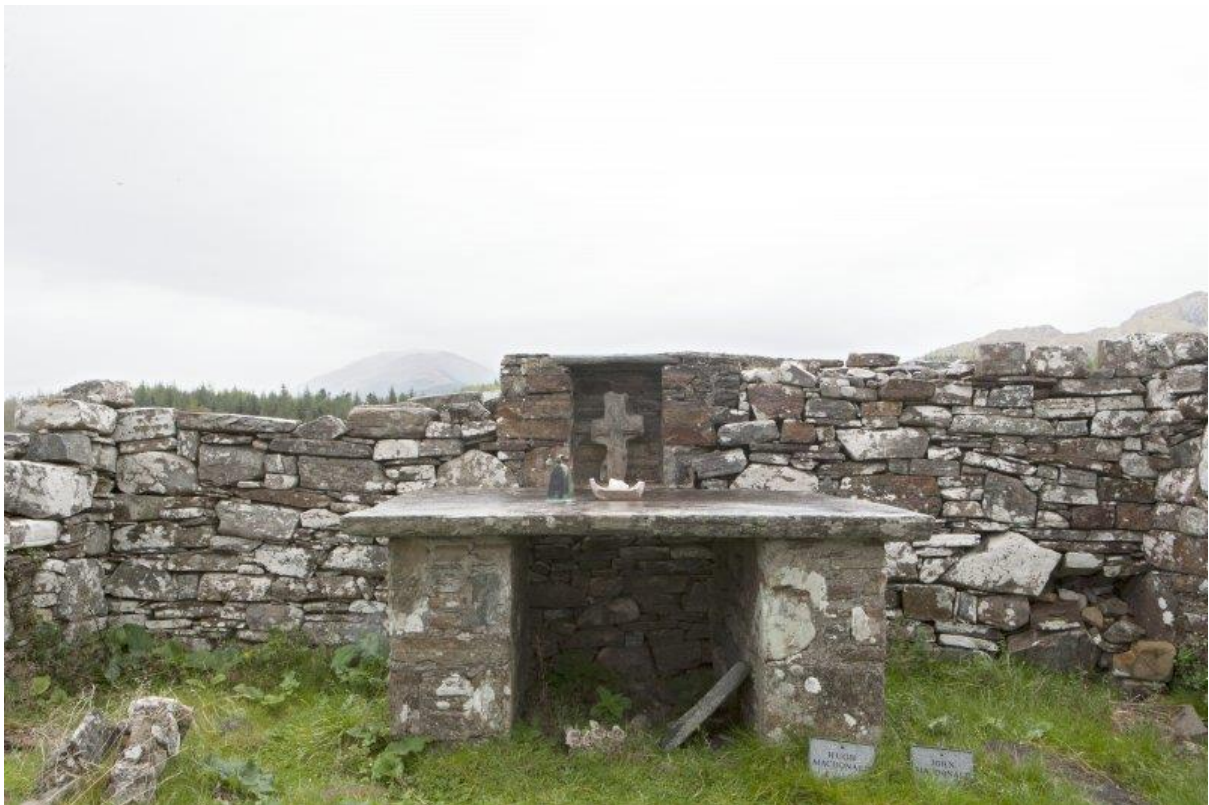
Figure 10 The 'altar' and niche at the E end of the church appear to be modern features, perhaps constructed as a backdrop for the bell, and the late-medieval cross-head set into the niche. Much of the gable behind has been reconstructed.
